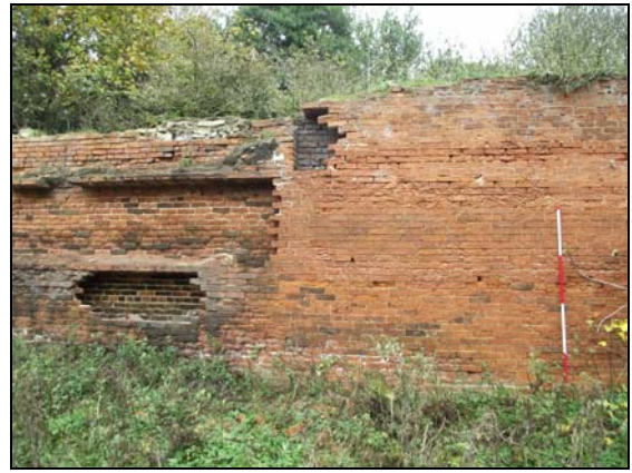
Plate 4, 95: general view of the NE wall, SW elevation, from the southwest
