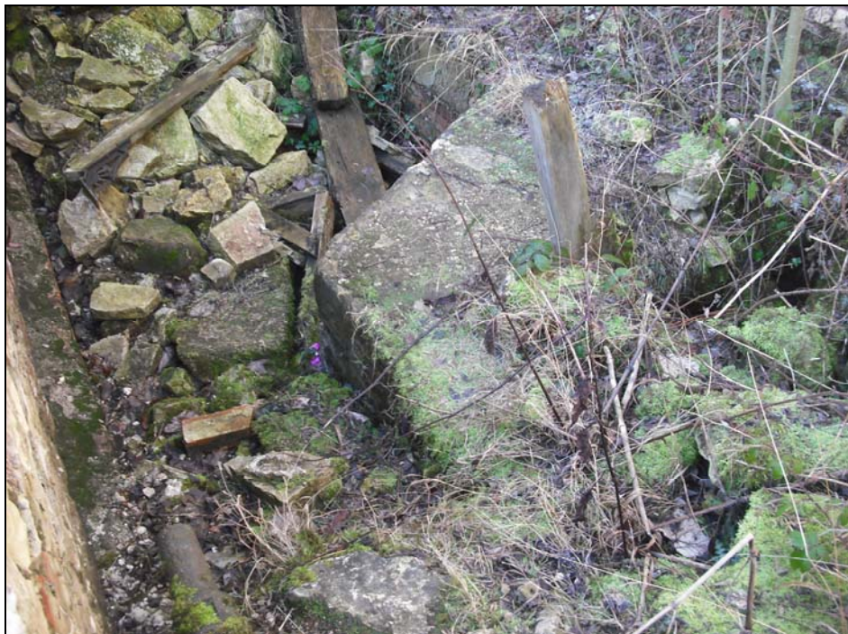
Plate 2: detail of the associated cast iron pipework and well
