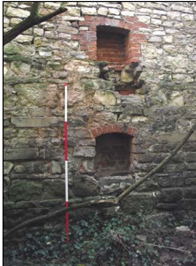
Plate 15 , 48: Detail of the arched alcoves [18], from the north
