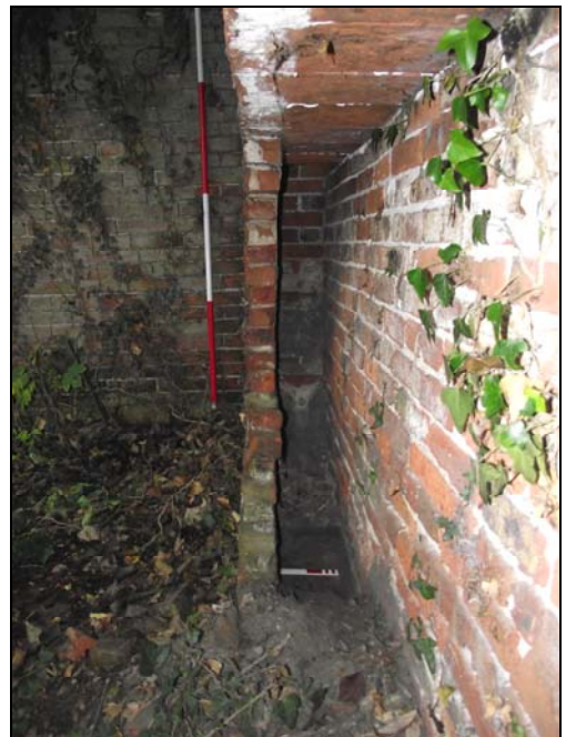
Plate 10, 70: detail of the exposed heating duct to the NW wall, SE elevation, from the northeast
