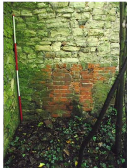
Plate 6, 14: detail of the twin furnace twin ducts [33], from the northwest
