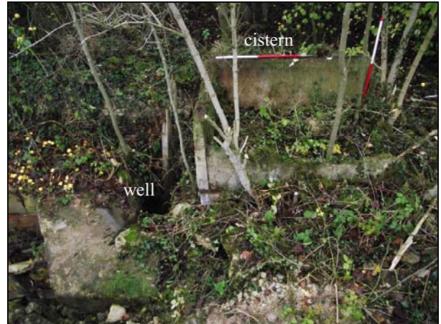
Plate 20, 120: View of the stone cistern [7] (with ivy removed), from the southeast
