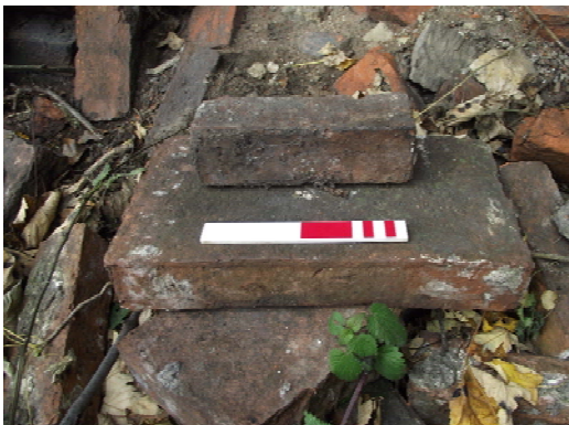
Plate 11, 128: Detail of the narrow facing brick with bridging brick beneath
