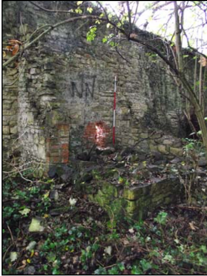
Plate 13 , 10: Oblique view of building 1, from the northeast
