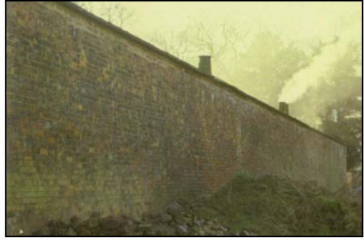
Plate 8: the heated fruit wall at Tatton Park without furnace sheds, which used bonfires at the base of the wall (Campbell 2011, 25)
