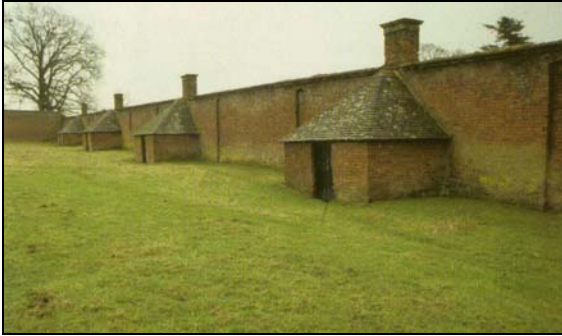
Plate 7: a row of furnace sheds behind the heated fruit wall at Weston Park Staffordshire (Campbell 2011, 25)
