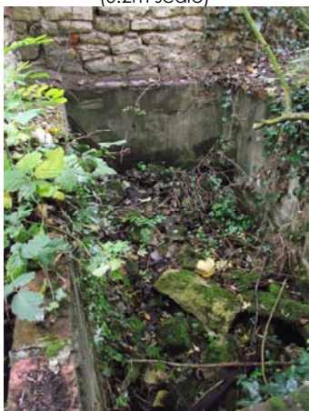
Plate 23, 47 : View into the cistern [17], building 3, from the northwest
