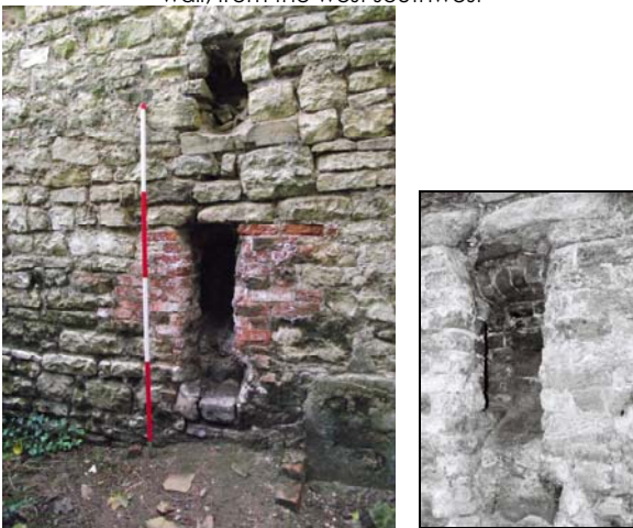
Plate 5, 133 detail of the furnace duct [19], from the northwest
