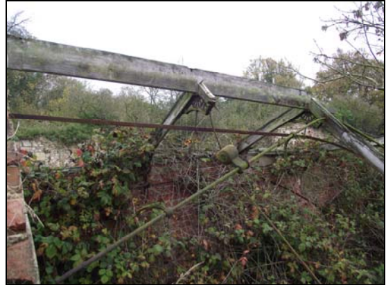
Plate 26 , 110: detail of the greenhouse roof, from the southwest
