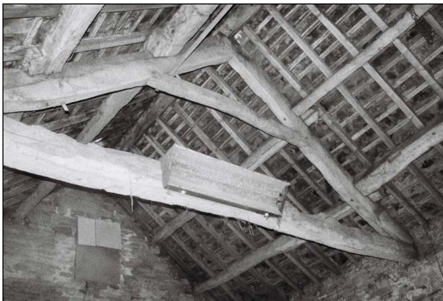
Plate 11, 25: view of the original oak roof truss (2), looking southeast
