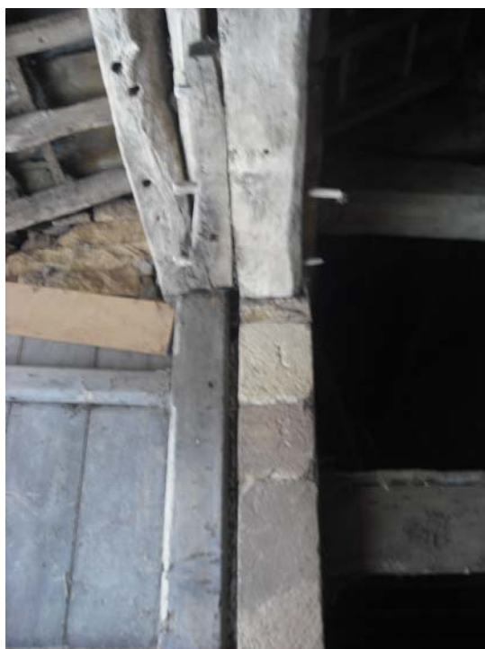
Plate 13, 24: View of the type 1 mason's marks and the inserted pegged timber for the hinge of the barn door [4], looking southeast
