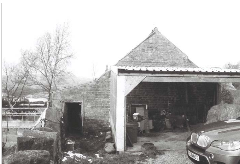
Plate 8, 3: The southeast gable obscured by later lean-to (Building 2), looking southwest
