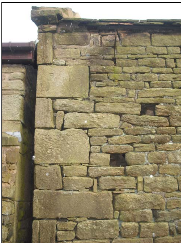
Plate 5, 38: detail of the rear southwest elevation (bay 3), looking northeast
