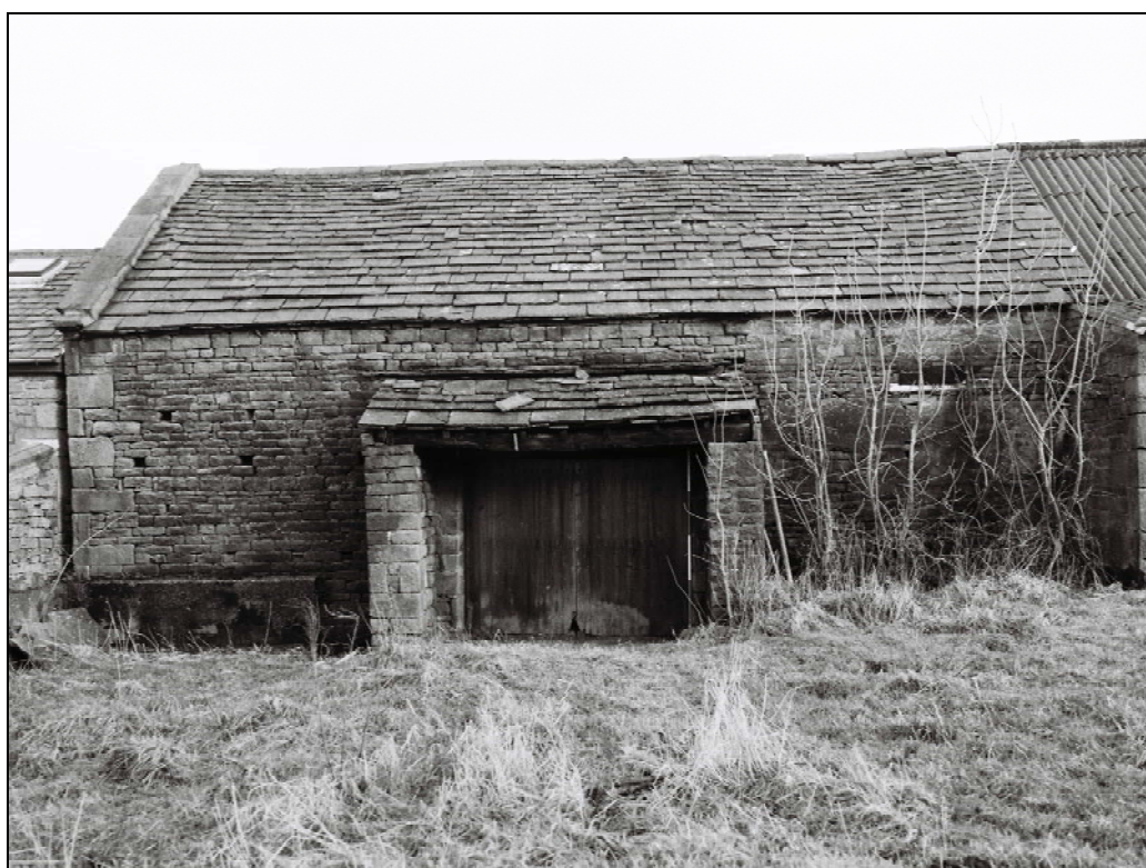
Plate 4, 40: view of the rear southwest elevation with the lower cheeked porch [8] and graduated stone flag roof, looking northeast
