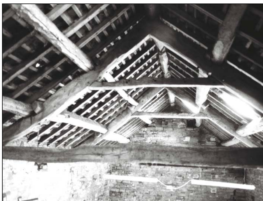
Plate 12, 50: view of the roof from the hayloft, looking northwest
