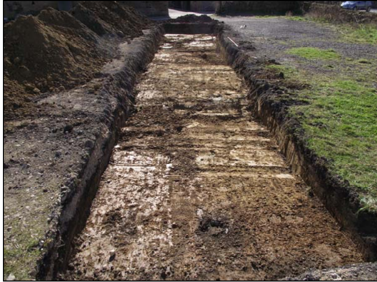
Plate 1 , 33: post-excavation view of trench 1 (with ridge to the right), looking southeast
