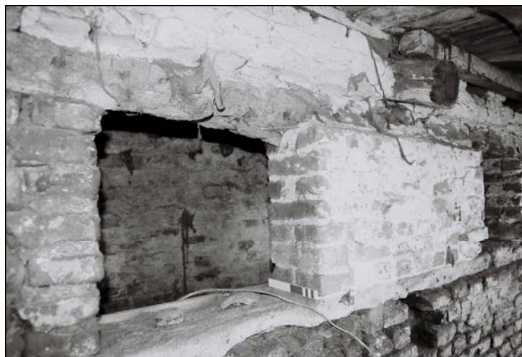
Plate 15, 56: oblique view of the feeding holes, looking southwest
