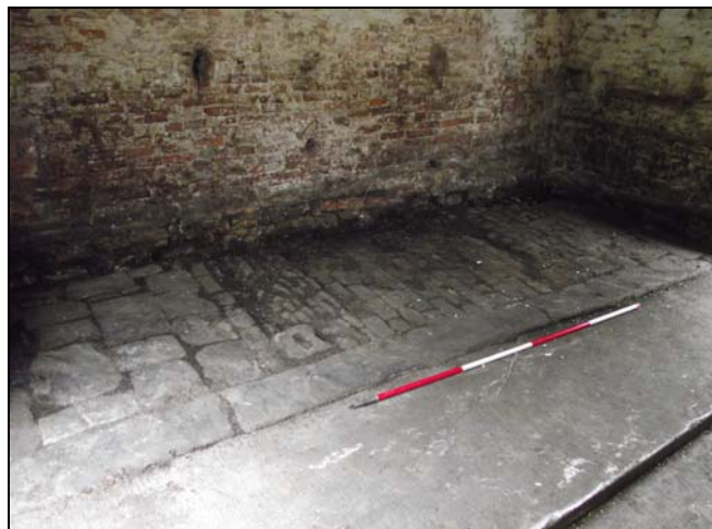
Plate 12, 29: view of the floor (stone setts in a 3 stall configuration), looking southeast
