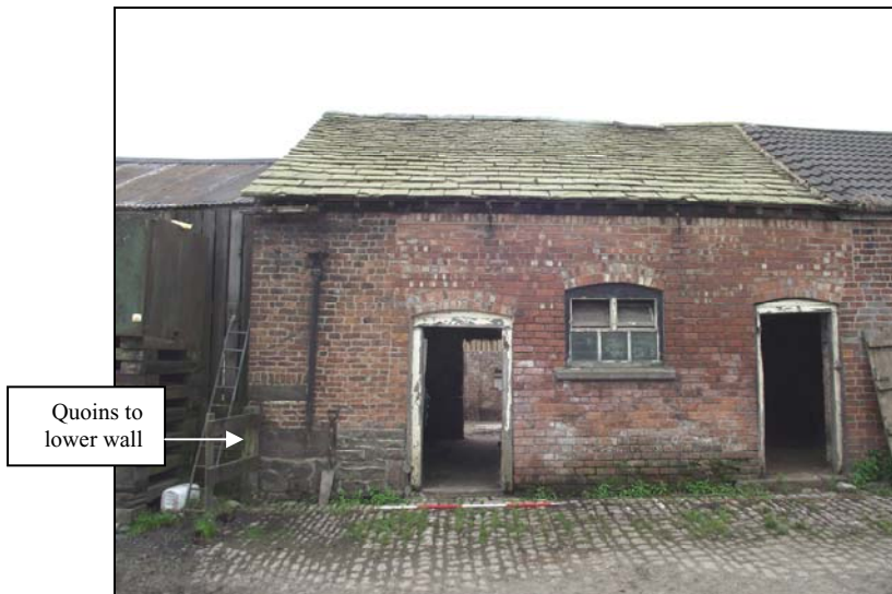
Plate 2, 4: view of the front, North Elevation (Bay 1), looking south
