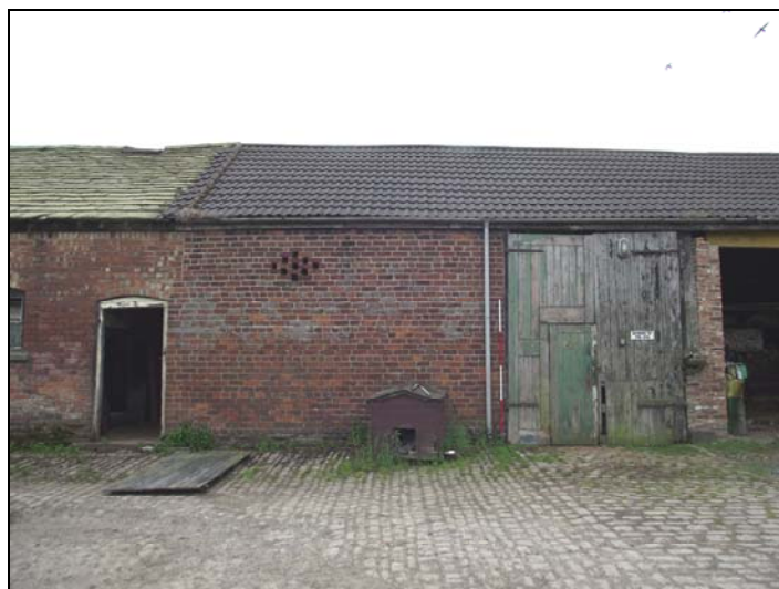
Plate 3, 5: view of the front North Elevation (Bays 2/3), looking south
