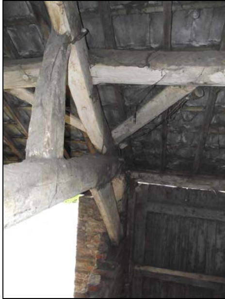
Plate 19, 58: detail of the northern side of truss T4, looking north
