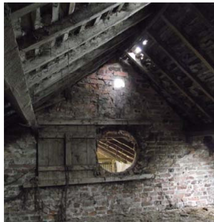
Plate 20, 47: View of the roof, truss T3, looking east
