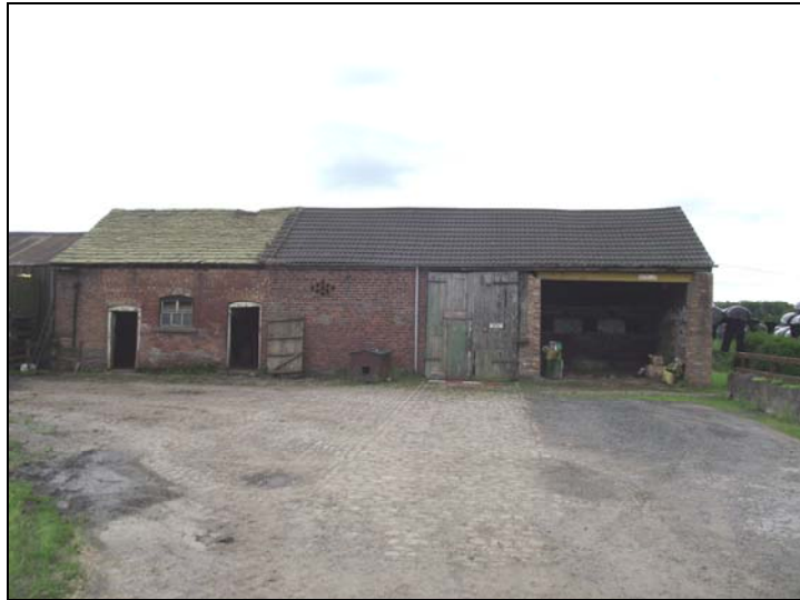
Plate 1, 1: general view of the front, North Elevation, looking south
