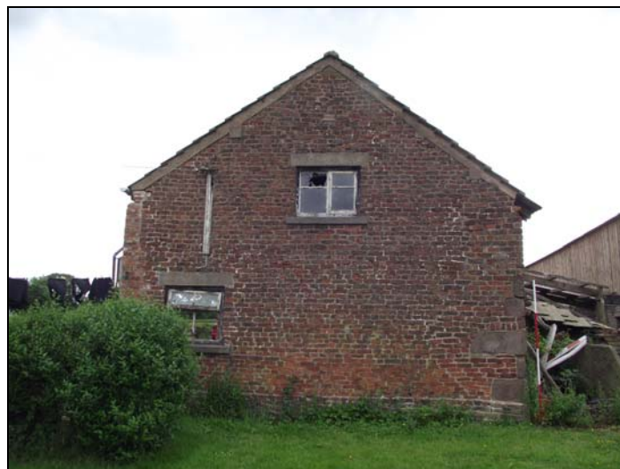
Plate 6, 9: View of the West Elevation (gable), looking east
