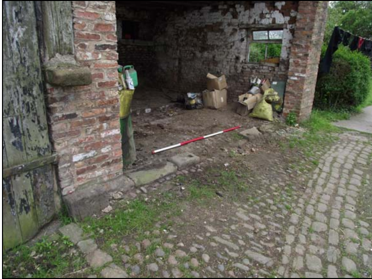
Plate 16 , 54: Oblique view of the post pads and door thresh, looking southwest
