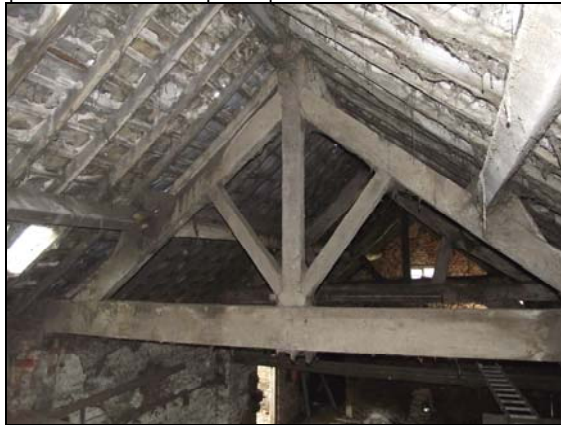
Plate 17 , 49: view of the roof truss T2, looking southwest
