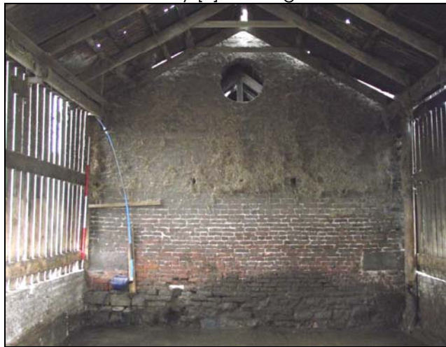
Plate 11, 22: View of the East Elevation with the circular pitching hole [6], looking west
