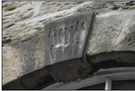
Plate 2: detail of the date stone 'built 1796'
