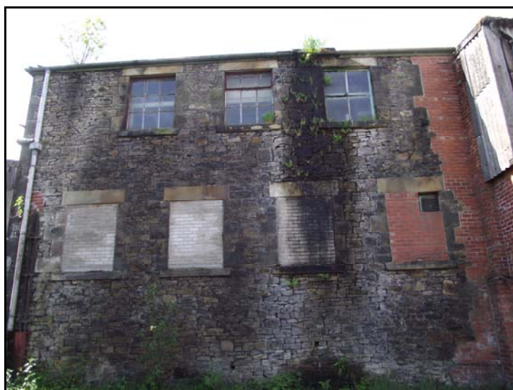
Plate 6: view of building [1G], from the northeast
