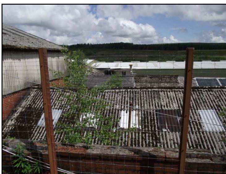
Plate 7: view across the modern asbestos sheeted roofs of the main mill building, from the southwest
