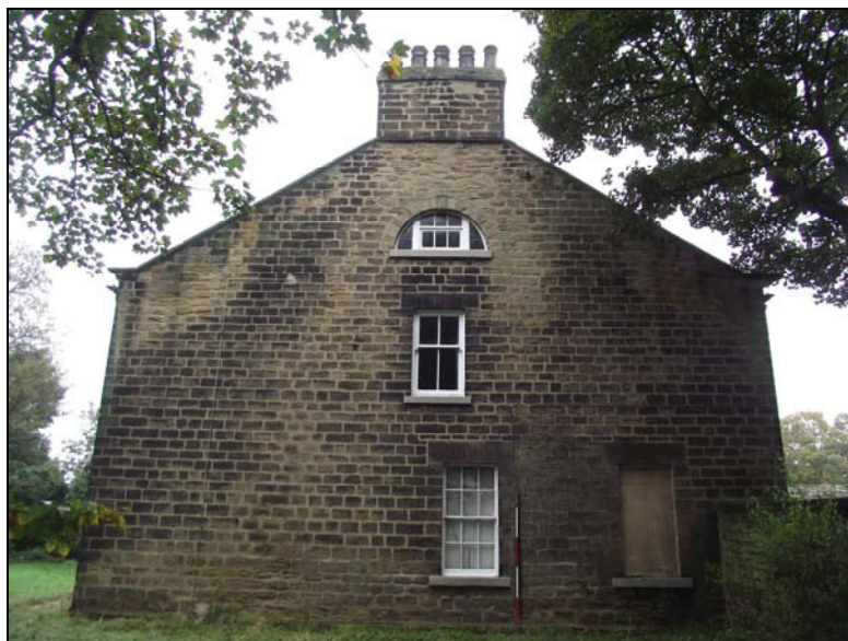
Plate 7, 162: The Southeast (gable) Elevation, from the southeast
