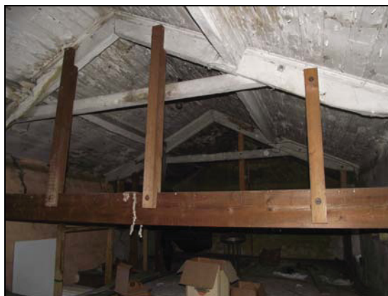
Plate 17, 88: General view of the exposed roof, from the northwest
