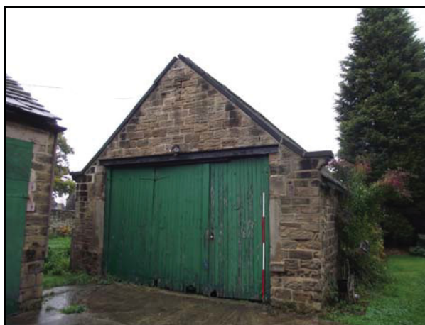
Plate 42, 129: View of the SW (gable) Elevation, from the south southwest
