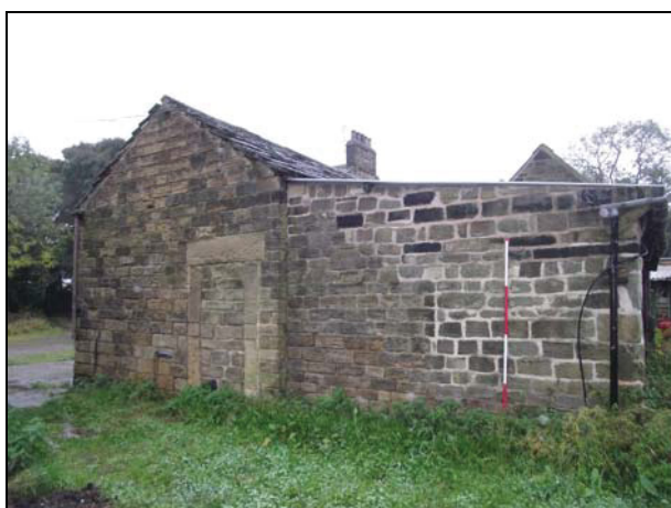
Plate 39, 109: Building C2-3, oblique view of the NE Elevation
