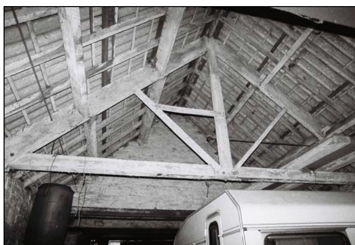
Plate 45, 126: View of the roof truss [21], from the east
