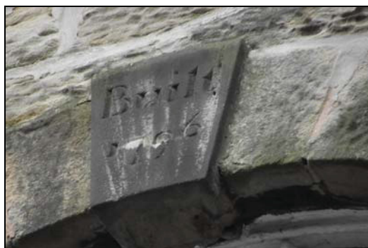
View of the date stone, to the NW Elevation
