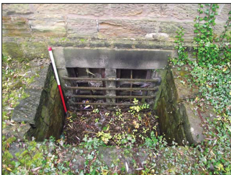
Plate 6, 155: Detail of the cellar window with defensive bars and spikes, from the northwest
