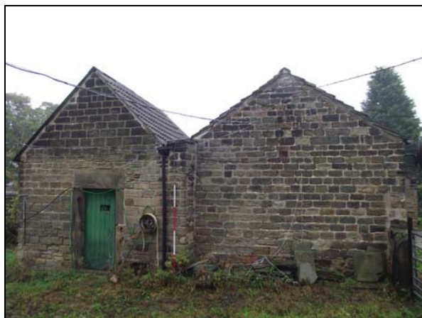
Plate 35, 104: General view of the SW Elevation, from the south southwest
