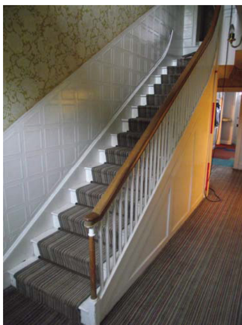
Plate 8, 21: View of the staircase, from the south
