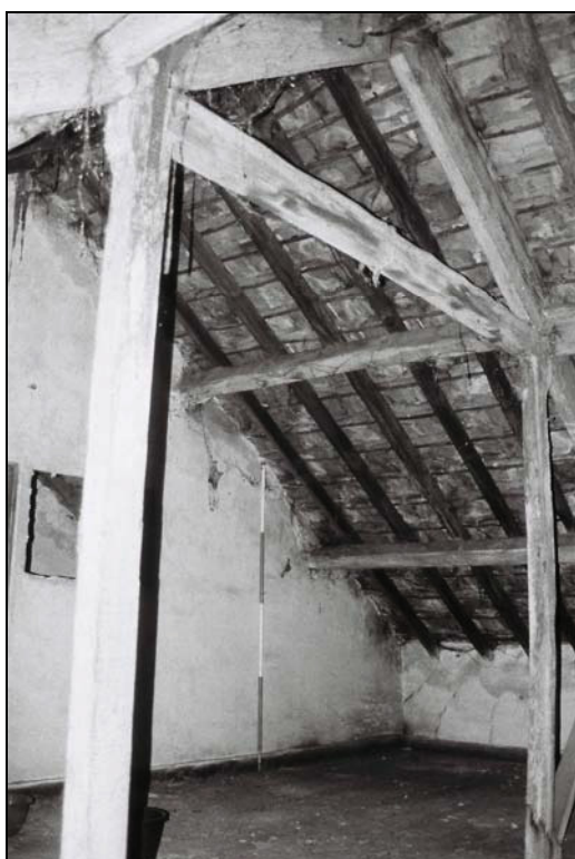
Plate 29, 74: Oblique view of the roof truss, from the southwest
