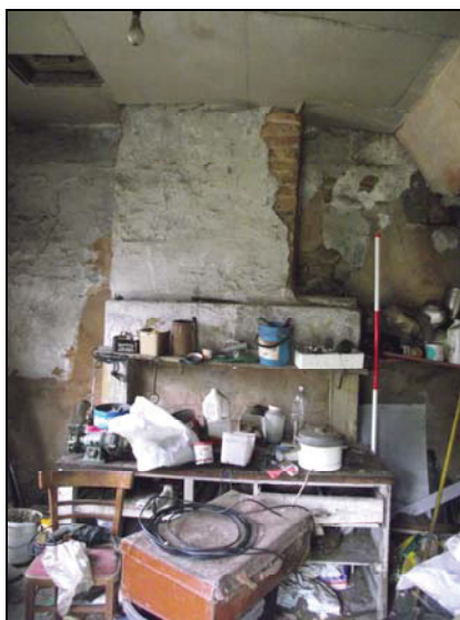
Plate 37, 96: General view towards the obscured fireplace [16], from the southwest
