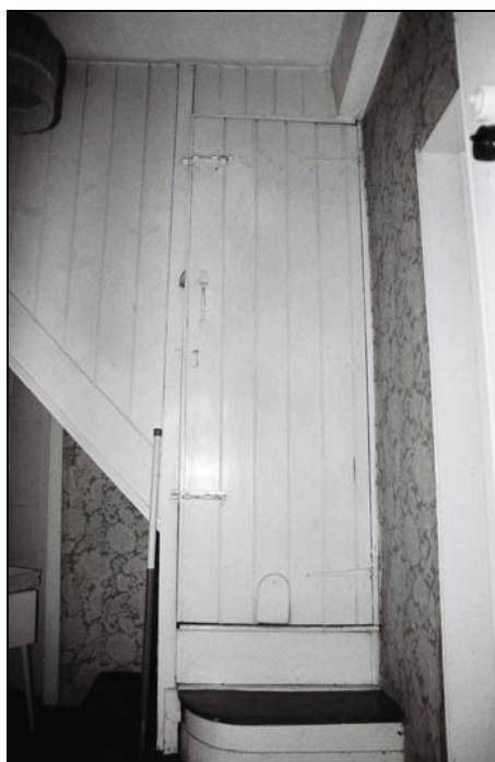
Plate 24, 141: View of the attic door with original latch, strap hinges and probably later cat flap, from the northeast
