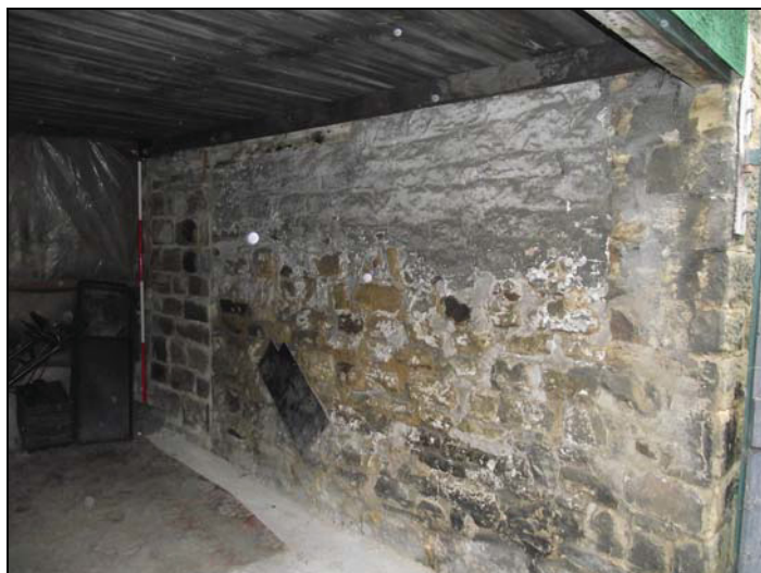
Plate 38, 114: General view of the northeast wall, with blocked doorway [18], from the south
