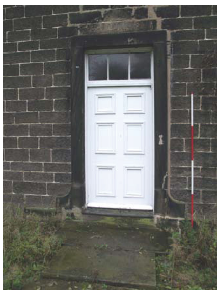
Plate 2, 161: Detail of the front door, from the south southwest
