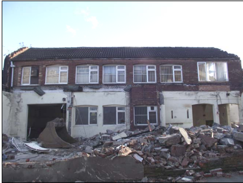
Plate 1, 64: View of Building A's, front, NW Elevation, from the northwest
