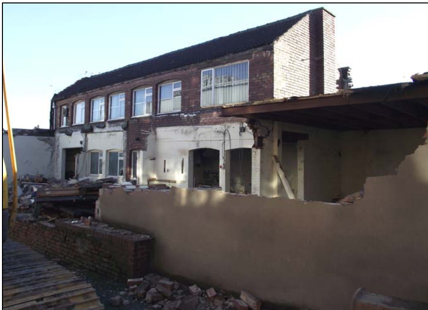
Plate 2, 58: Oblique view of Building A's NW Elevation, from the west southwest
