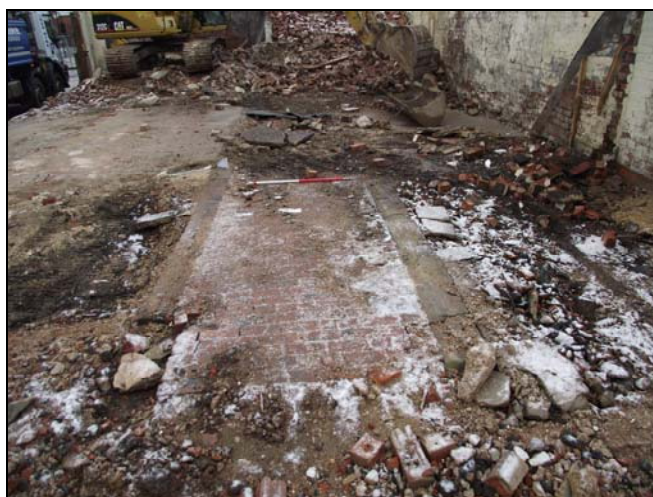
Plate 7, 77: View of the original brick set floor [B], from the southwest
