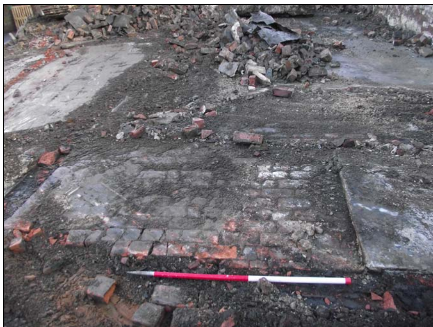
Plate 9 , 82: View of Building A's original brick set floor [D], from the southwest
