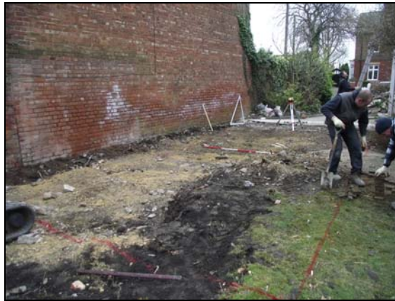
Plate 1, 2: pre-excavation view of the site, from the northeast
