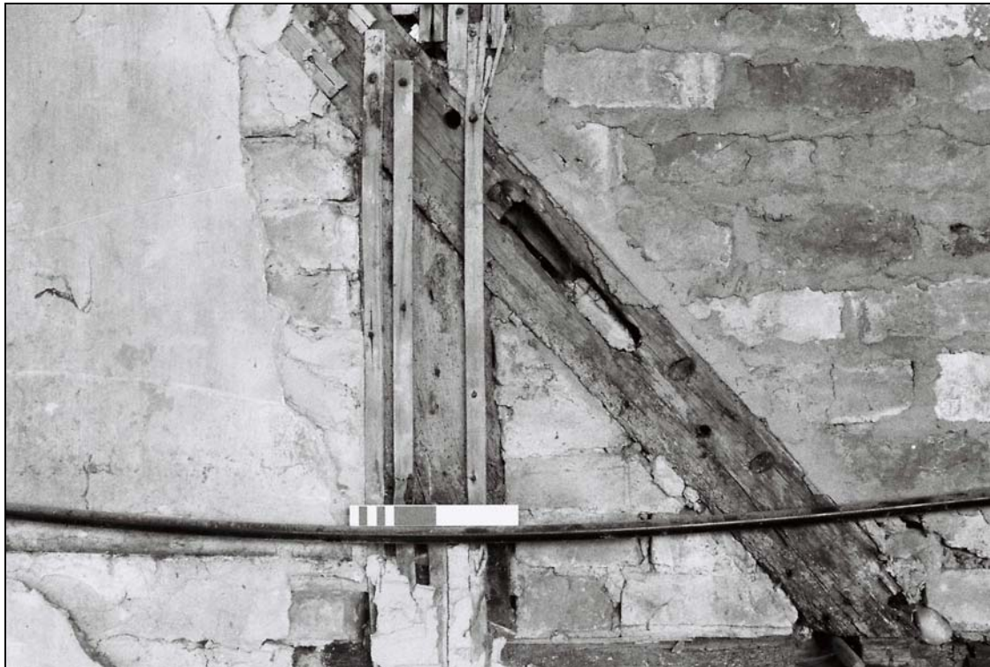
Plate 22/65: detail of the east wall (re-used straight brace), from the west
