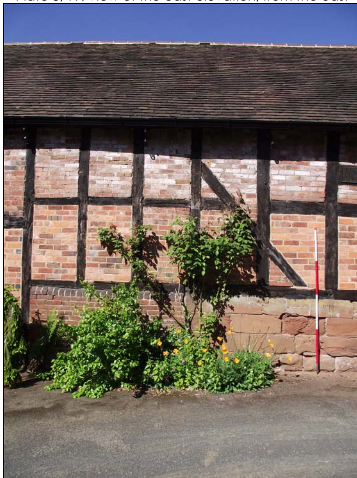
Plate 4, 21: detail of the east elevation (bays 2-3, phases 1-2), from the east
