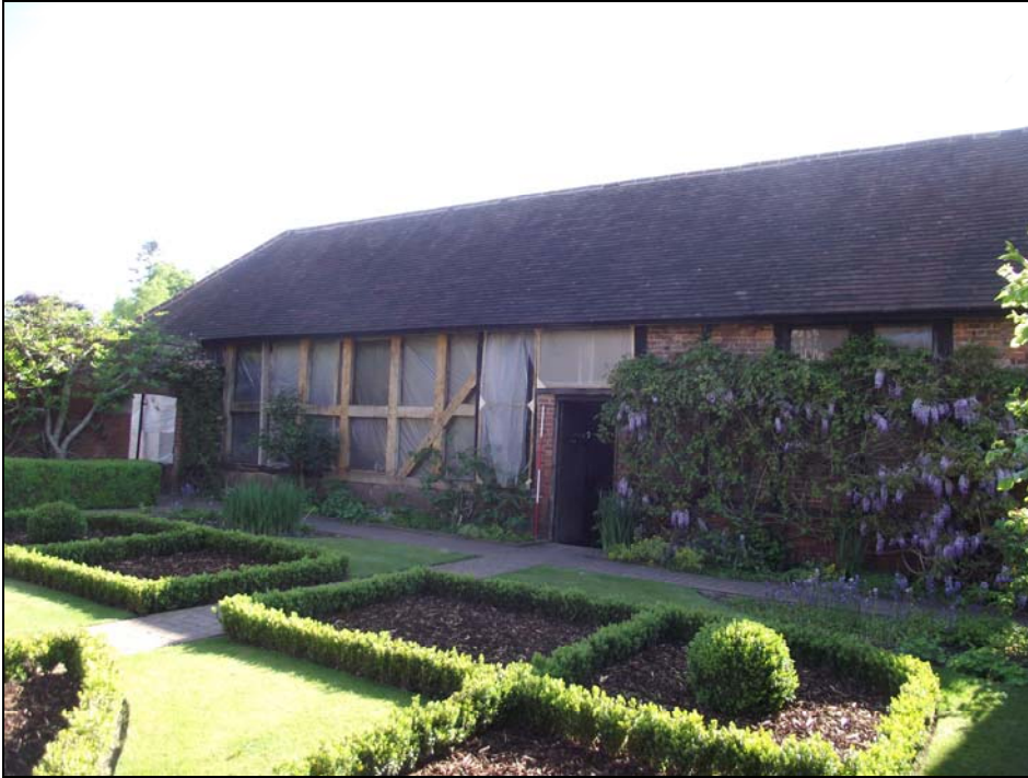
Plate 1, 8: view of the west wall with partially rebuilt oak framing, from the southwest
