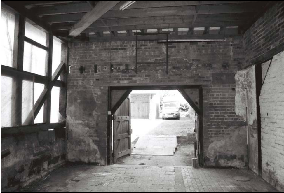
Plate 7, 17: Room 1, general view of the north wall with line of joist holes above the inserted doorway, from the south
