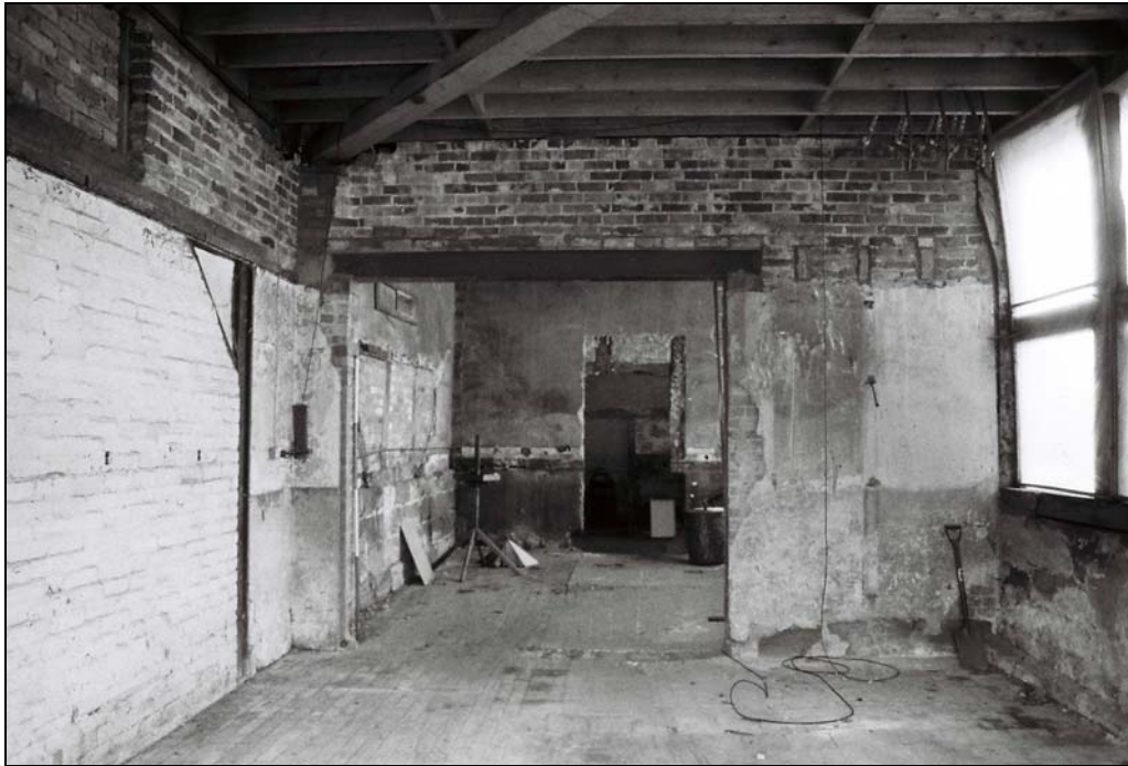
Plate 9, 13: room 1, general view of the south wall, from the north
