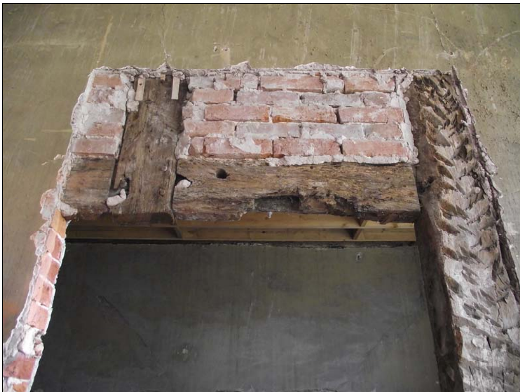
Plate 24/67: detail of the frame rail to the south wall
