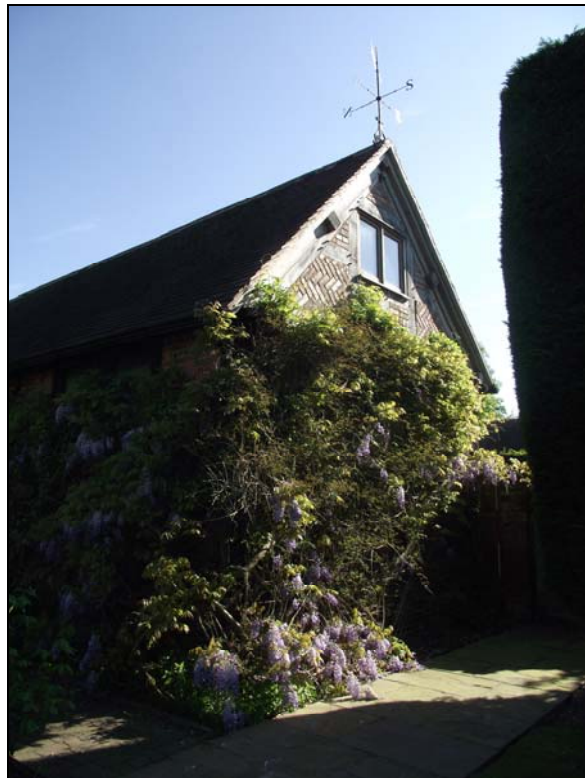
Plate 6, 10: view of the rebuilt gable wall, from the southwest
