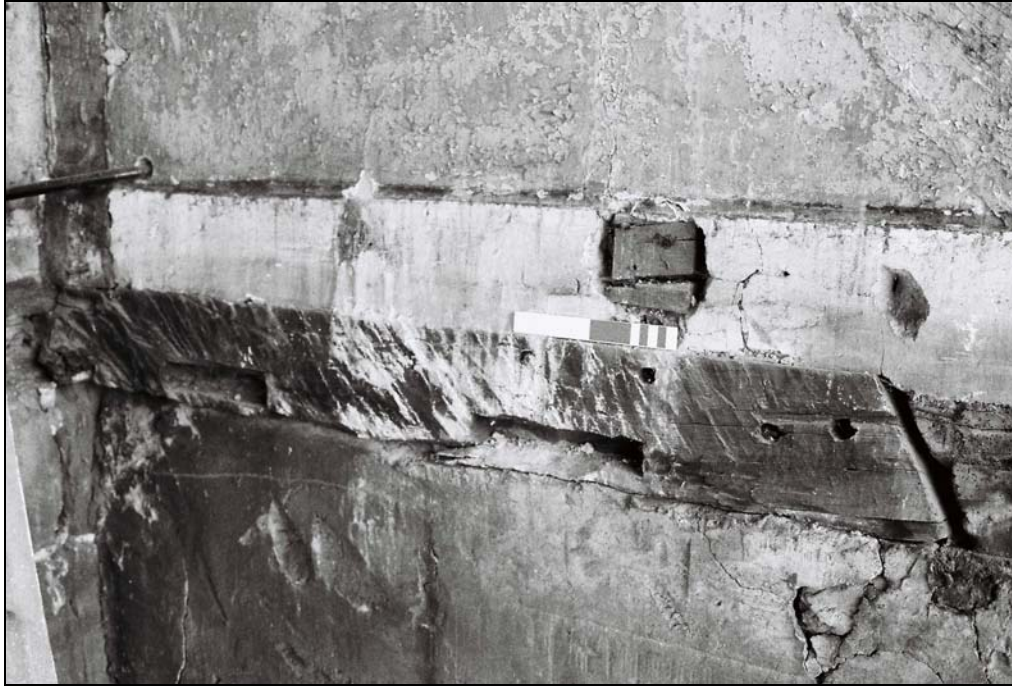
Plate 23/66: detail of the south wall (re-used sill beam), from the northwest
