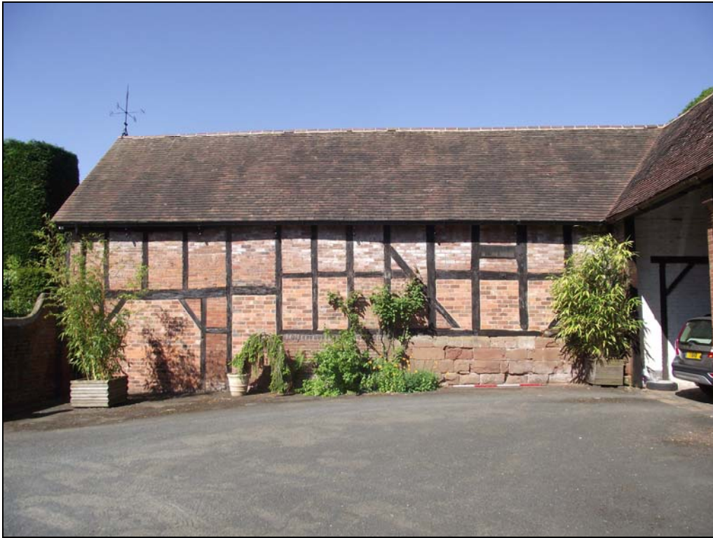
Plate 3, 19: view of the east elevation, from the east
