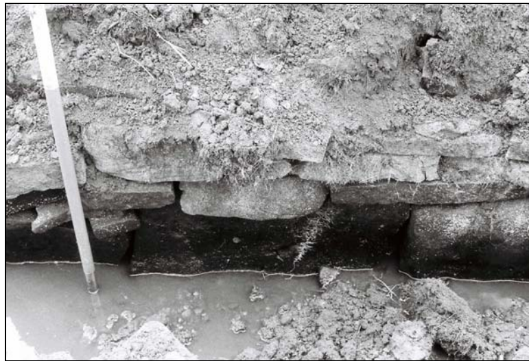
Plate 8. 23: Detail of the culvert's north facing wall with orthostats, from the north
