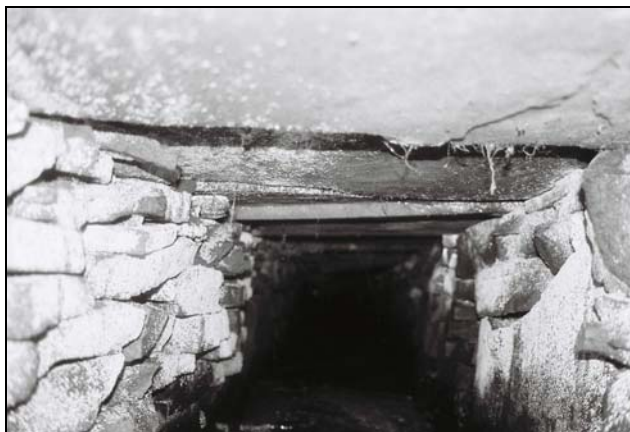
Plate 3, 6: view down the culvert, from the west
