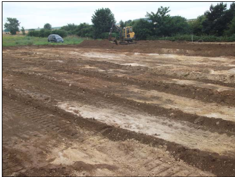
Plate 1, 7: General view, looking southwest
