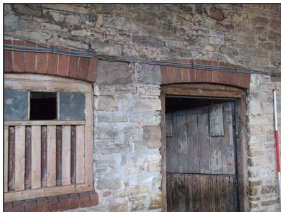
Plate 15, 15: Detail of the stables modified fenestration (Blg. E), looking northeast
