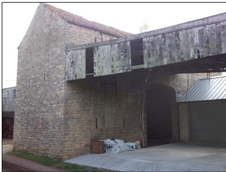
Plate 11, 11: oblique view of the obscured west elevation
