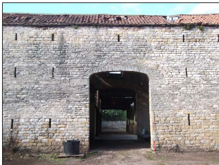
Plate 9, 9: the front east elevation (Blg C), looking west
