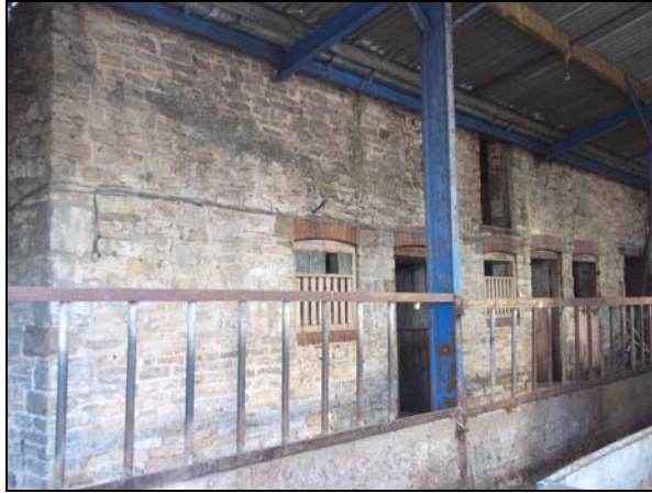
Plate 13, 13: oblique view of the front south elevation (Blg. E), looking northeast
