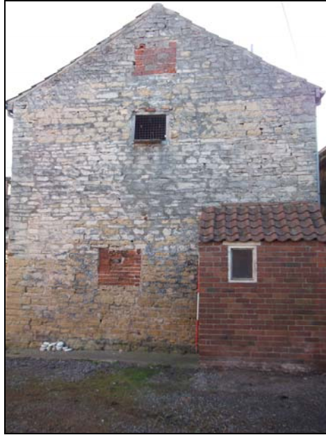
Plate 7, 7: view of the rear gable (Blg B), looking east
