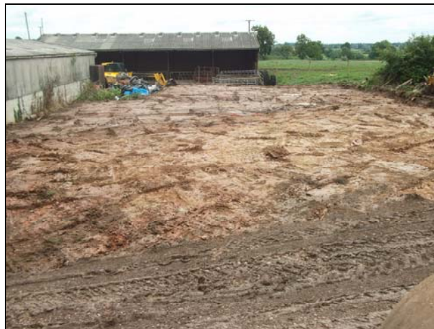
Plate 6, 11: general view of the stripped PDA, looking east
