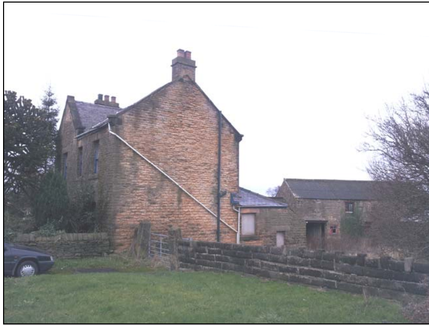
Plate 22: view of the side of the farmhouse (Bldg. A), with walls J & K, looking west
