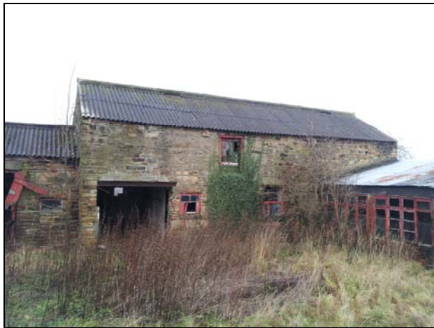
Plate 15: the barn (Blg. F), view of the front elevation, looking northwest
