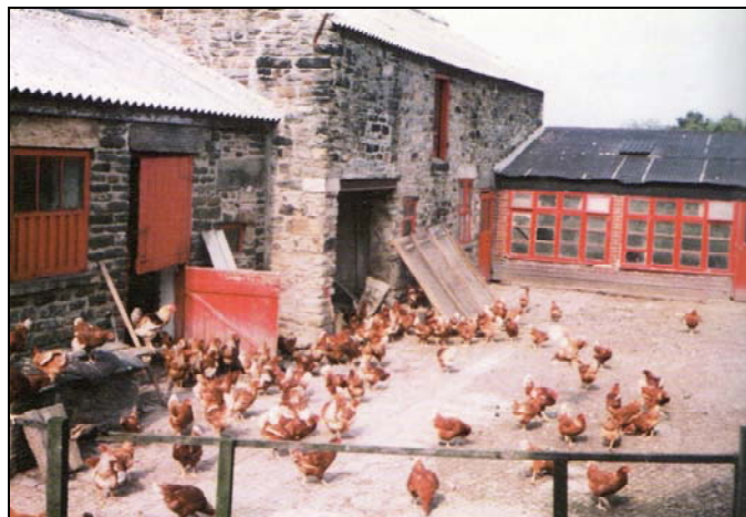
Plate 6: Further view of the farmyard probably c. 1979 (Hanson 2010, 48) oblique view of buildings E, F & G, looking north northwest
