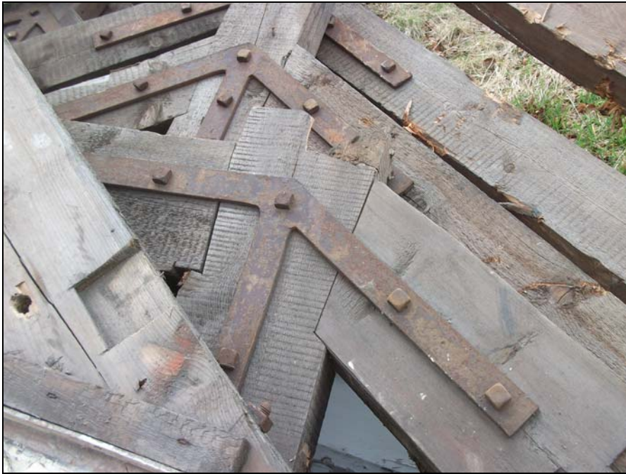
Plate 15, 74: detail of the type 3 upper truss, from the east
