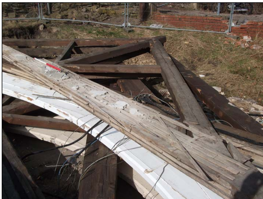
Plate 12, 53: view of the removed roof type 1 roof truss
