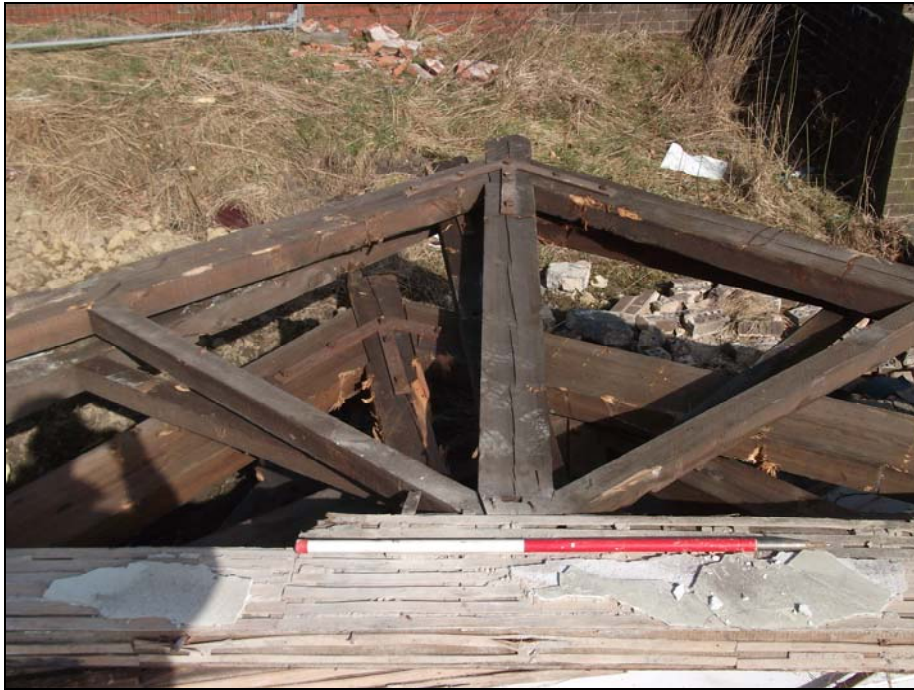
Plate 13, 54: view of the removed roof type 1 roof truss
