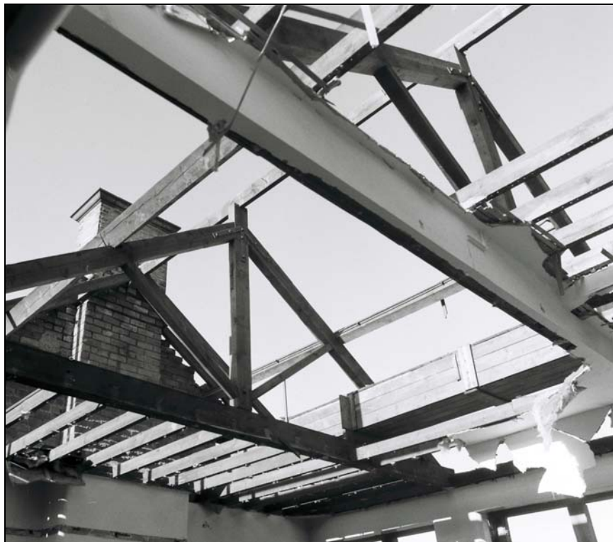
Plate 10, 9: view of the type 1 roof trusses, from the west
