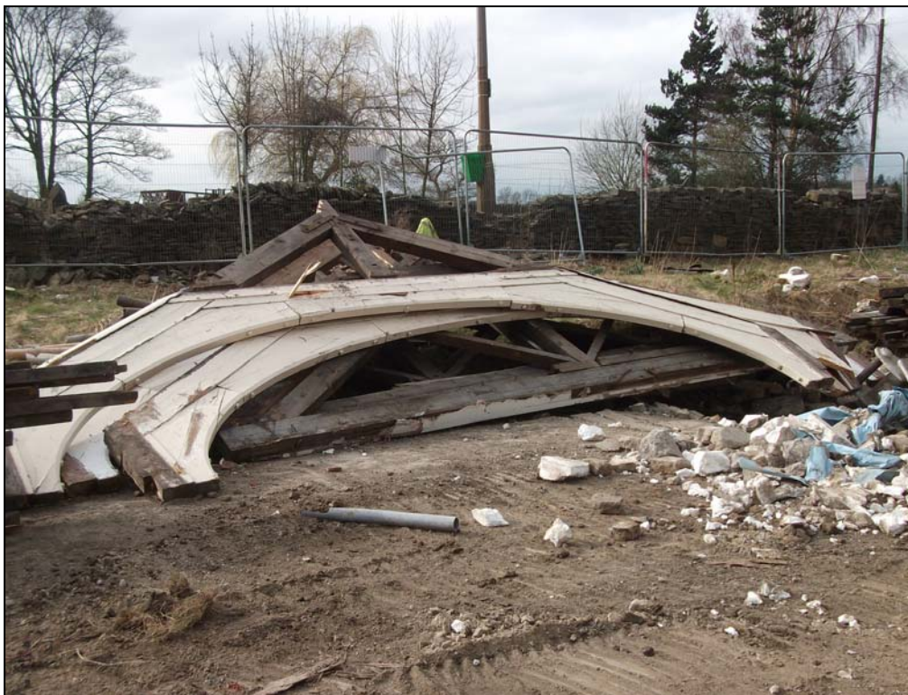
Plate 14, 73: view of the removed type 2 roof trusses, from the east
