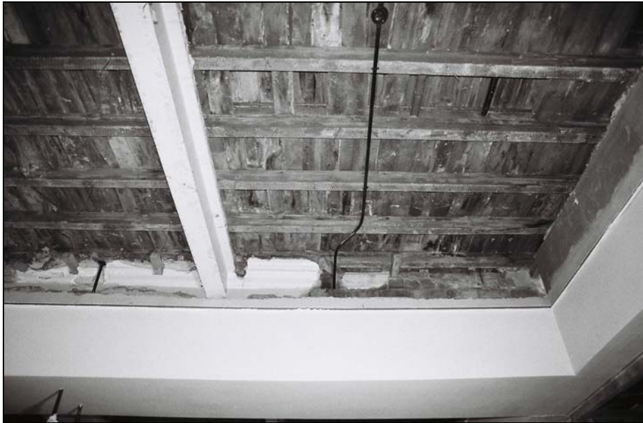
Plate 3, 18: room 15, view of the revealed ceiling/first floor arrangement, from the northeast
