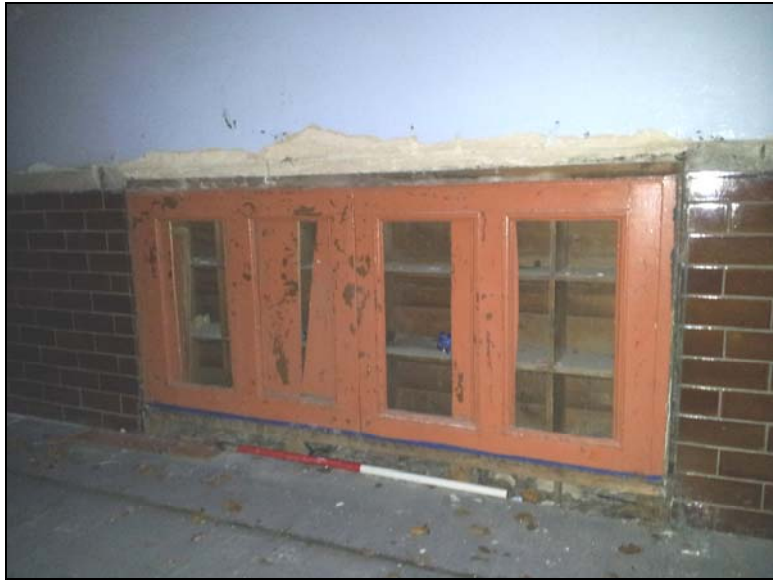
Plate 1, 16: room 49, view of the southern built in cupboard, from the west
