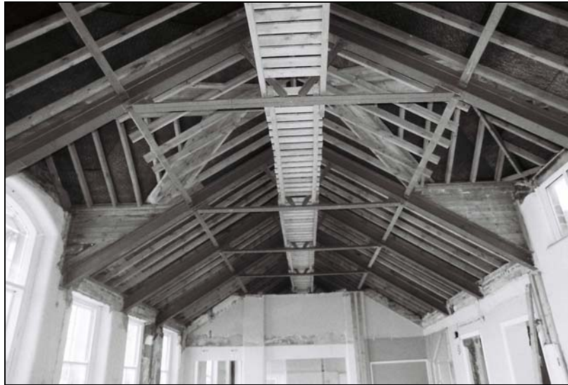
Plate 9, 33: view of the modern roof, from the northeast
