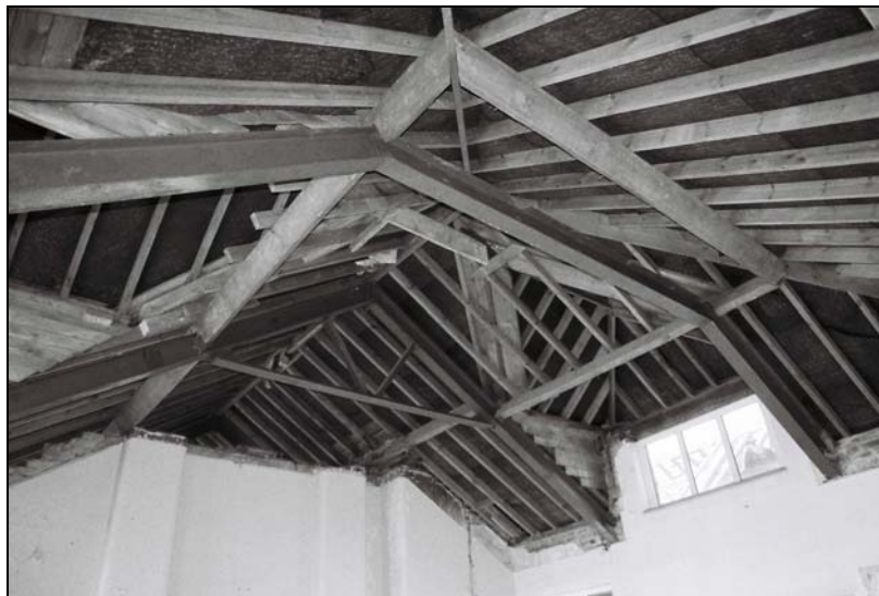
Plate 8, 31: view of the modern hipped roof, from the east
