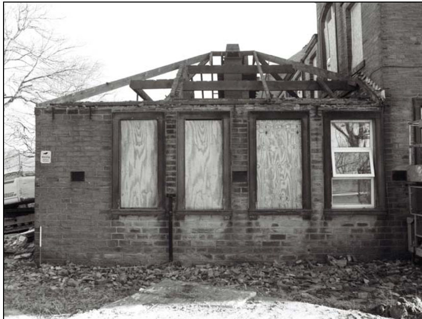
Plate 7, 1: view of the single storey kitchen's SW elevation, from the southwest
