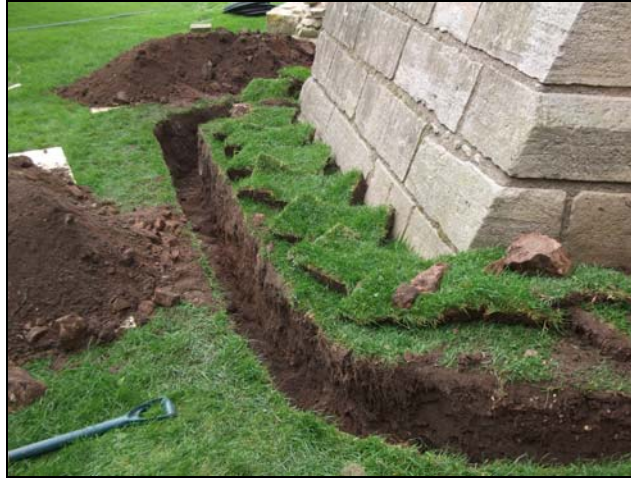
Plate 3, 3: general view of the cable trench, from the northeast
