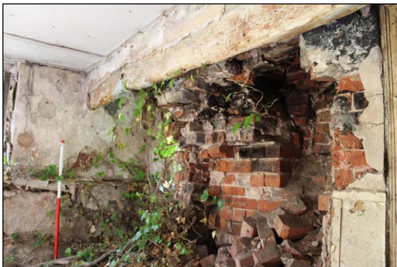
Plate 17, 79: oblique view of the small brsummer beam [Q] with slope made bricks above, looking west
