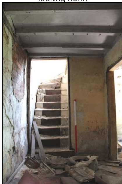
Plate 14, 24: room 2, general view towards the staircase (Rm. 6), looking south southeast
