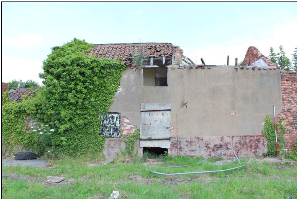
Plate 9, 13: view of the rear SW Elevation, looking east northeast
