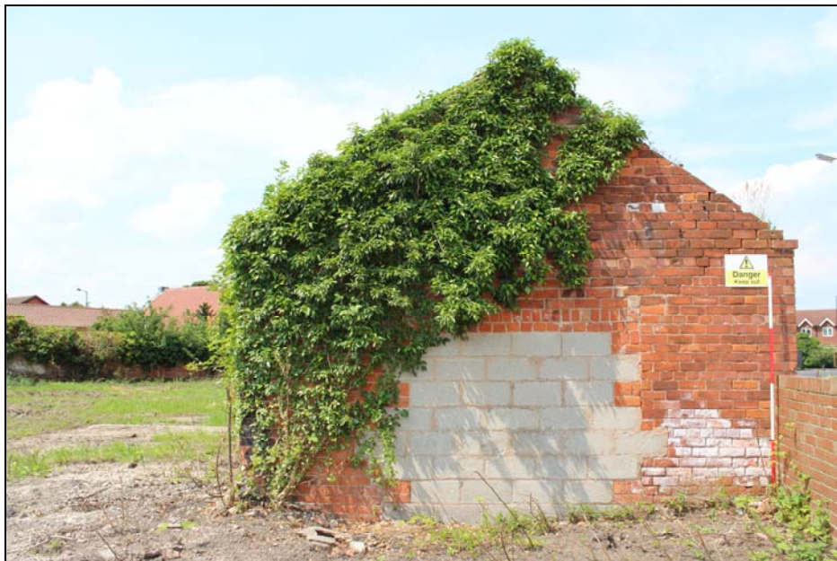
Plate 5, 8: view of the garage gable, looking north northwest
