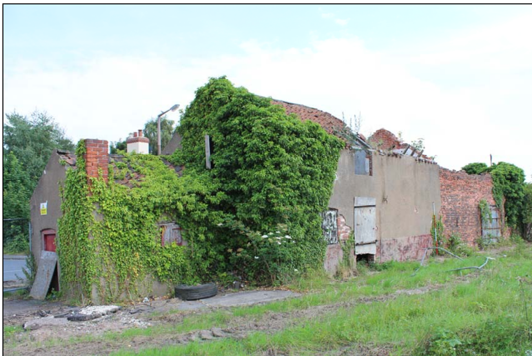
Plate 10, 14: general oblique view of the rear SW Elevation, looking south southeast
