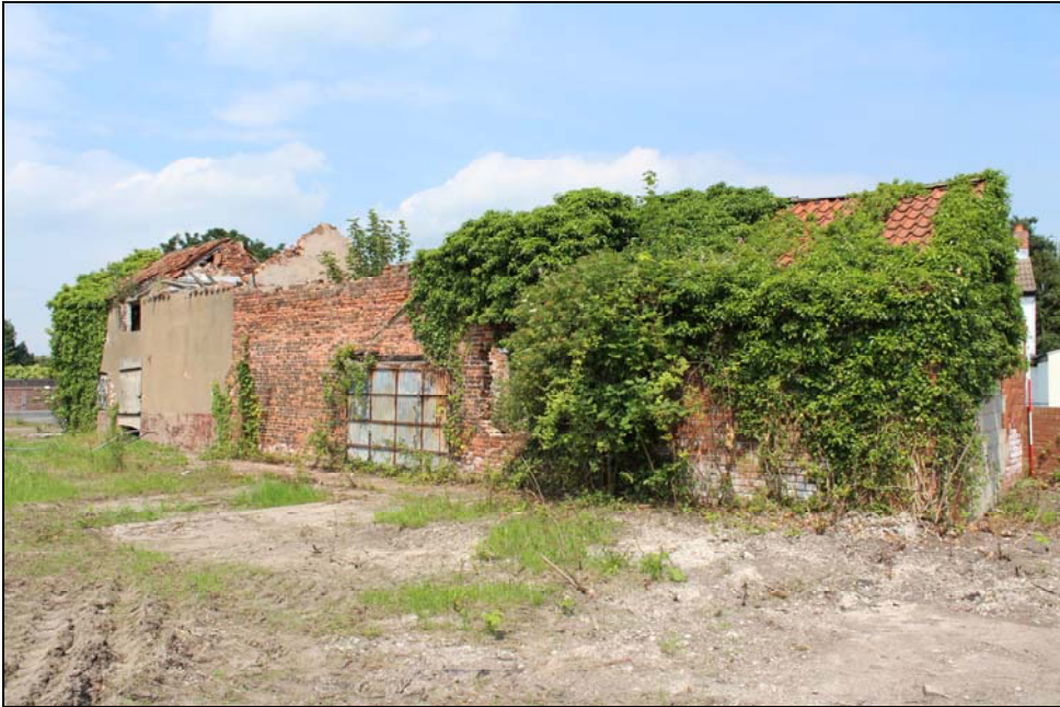
Plate 6, 9: general oblique view of the rear SW Elevation, looking north northeast
