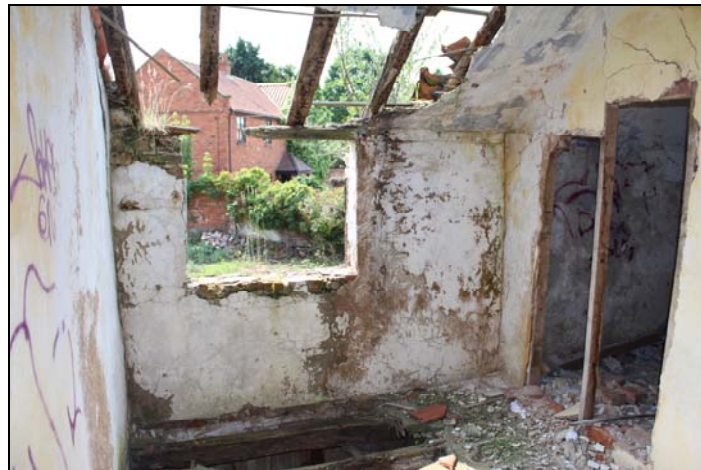
Plate 25, 26: room 8, general view with exposed stud wall, looking southwest
