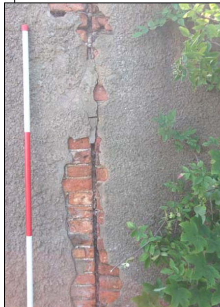
Plate 3, 62: Vertical building line between the house (Blg. A1 and the extension (Blg. A2) looking southwest
