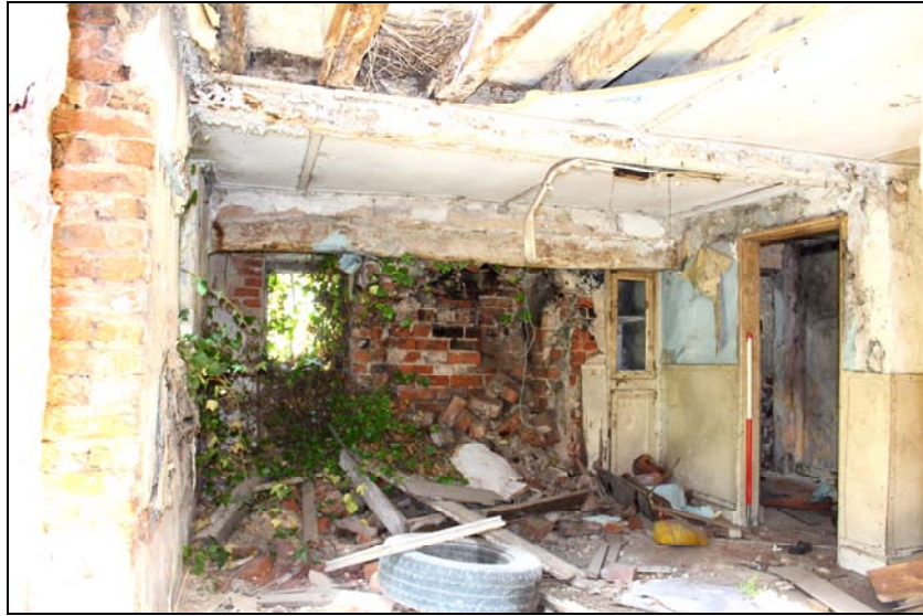
Plate 15, 44: room 3, view of the Kitchen from the Parlour (Rm. 4), looking north
