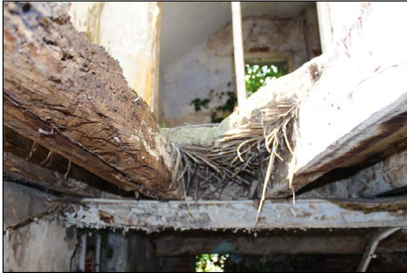
Plate 16, 46: room 3, detailed view of the ceiling showing the reeds and limecrete floor, looking north northwest
