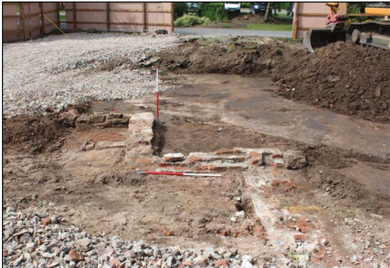
Plate 13, 59: detailed view of the building footings, from the east northeast
