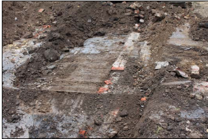
Plate 6, 48: Excavation views of the front (SE facing) conservatory wall, from the east northeast
