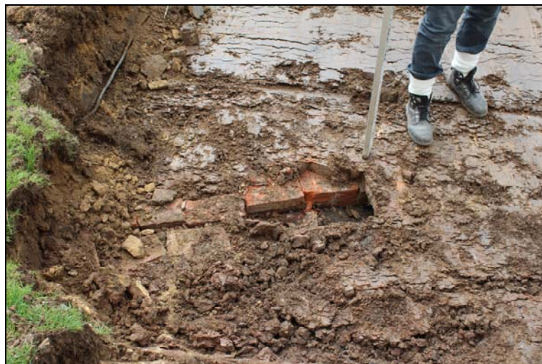
Plate 11, 77: View of the exposed culvert [319], from the north northwest
