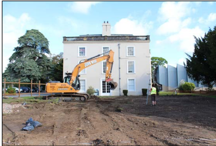
Plate 3, 40: Pre-excitation view of the PDA, from the south southeast
