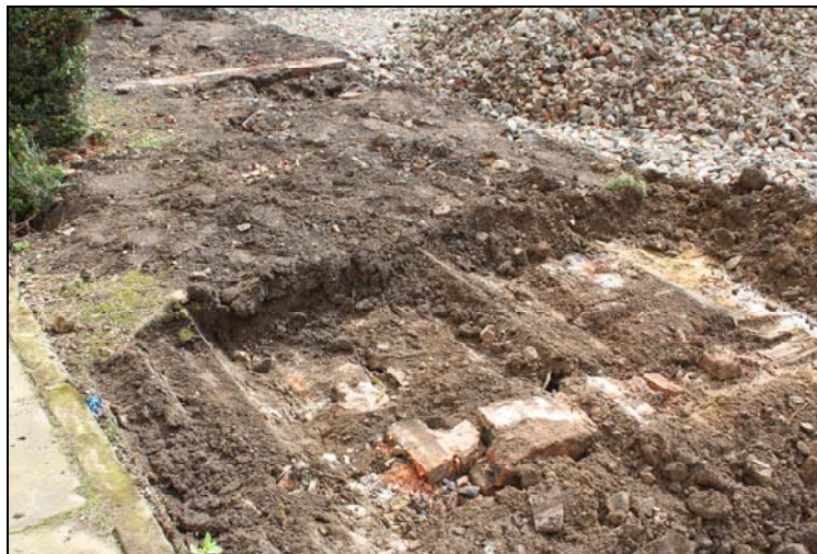
Plate 10, 79: View of the water cistern [311], from the northwest
