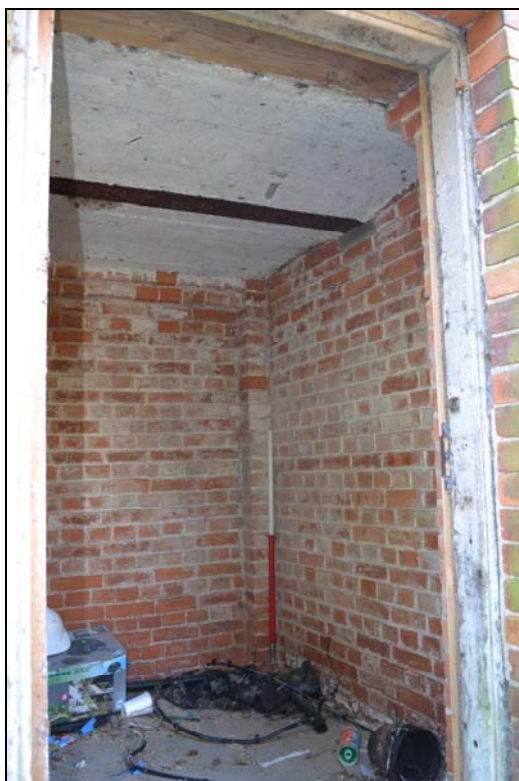
Plate 8, 18: the tower, internal view of the tower's ground floor, looking west
