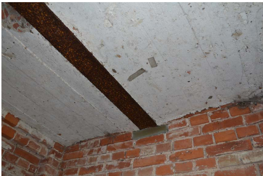
Plate 9, 19: the tower, detail of the ceiling, looking west
