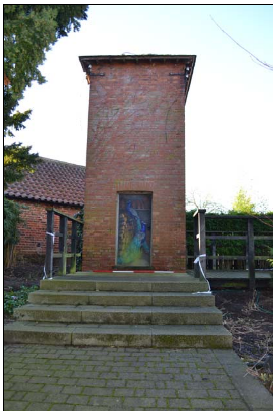
Plate 3, 1: the tower, view of the northeast elevation, looking southwest
