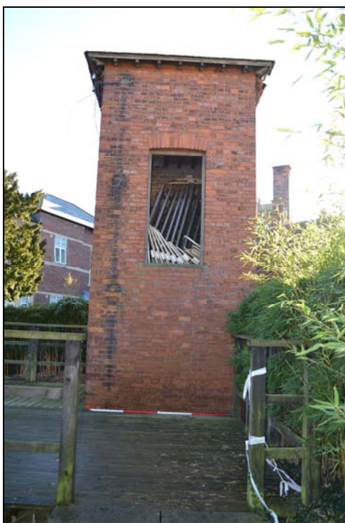
Plate 5, 3: the tower, general view of the northwest elevation, looking southeast
