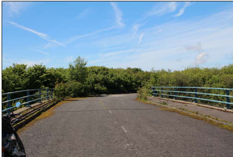
Plate 5, 5: view across the test track bridge, looking west
