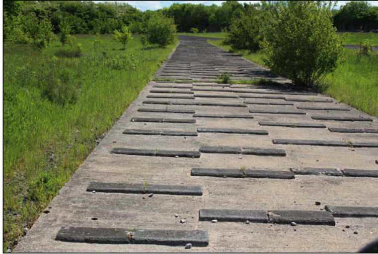
Plate 7, 10: a section of rumble track (F) with staggered concrete strips, looking south south-east
