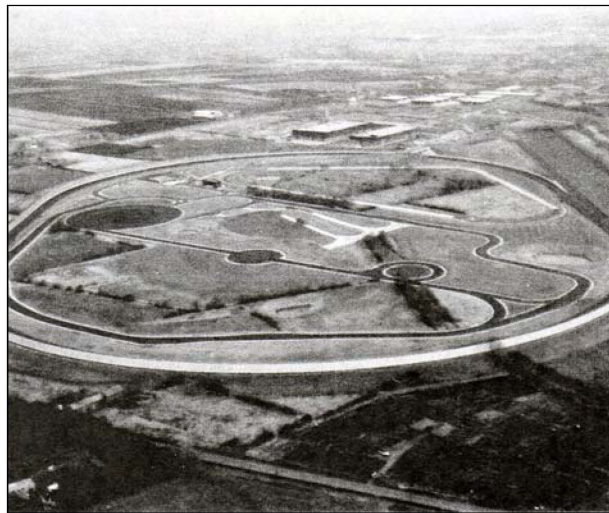
Aerial view of the test track from the south-west
