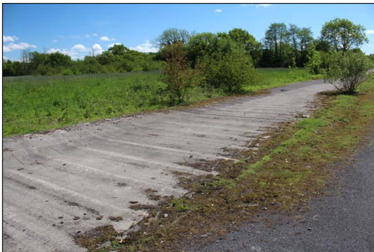
Plate 11, 19: corrugated concrete surface to the inner 'rumble' track, looking south-east
