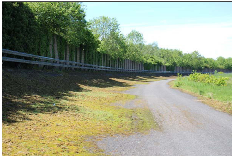
Plate 2, 24: the outer speed track with embanked sides, crash bars and sectional concrete fence, looking north-west
