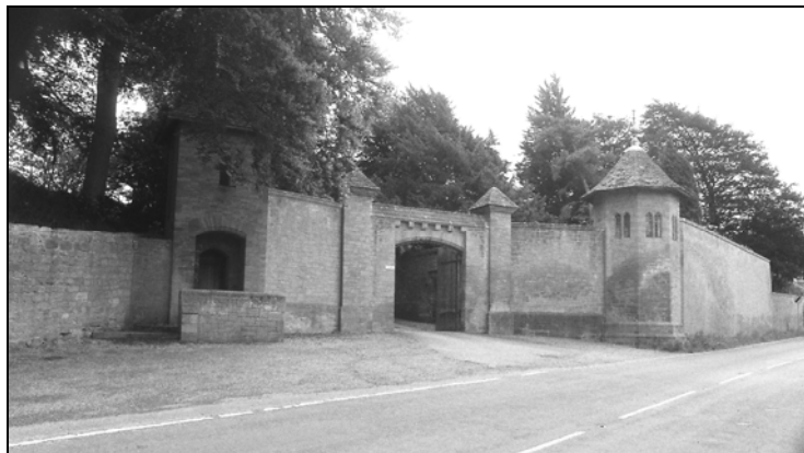
Plate 20, 10-9: general view of the gateway, looking south [1]
