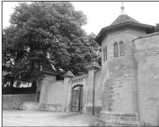
Plate 4, 32-37: general oblique view of the gateway, looking north-east [1]
