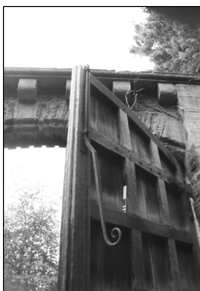
Plate 15, 16: detail of the latch [5f] (0.2m scale)
