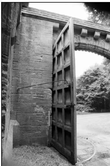
Plate 13, 18: general view of the southern gate [5e, 5f]
