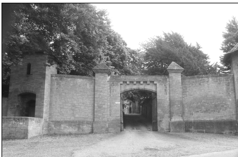
Plate 21, 8-7: general view of the gateway, looking south-east [1]
