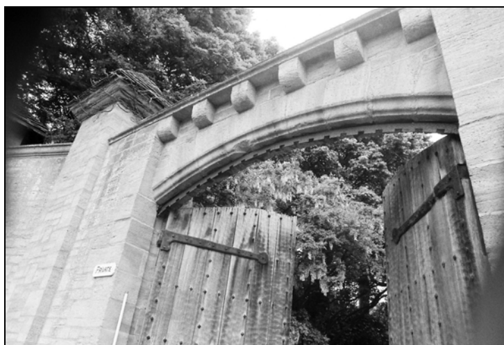
Plate 7, 29: detail of the brattished iron detail within the stone arch above the gates, looking north-east [2]
