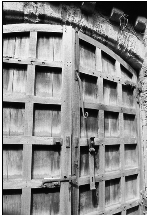
Plate 11 , 24-22: view of the latch, brace and bolt looking north-west [5b]
