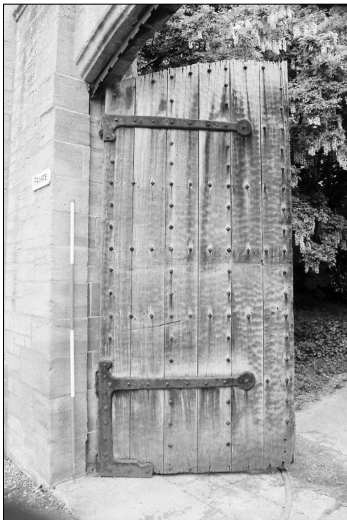
Plate 6, 30: detail of the gate door adzed surface of the oak cladding boards, looking north-east [4]
