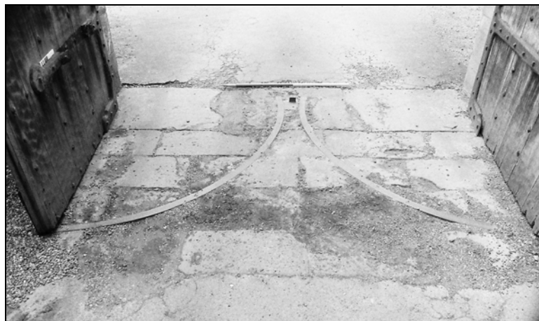
Plate 19, 12: view of the iron gate-runner [5f]
