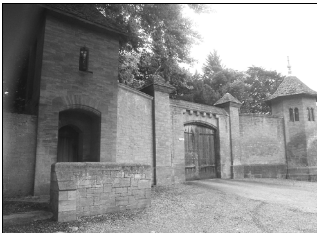
Plate 1, 36: general view of the gateway, looking south [1]
