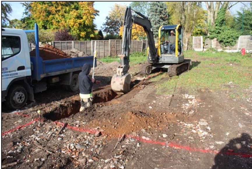
Plate 2: excavation view of the site, looking north
