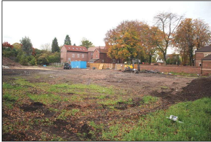
Plate 1: pre-excitation view of the site, looking southeast
