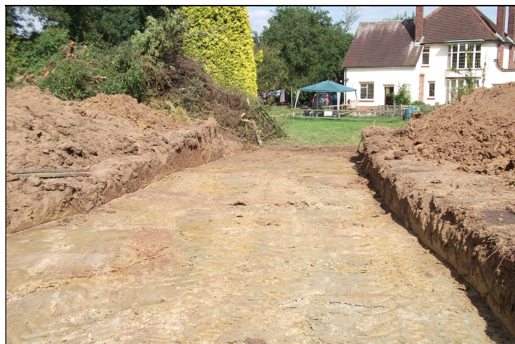
Plate 3: view of the excavated formation level of the driveway, looking east
