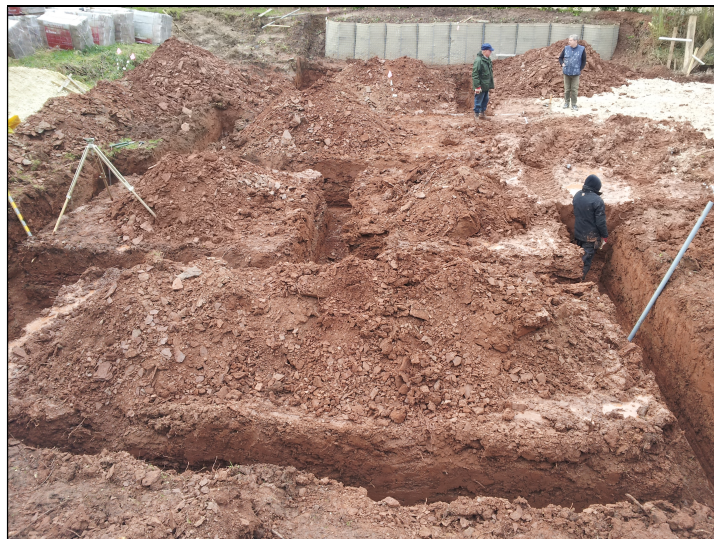
Plate 12: plot 4, excavation view, looking west
