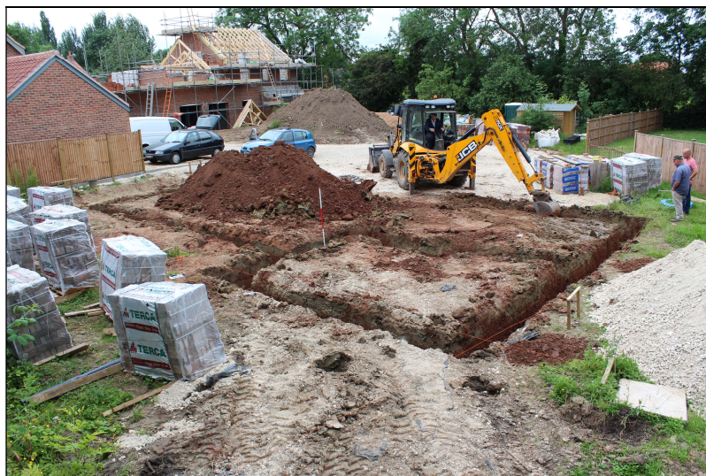
Plate 9: Plot 3, post excavation view, looking northwest
