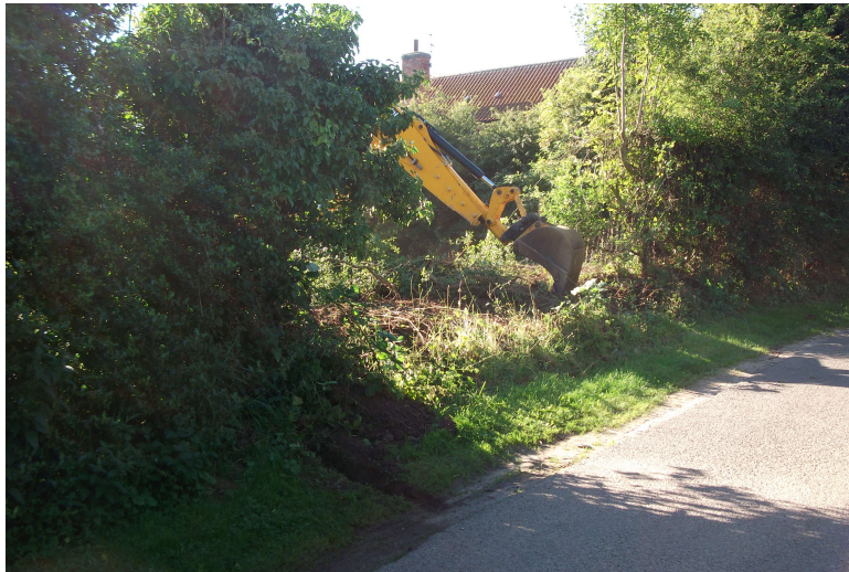
Plate 1: excavation of the driveway, looking south southeast
