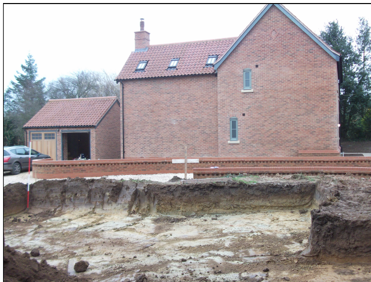
Plate 5: Plot 1, post-excavation view, looking south
