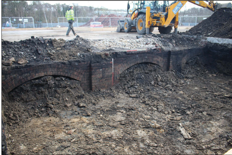
Plate 10: oblique view of the exposed wall, from the west
