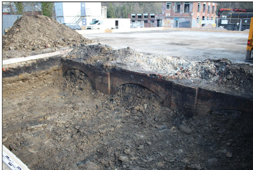
Plate 9: oblique view of the exposed wall, from the west
