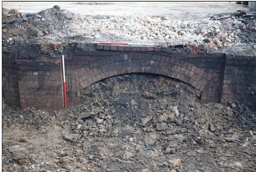
Plate 8: detail of the exposed wall (central arch), from the west
