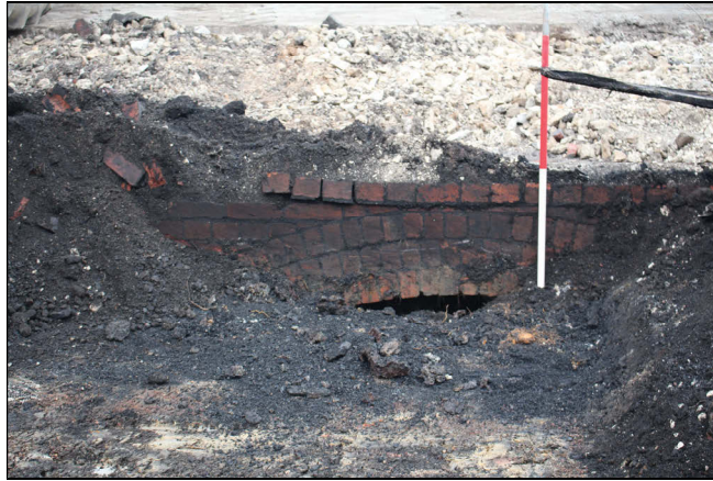
Plate 7: view of the upper part of an exposed arch, from the northwest
