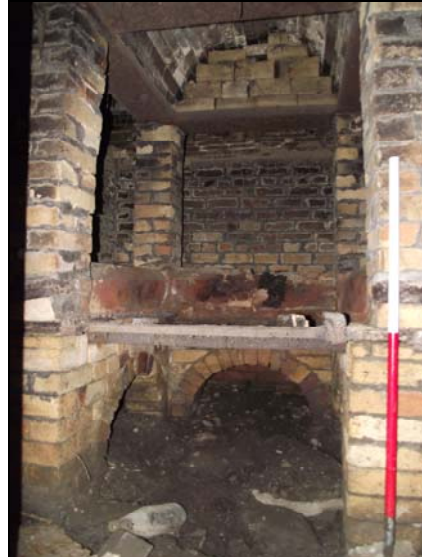
Plate 21, 94: View of the corn dryer defined by brick columns and arched heating ducts, from the west
