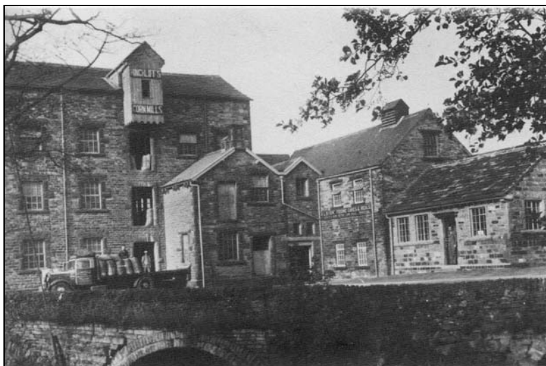
Plate 3: The front Northeast Elevation c. 1930, with the arched millstream in the foreground, from the east (Brownbill 1987, 71).
