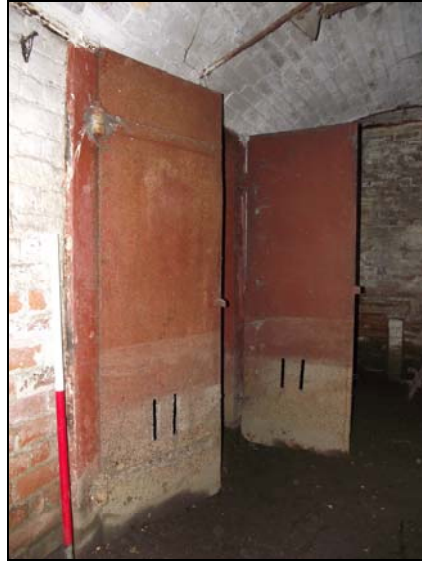
Plate 22, 226: View of the iron doors to the dryer, from the northwest
