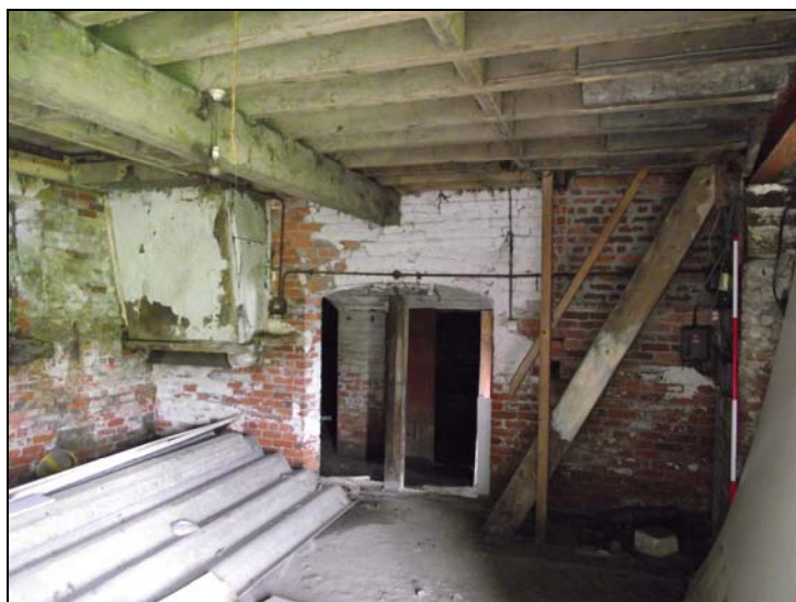
Plate 16, 87: General view, from the southwest
