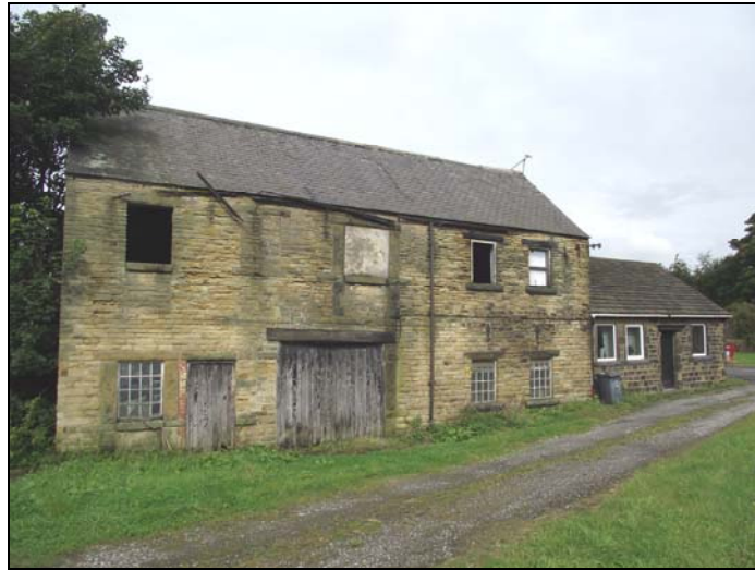
Plate 6, 82: General view of the mill's, front South Elevation, from the southwest
