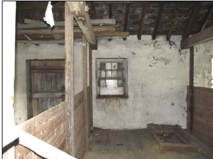
Plate 26, 100: View of the central storeroom with original opening to the hopper that controlled descending grain into sacks, from the south southeast
