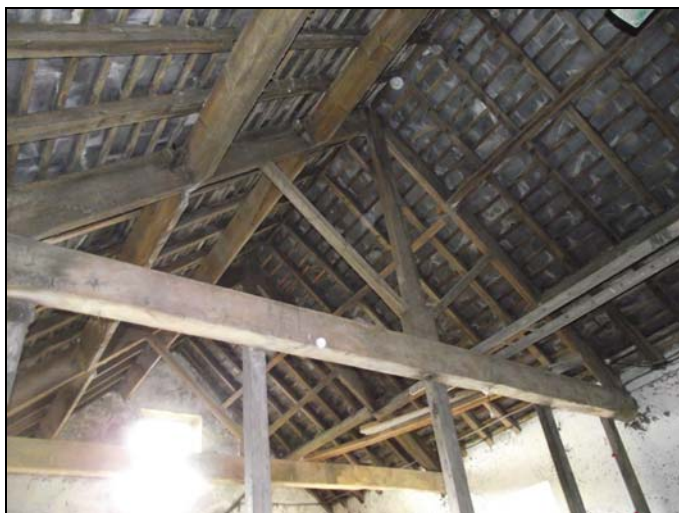
Plate 28, 216: View of the king-post roof truss, from the east
