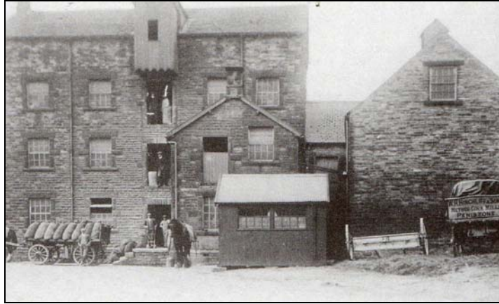
Plate 4: Further earlier view of the front of the mill with its external hoist and loading doors, with late 19 th century extension (Blg. H: [14]) to the right, from the northeast (Hey 2002, 52)
