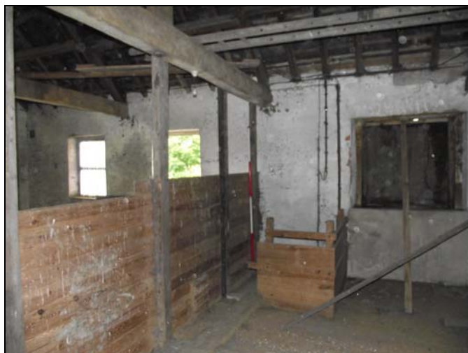
Plate 27, 215: View of the central storeroom with inserted ladder, from the north
