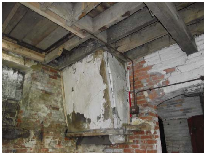
Plate 19, 214: view of the stone chute, from the southwest
