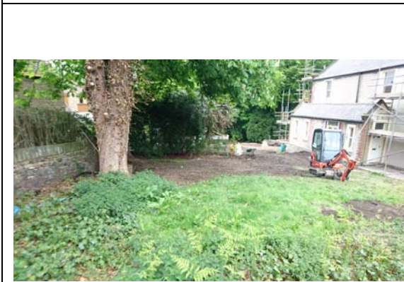
Plate 27: view of PDA 4, looking NE
