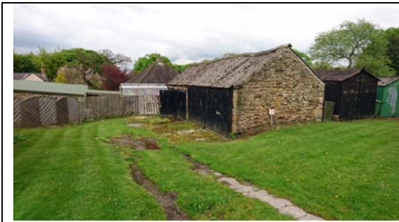
Plate 11: view of PDA 3, with the open sided shed, looking NE
