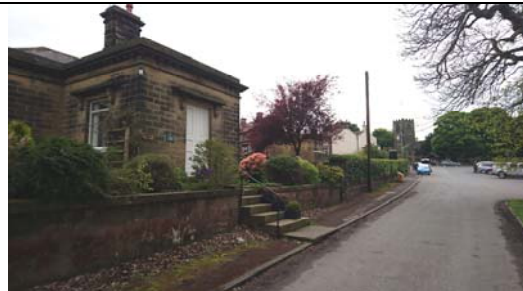
Plate 14: view of Top Lodge [10], looking W
