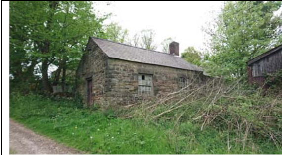
Plate 23: view of PDA 10, with gabled shed, looking W
