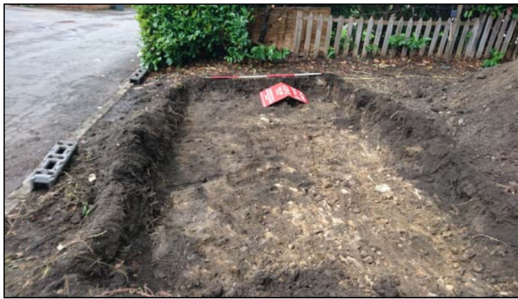
Plate 5: post excavation view of the southern half of the site, looking northeast
