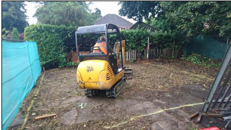
Plate 2: pre-excitation view of the site, looking southwest
