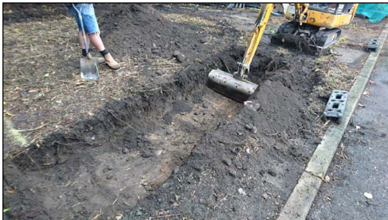
Plate 3: excavation view of the site, looking northeast
