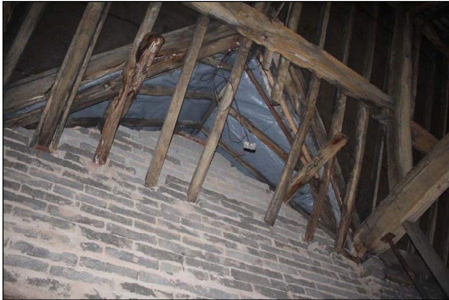
Plate 17, 47: View of the roof junction blds. B & C, from the west
