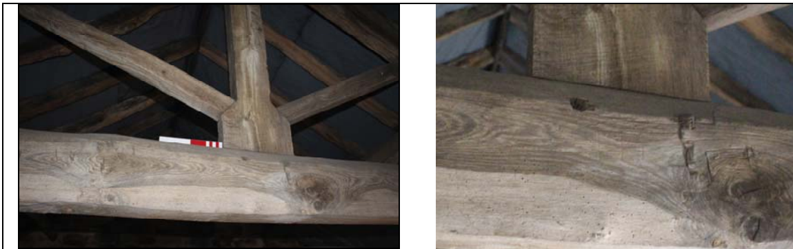
Plate 9, 21: Rm. B.2, detail of feint carpenter's mark 'IIII' to the tie-beam and strut, from the west
