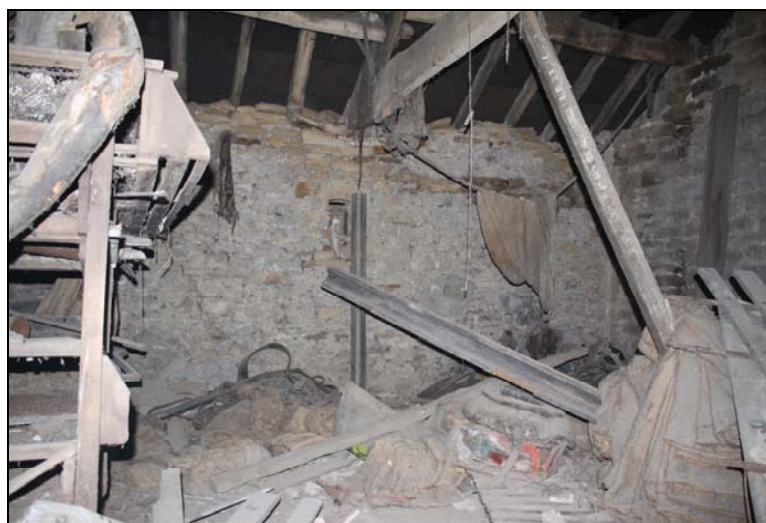
Plate 26, 75: D.3, general obscured view, from the east
