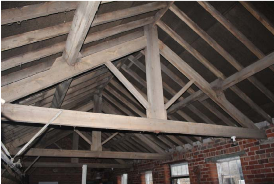
Plate 40, 104 : general view of the roof, from the east
