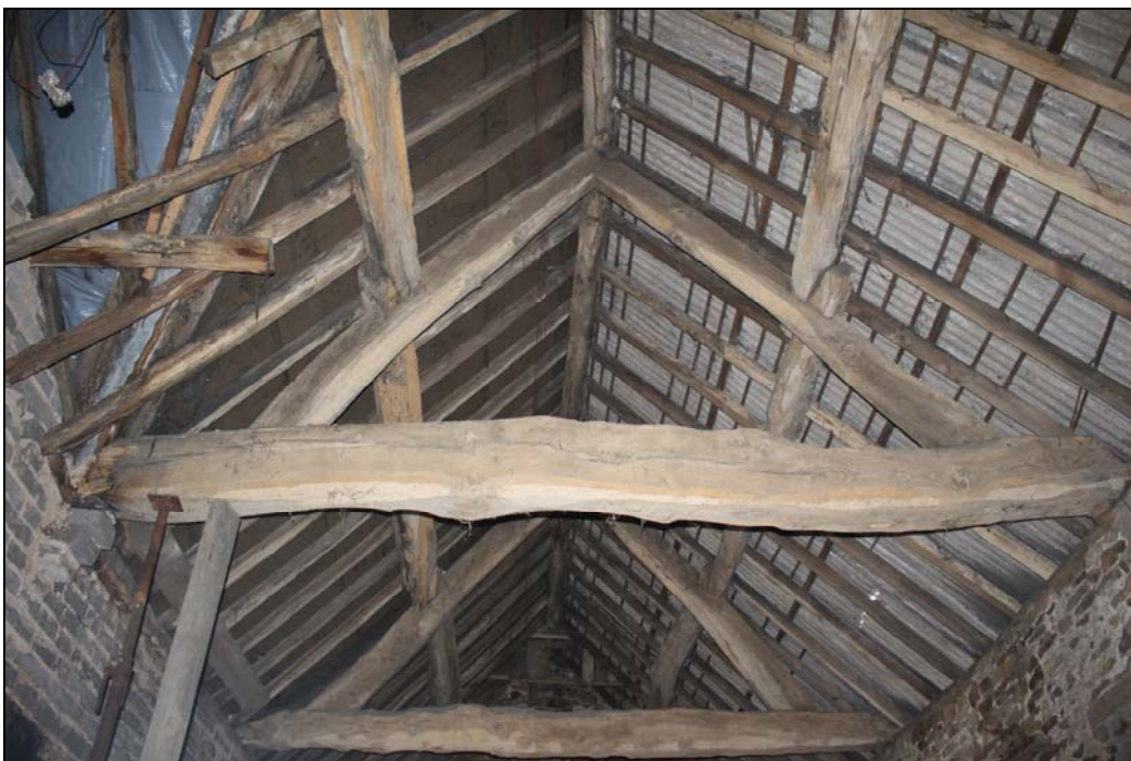
Plate 14, 46: C.1, view of the roof T3, from the north northwest
