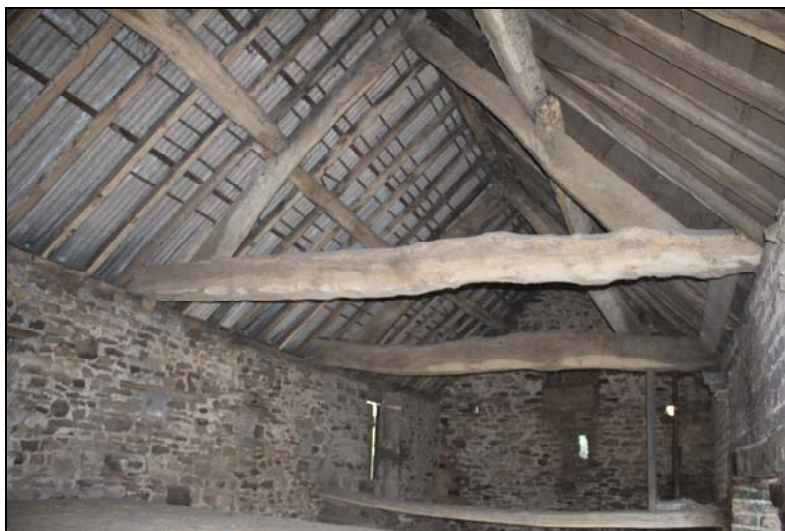
Plate 20, 113: C.3, View of the barn's roof, from the southeast
