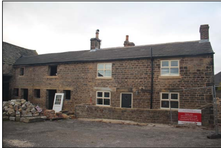
Plate 1, 2: View of the farmhouse (Bldg.A) and attached Stable with loft over (Bldg.B), from the south east
