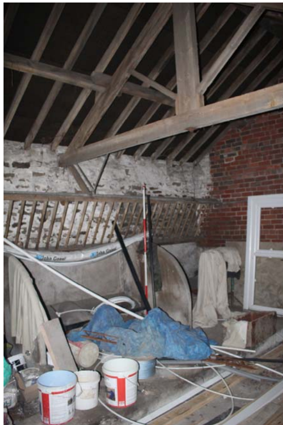
Plate 39, 108: F.3, general view of the roof, from the east
