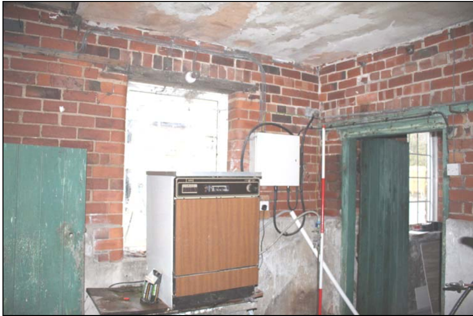
Plate 38, 100: General view, from the southwest
