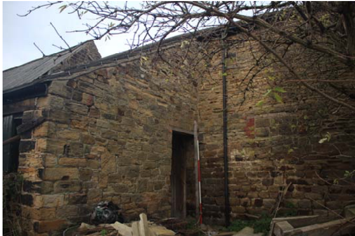
Plate 33, 32: General view, from the southwest
