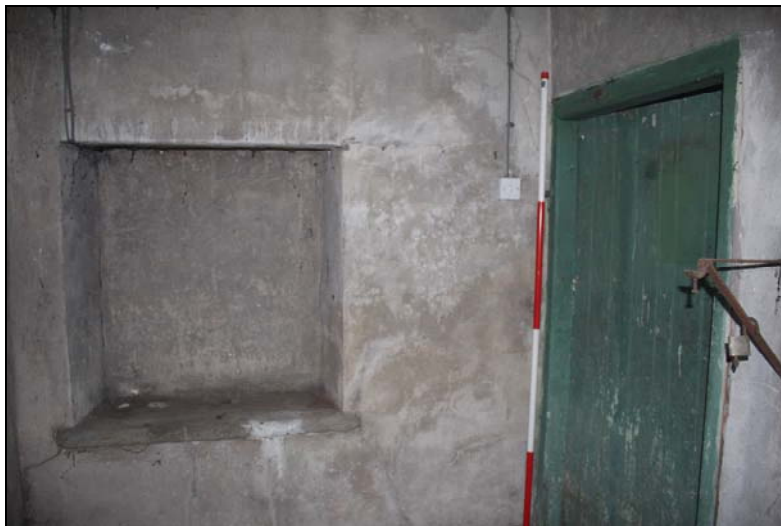
Plate 37, 99: Rm. F.1, General view, from the east
