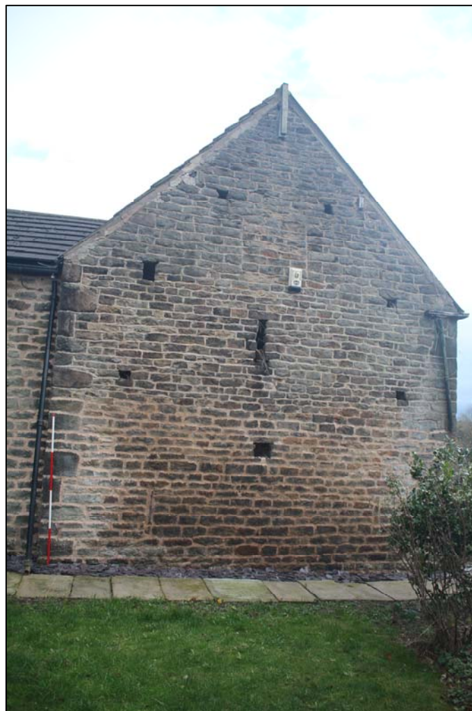
Plate 12, 89: view of the barn's gable wall, from the north.
