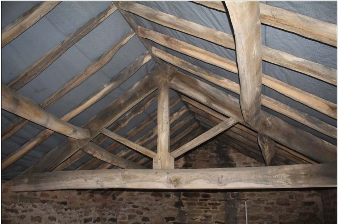
Plate 6, 11: Rm. B.2 , View of the roof truss ('III'), from the southwest
