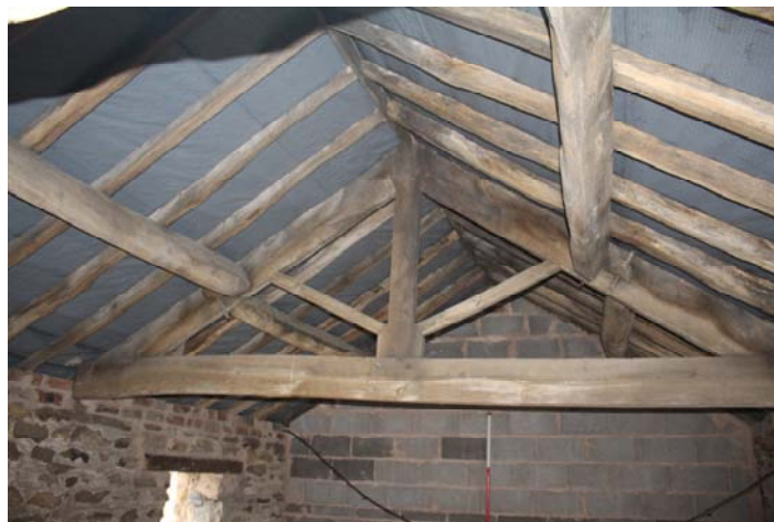
Plate 7, 16: View of the roof truss [T2] ('IIII'), from the north east
