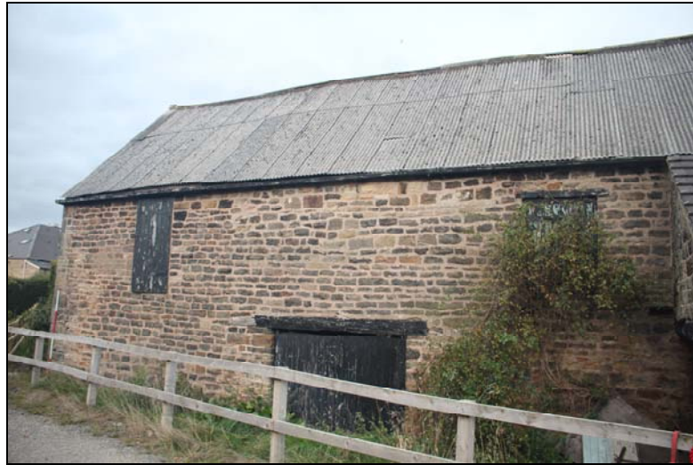
Plate 11, 88: General view of the rear elevation, from the southwest
