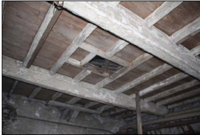
Plate 24, 114: D.1, view of the ceiling, from the east
