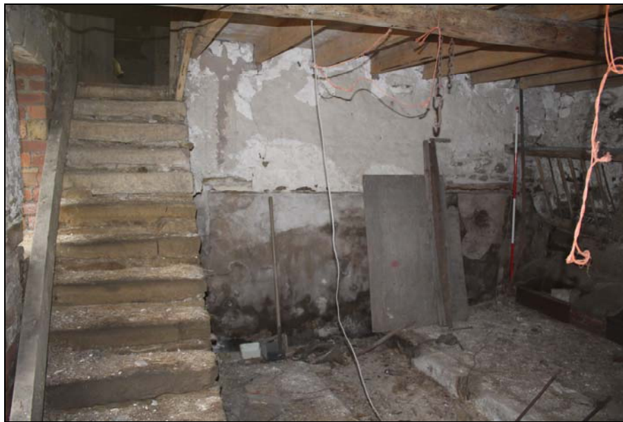
Plate 18, 51: roomC.2 , general view with inserted stone staircase, from the north northwest
