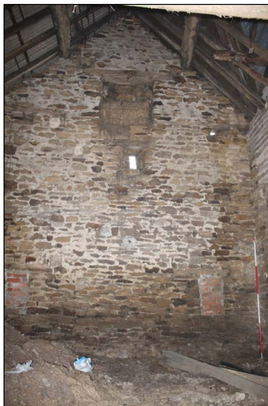
Plate 16, 41A: C.1, north gable wall (full height), from the south southeast
