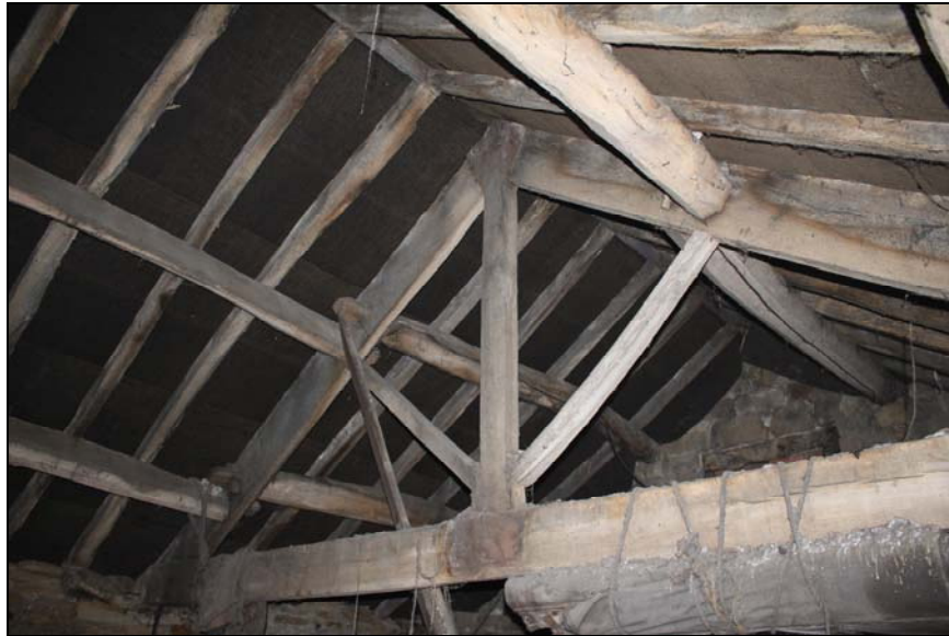
Plate 27, 69: D.3, View of the roof and truss [T5], from the southeast
