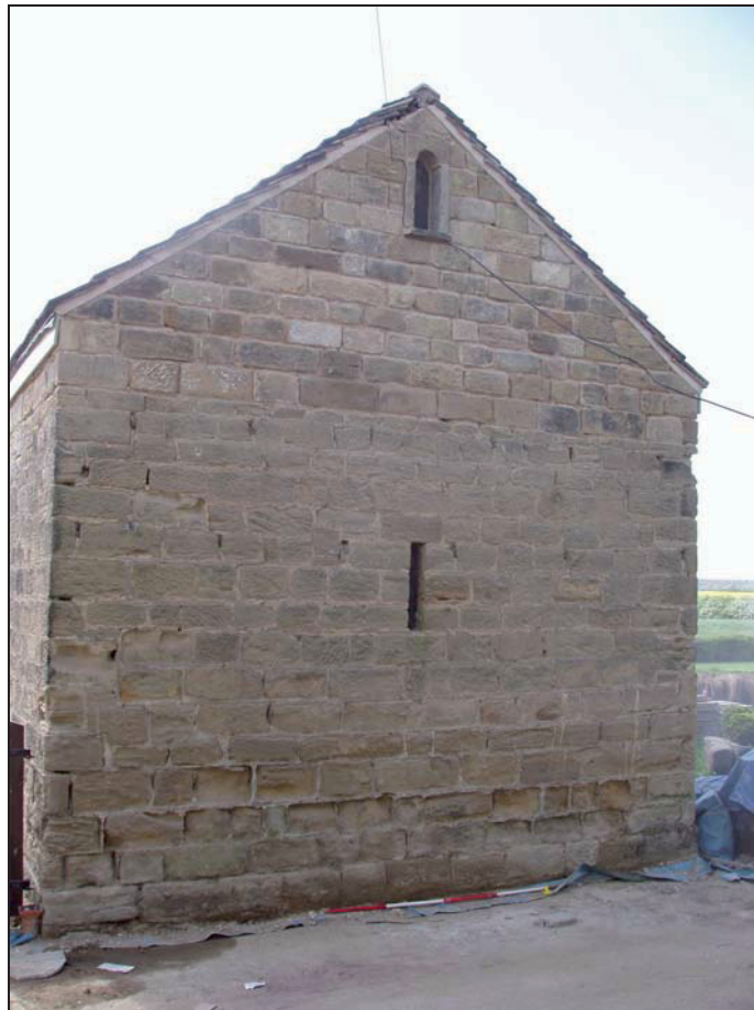
Plate 6 (3): view of the barn's north east elevation (Building A) with lower original ventilator [7] and modern repositioned ventilator above, from the north-east
