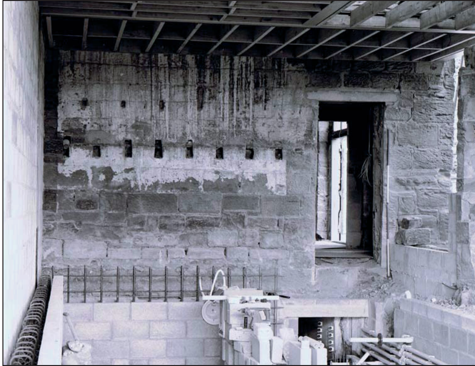
Plate 9 (14): view of the barn's lower south-west elevation (Building A) with the historically inserted floor joists [2] of Building C, from the south-west
