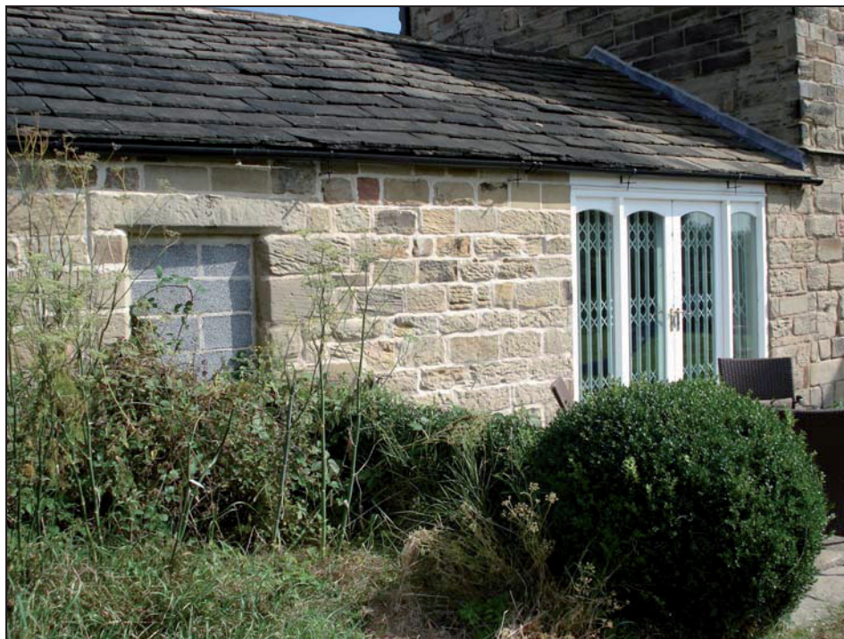
H14: Building B, external view of a repaired (narrowed) original doorway with a possibly inserted linel, from the west, c. 9/2007
