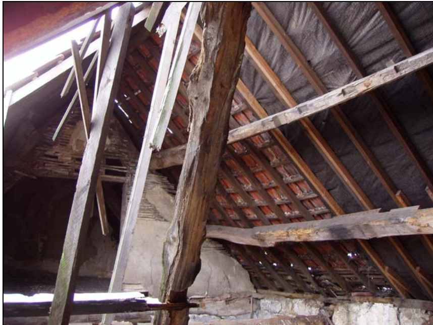
Plate 41, 79: view of the roof with fallen truss, from the southeast
