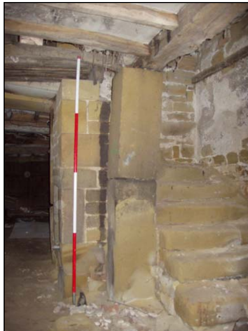
Plate 20, 59: view of the inserted quarter-turn stone staircase [11], from the north
