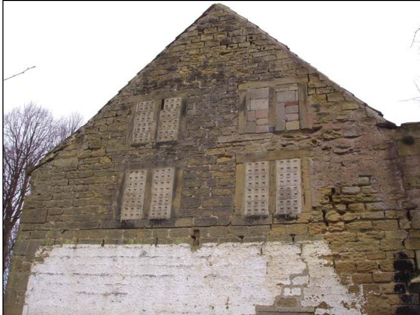
Plate 9, 14: view of the South Elevation with blocked mullion windows [4] to the first and second floor level, from the south southeast
