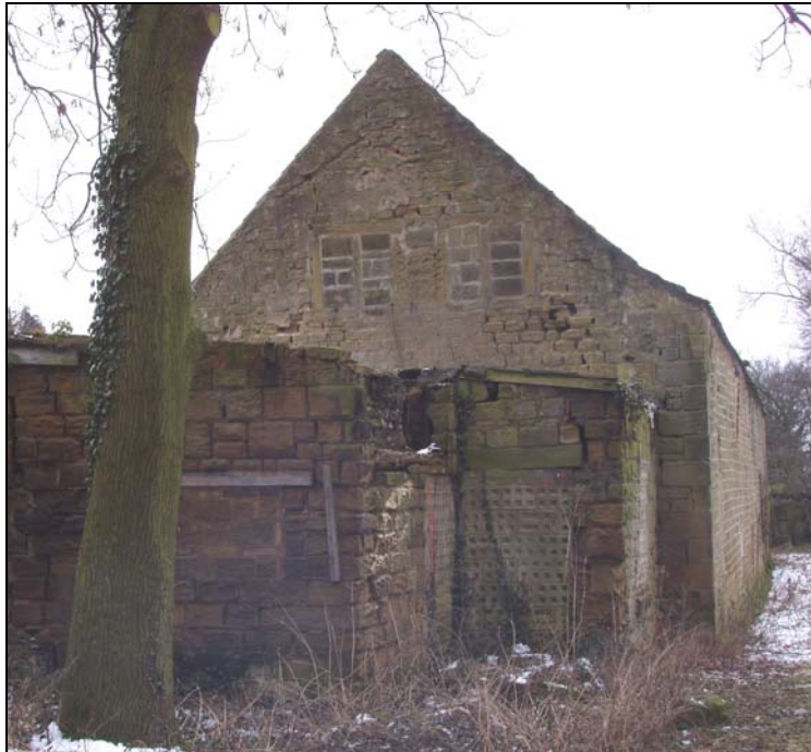
Plate 3, 5: view towards the North Elevation with the later appended buildings, showing the blocked upper mullions [1], from the north
