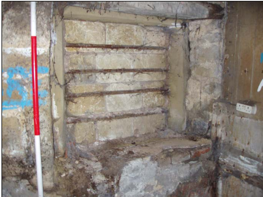
Plate 16, 82: detail of original windows with horizontal bars, from the southeast
