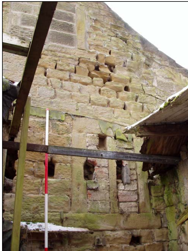
Plate 4, 20: detail of one of the two lower blocked mullion windows [1], from the northeast
