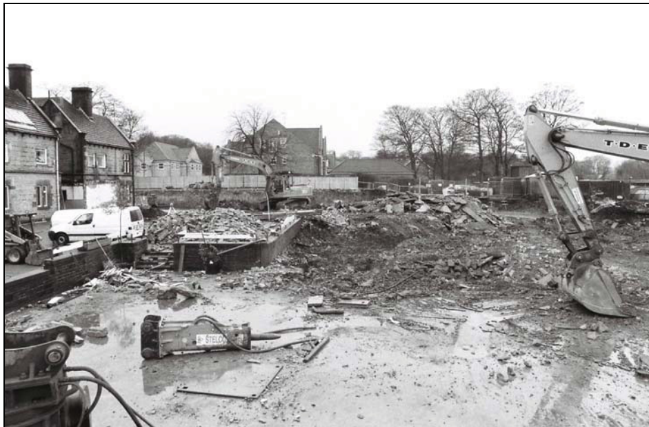
Plate 20: Post-demolition view, from the east
