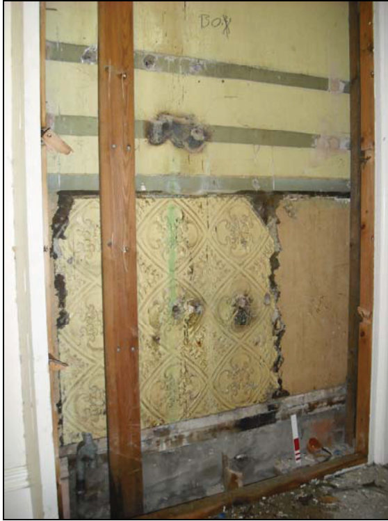
Plate 23: Detail of the room's original decoration (heavily embossed wall paper) in the former bedroom 'Kitchen' (Room 1/12), from the west
