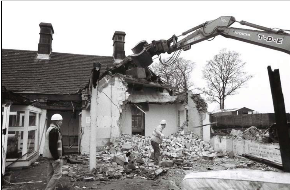
Plate 15: Working view, from the east
