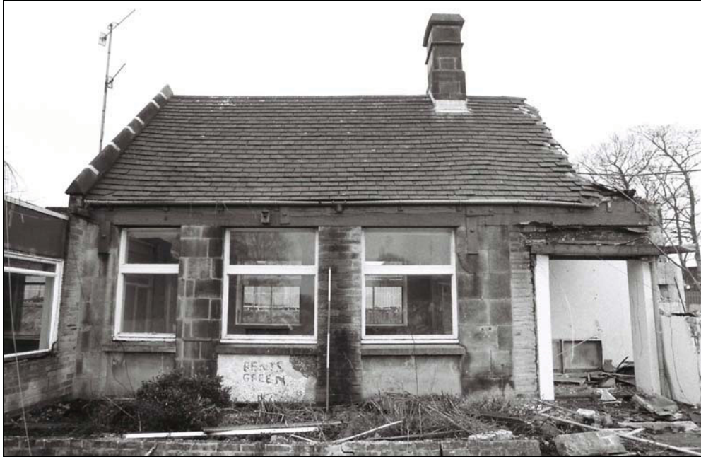
Plate 17: View of the blocked 'cartdoor' [9] with doorway [10] to the left hand side, from the east
