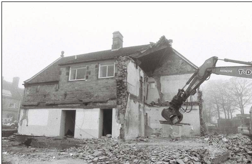
Plate 6: Building 3, general view, from the northeast
