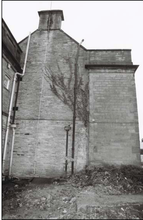
Plate 25: The western gable of the phase 1 building, from the west
