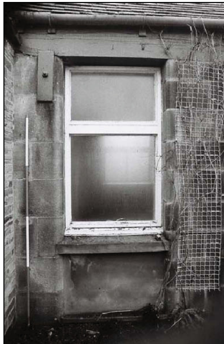
Plate 18: View of the blocked doorway [10], from the east
