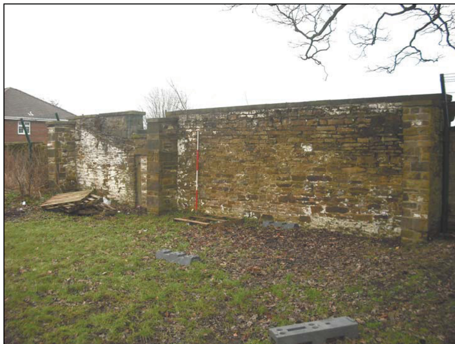
Plate 28: The North Elevation of the walled garden's north wall with lean to roof line and lime wash still adhering, from the northwest
