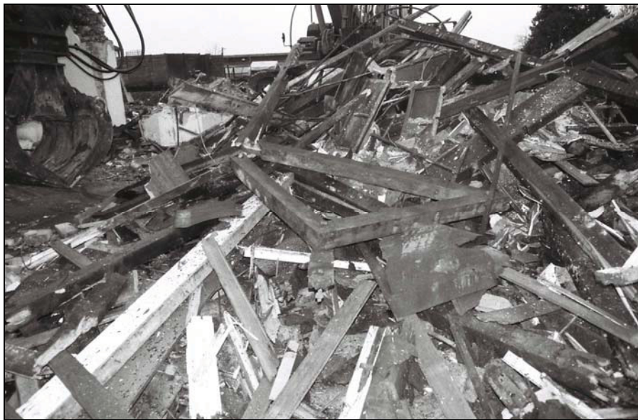
Plate 14: Demolished roof with a collared roof truss [12], from the south
