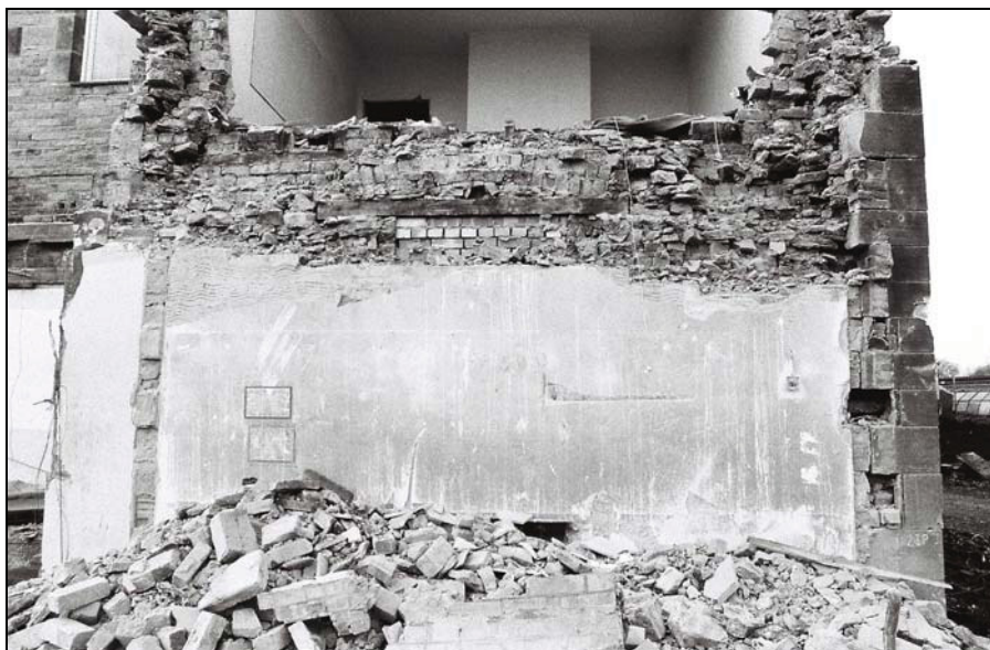
Plate 4: Building 3, detail of a blocked and obscured window [2] represented by the timber lintel and arched brickwork above to the lower East Elevation , from the east
