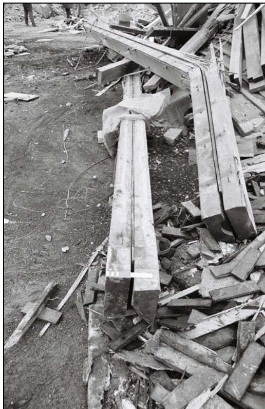
Plate 8: Building 3, view of the two extracted composite beams [4], from northeast
