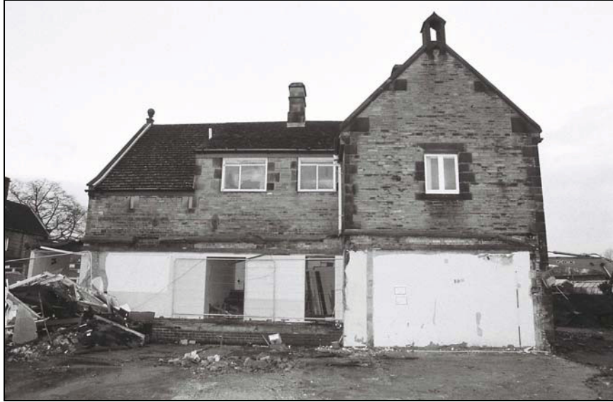
Plate 1: Building 3, general view of the East Elevation , from the east
