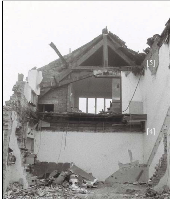
Plate 7: View of the in situ roof truss [5] and the northern transverse first floor beam [4]
