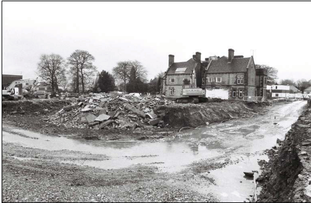
Plate 21: Post-demolition view, from the northwest
