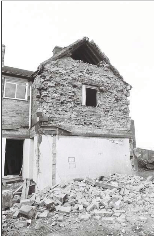
Plate 3: Building 3, view of the partially demolished East Elevation , from the southeast
