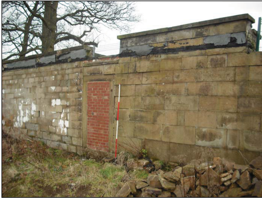
Plate 27: Oblique view of the south ashlar elevation, from the east southeast
