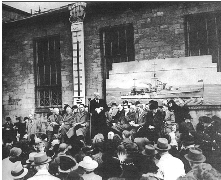
Plate 12: view of the northwest elevation in 1942 during the fund raising for H.M.S. Wallflower , from the west
