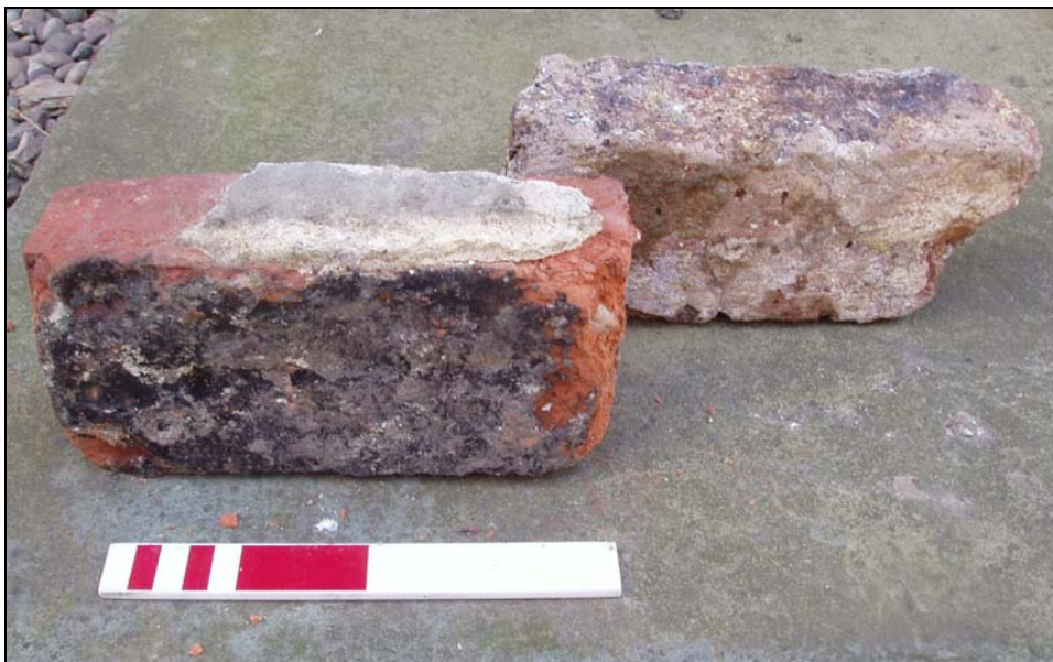
Plate 8, 98: detail of bricks used in the duct [108] with lime mortar and soot still adhering
