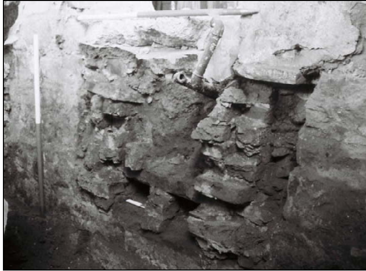
Plate 11, 31: trench 20b, oblique view of the brick duct [108a] below Doorway B, from the west
