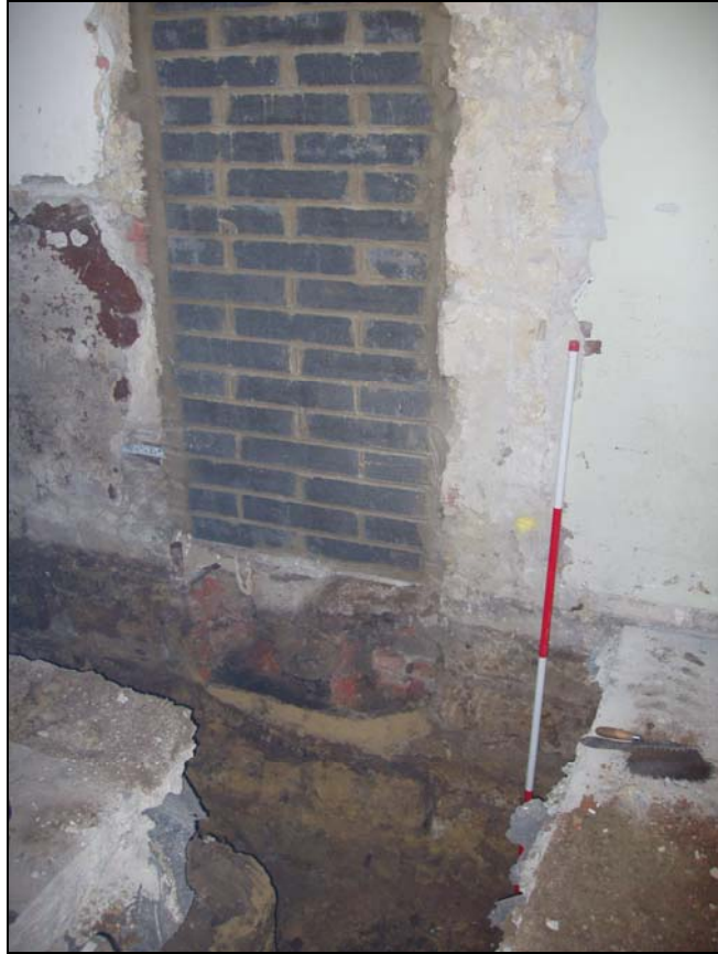
Plate 5, 37: trench 1b, Doorway A with the brick duct [108], from the northwest
