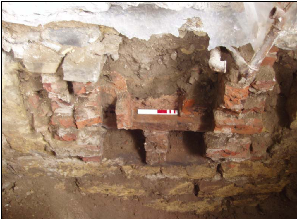
Plate 10, 32: trench 20b, detail of the brick duct [108a] below doorway B, from the northwest
