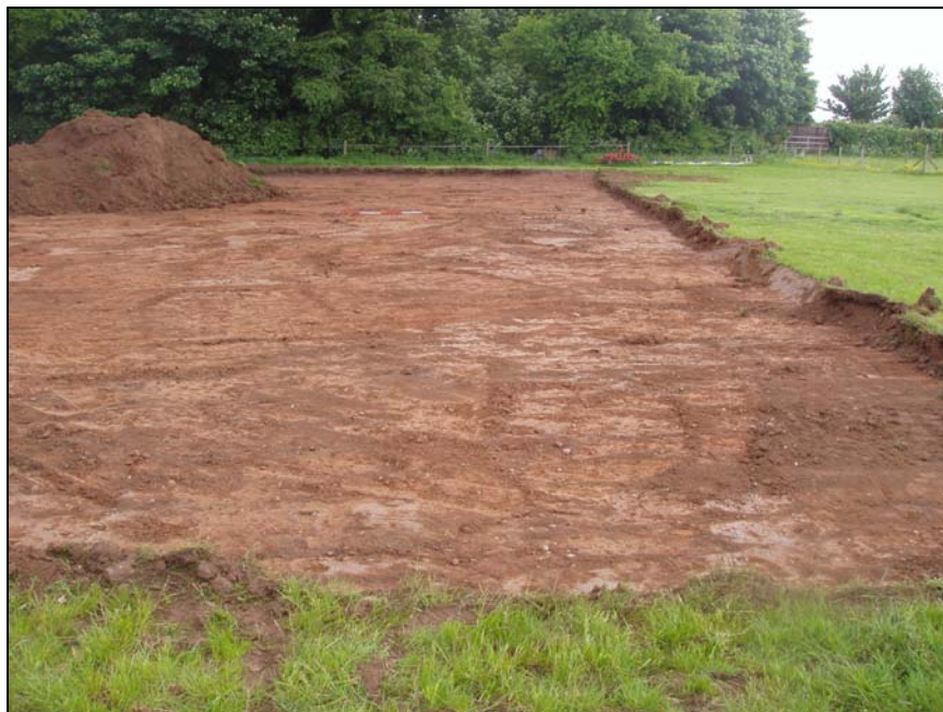
Plate 8: the excavated south-western half of the PDA, from the northwest
