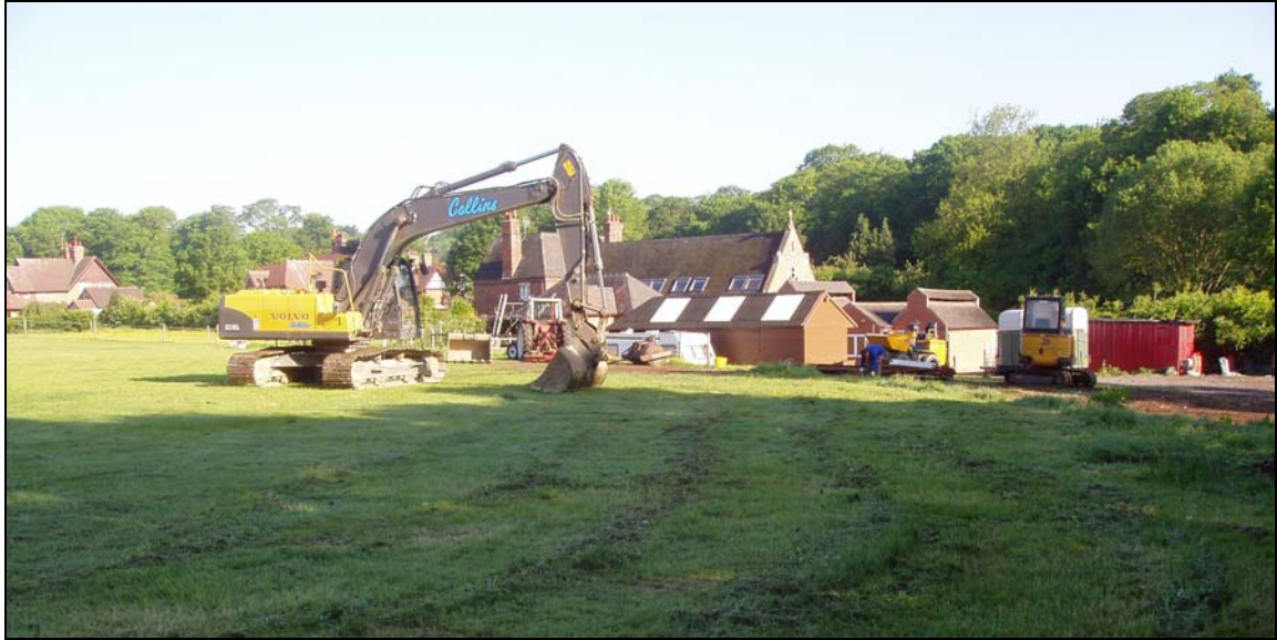
Plate 1: Pre-excitation view of the PDA, from the southeast
