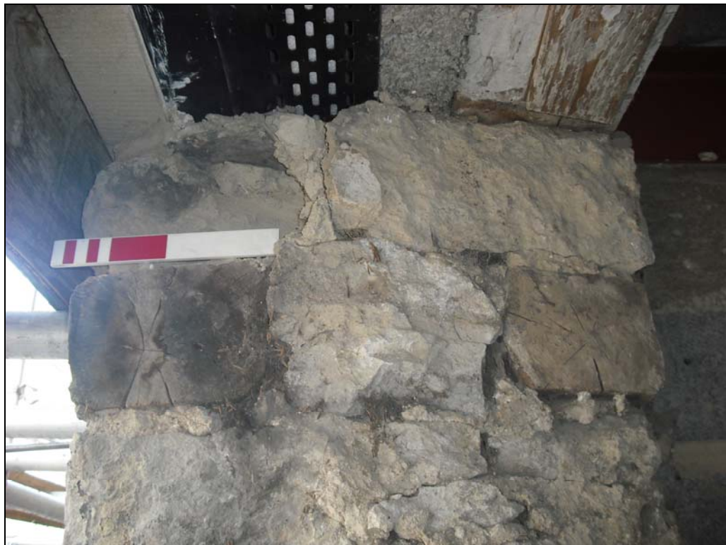
Plate 10, 65: detail of the truncated oak beams [4], from the southwest
