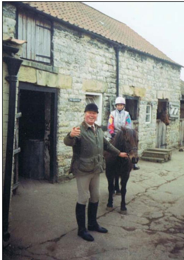
PLATE 4 view of building A, with Mr Anthony Barker, c. 1970
