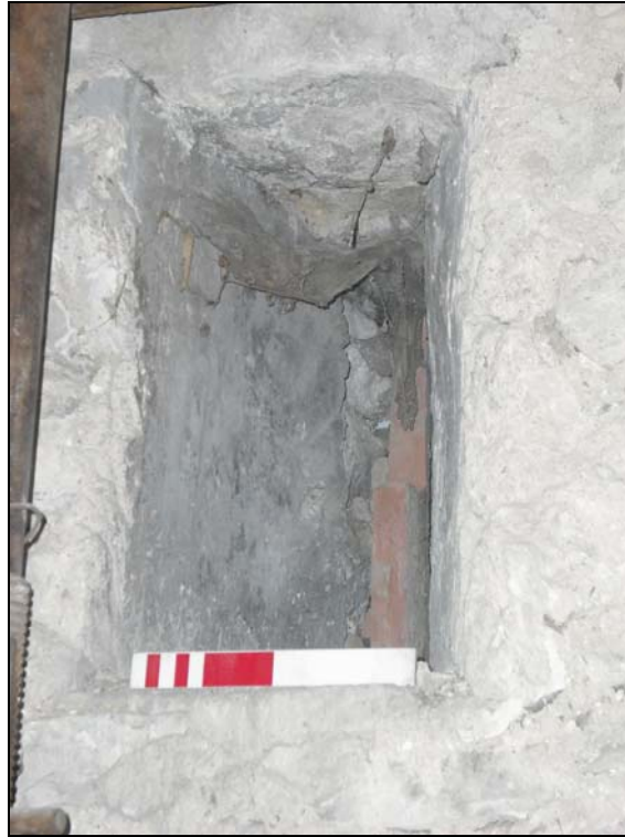
Plate 11, 20: detail of the partially extant slit ventilator [1], from the northwest
