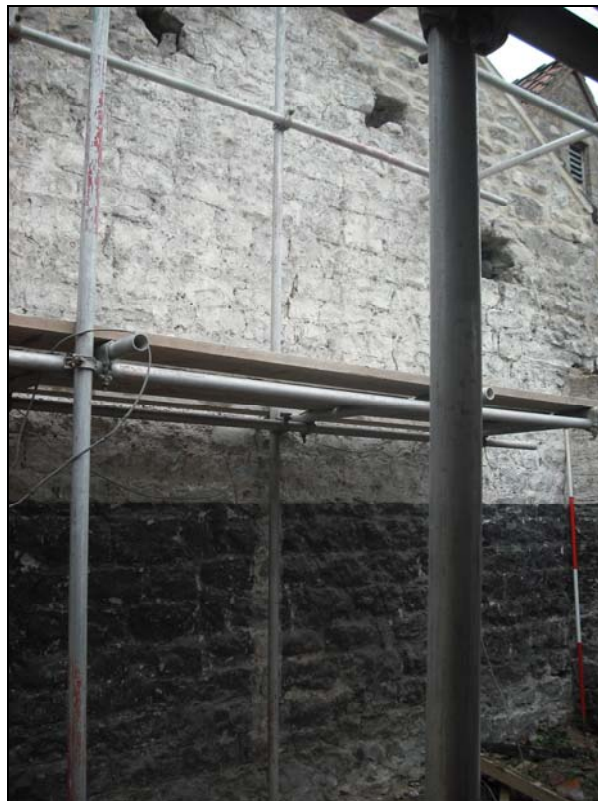
Plate 12, 12: view of the southwest wall with purlins removed, from the west
