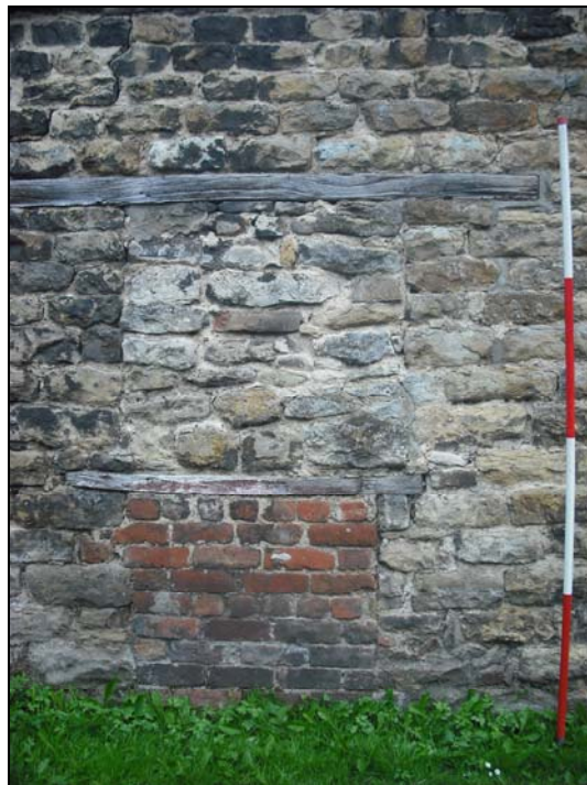
Plate 27, 75: detail of the blocked door (internal location: Bldg. B, Rm. 10)
