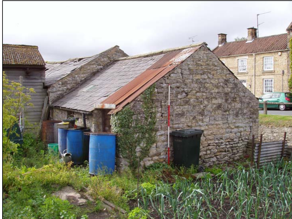
Plate 19, 79: view of building B's northern end ( Northwest Elevation ), from the north
