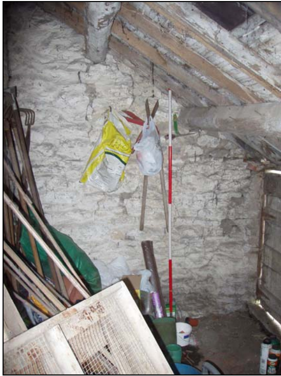
Plate 26, 81: building B, Room 11, general view from the southeast
