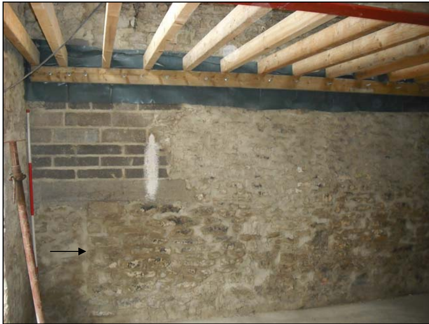
Plate 9, 27: view of the northeast wall (ground floor level) with vertical building below the modern rebuilt wall, from the southwest
