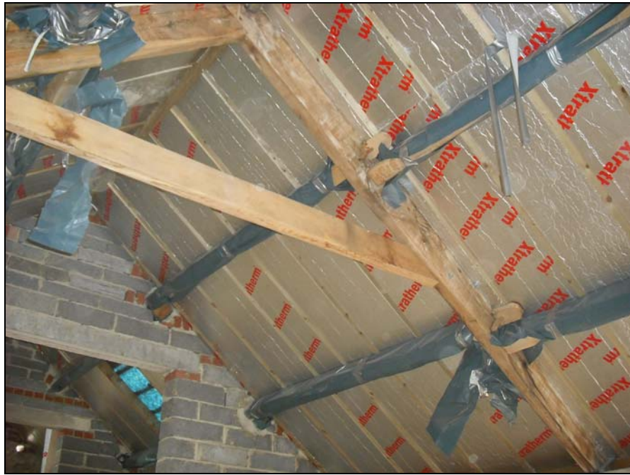
Plate 13, 36: view of the repaired and modified roof truss, from the east
