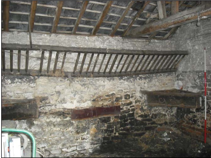
Plate 25, 50: building B, room 8, view of the southwest wall, from the northeast
