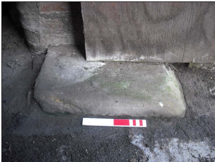
Plate 25a, 66: building B, room 7, detail of the stone post pad, from the southeast
