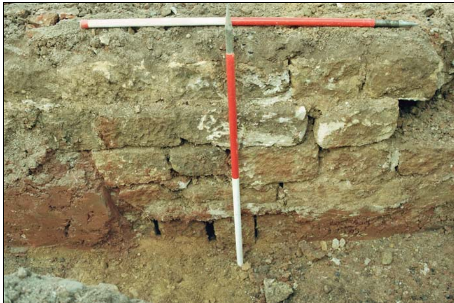
Plate 6: Detail of wall D's, 'external' east facing elevation, from the northwest
