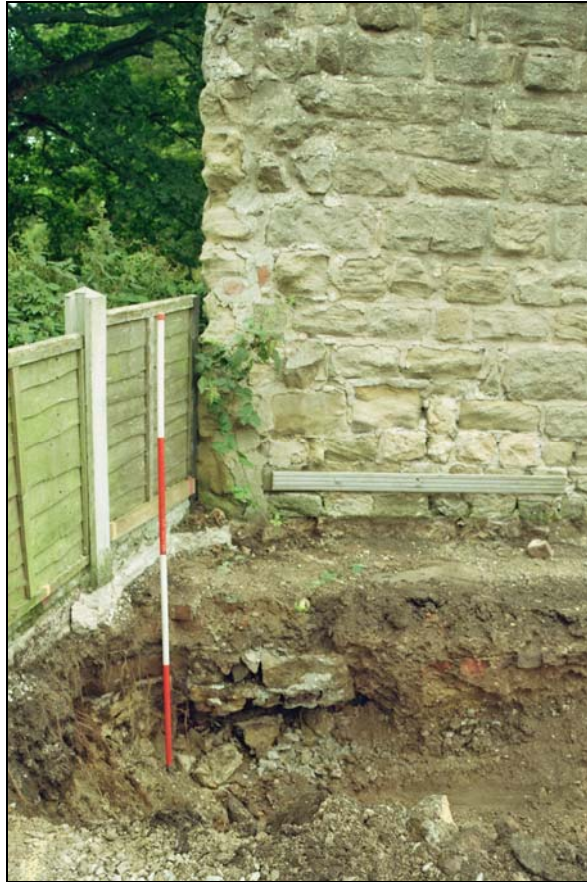
Plate 5: View of the end of the extant butressed wall with the vertical scar of the return (southern) wall with in situ footings, from the east southeast
