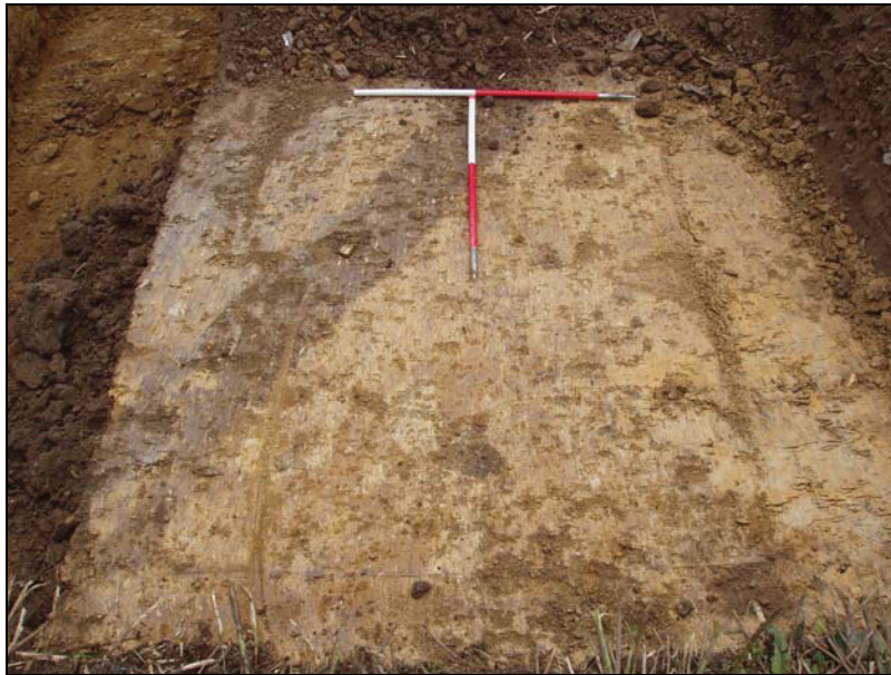
Plate 2: view of the sub station trench with modern land drain, looking south
