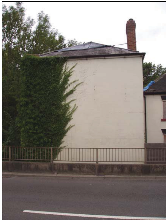
Plate 2: the rendered and obscured gable wall (Building A1), from the southeast
