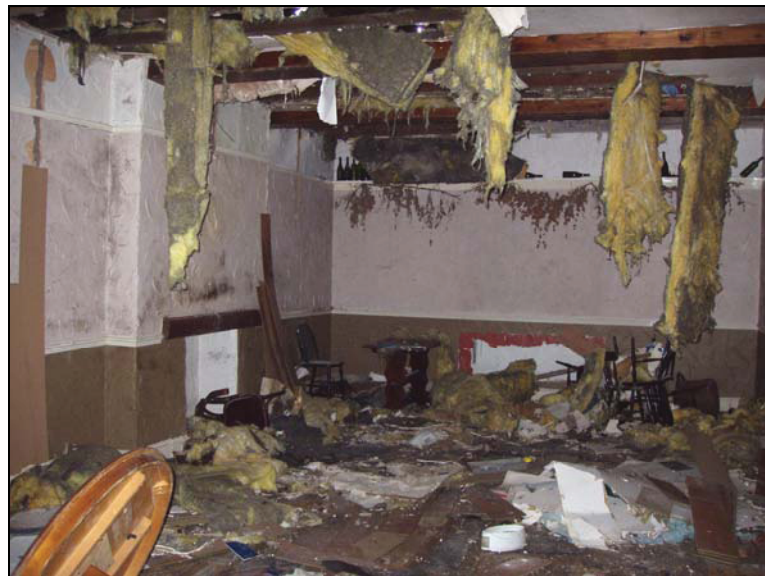
Plate 6: Principal first floor bedroom, from the west
