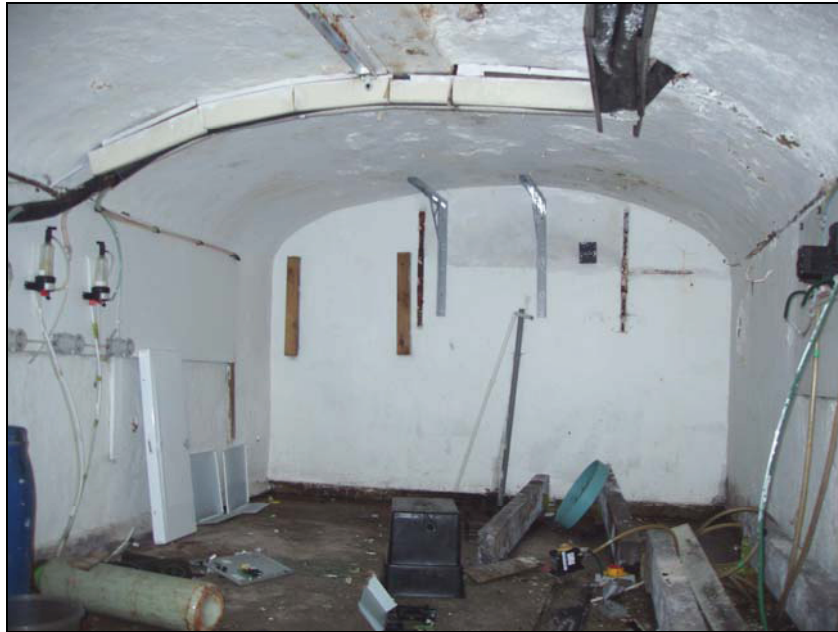
Plate 9: The vaulted cellar (Building A2), from the southwest
