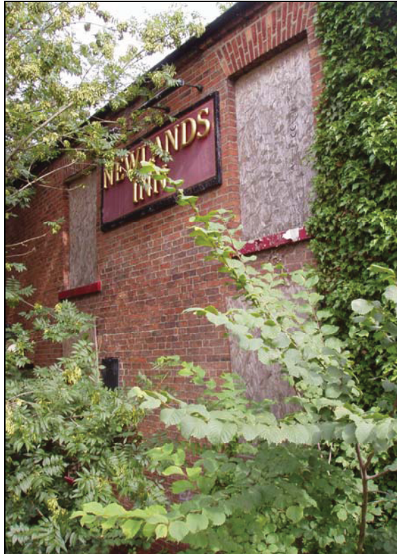
Plate 1: the front southwest elevation (Building A1), from the south southeast
