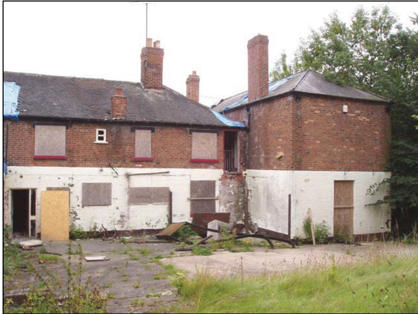
Plate 13: the rear northwest elevation (Building A1/A2), from the north
