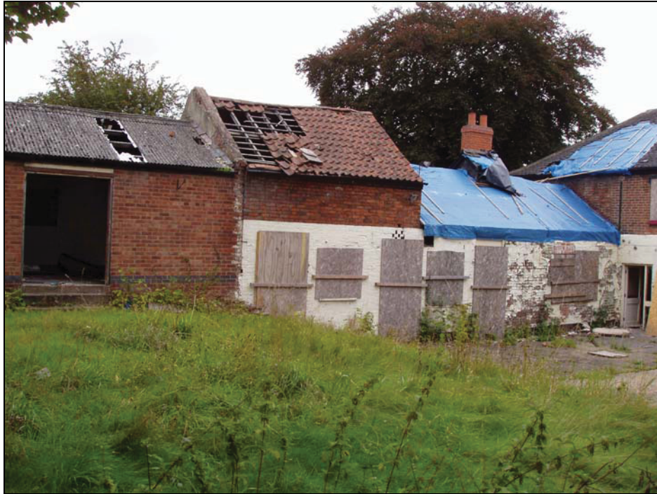
Plate 21: the front southwest elevation (Building A3), from the west
