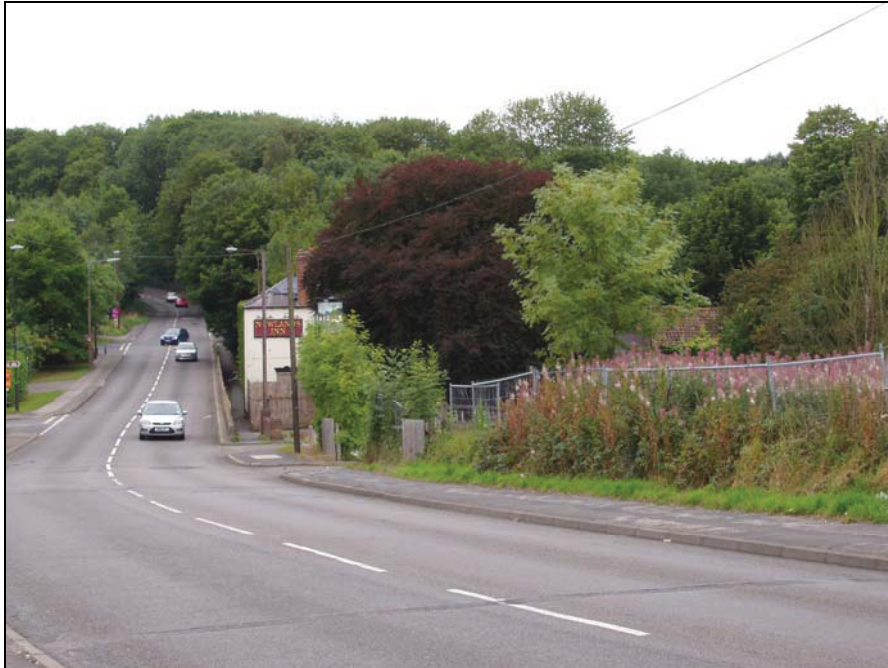
Plate 25: Newlands Inn from the northeast
