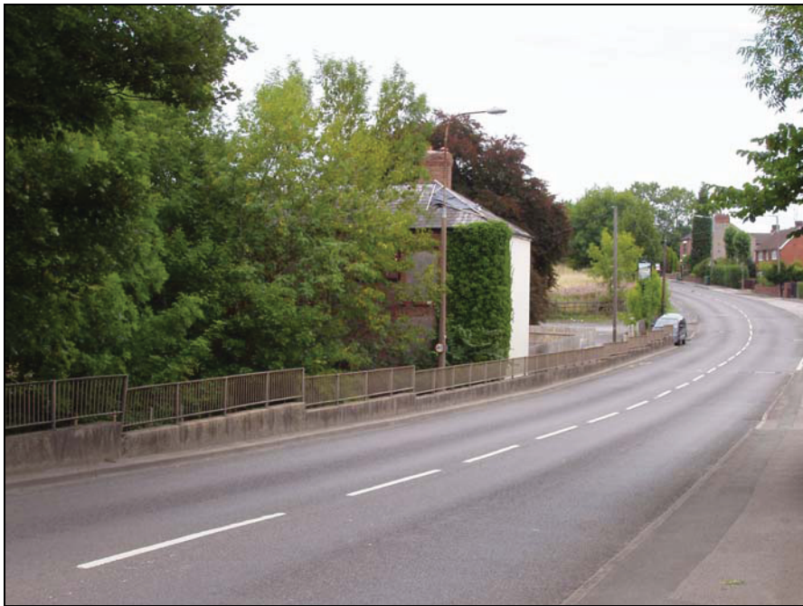
Plate 24: view of Newlands Inn behind the raised road, concrete walls and historically unsympathetic railings, from the south southeast
