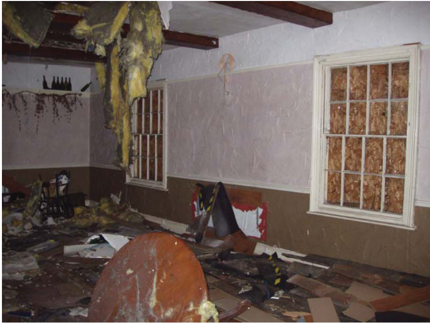
Plate 5: Principal ground floor bar recently the 'family room', from the north
