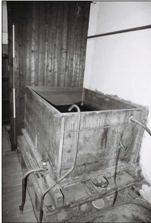
**Plate 43, 70:** room 1/2/31, view of the slate header tank, from the southwest
