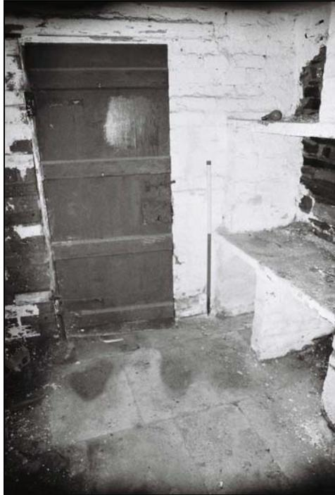
**Plate 23, 4:** Room 1/-1/2, view of the Wine Cellar door with plank and battened with internal lock, from the south southeast
