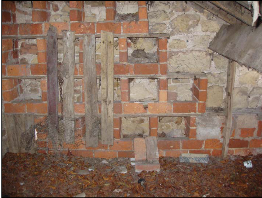
Plate 37, 234: view of the brick hen boxes, from the north
