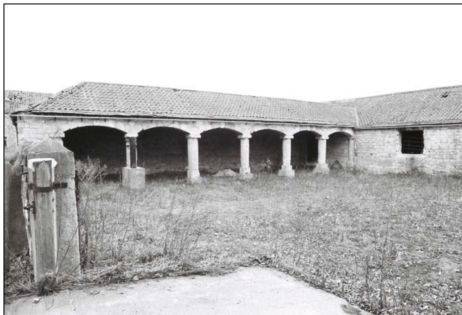
Plate 44, 30: view of the shelter shed's south elevation, from the southwest
