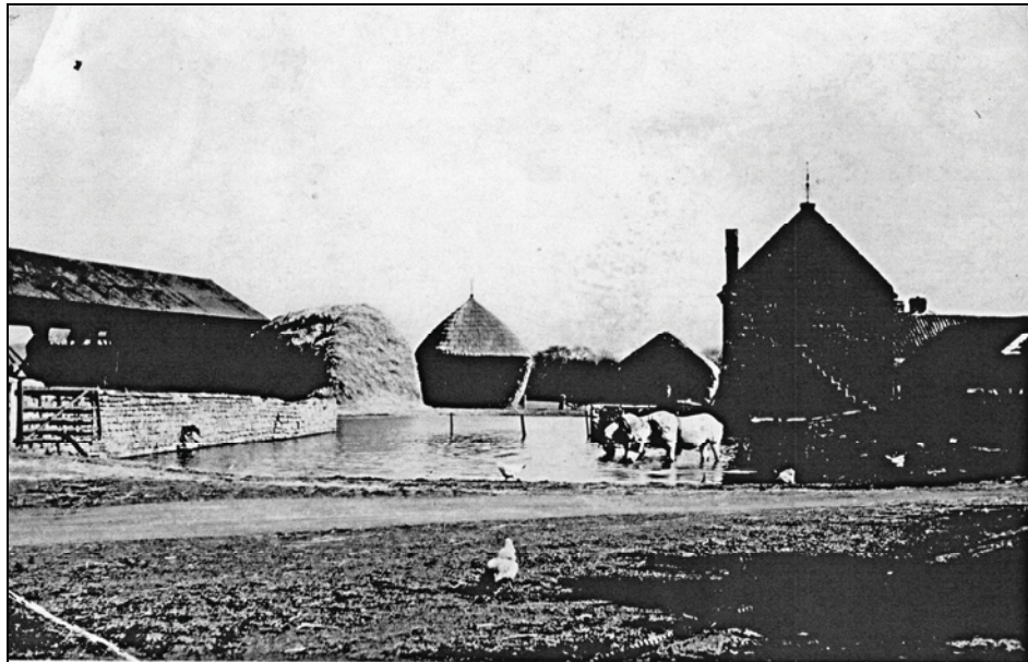
Plate 5 (historic photograph), view of the former pond north of Building 1, from the west
