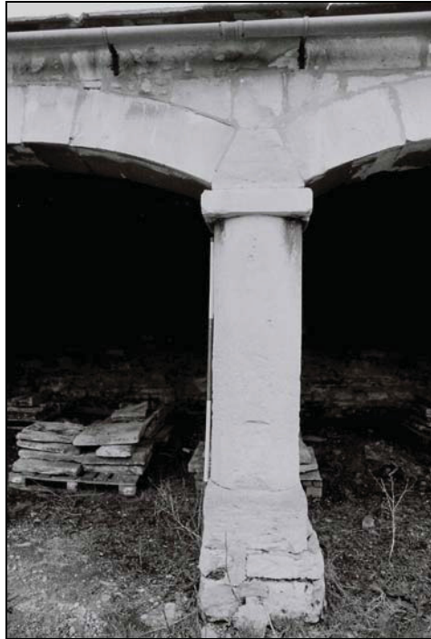
Plate 41, 20: view of the front, east elevation of the eastern extension, from the east
