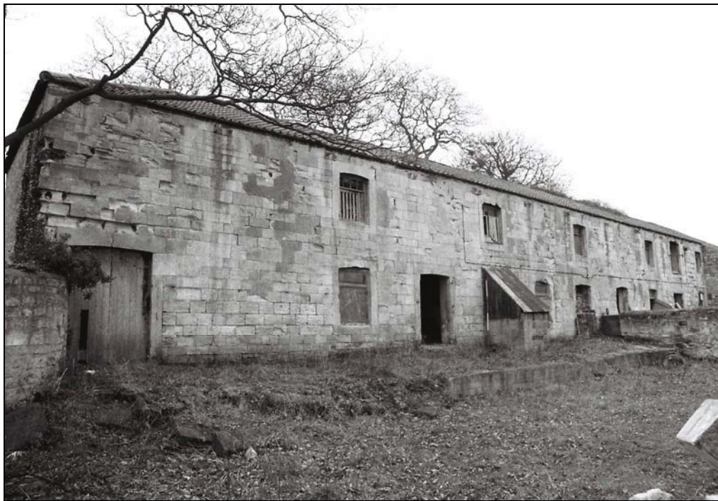
Plate 20, 38: oblique view of the east elevation, from the southeast
