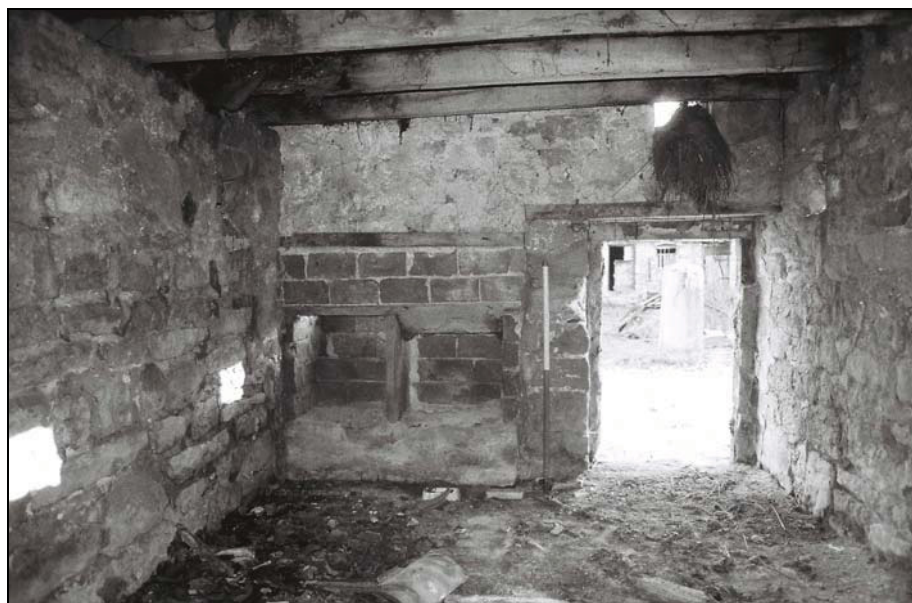
Plate 30, 210: general view, from the west
