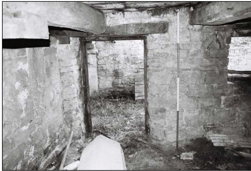
Plate 11, 146: general view with the beam notched onto the oak lintel, from the north
