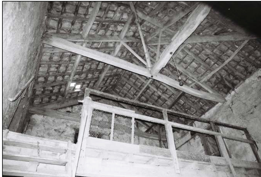
Plate 36, 81: general view of the hipped roof, from the north northeast
