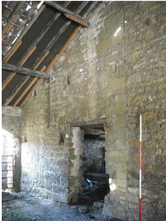
Plate 14, 11: general view of the inserted doorway, from the southeast
