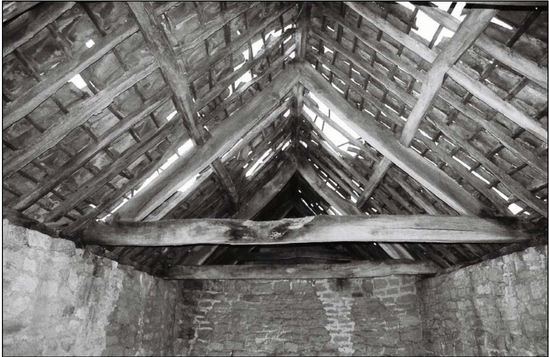
Plate 19, 174: general view of the roof, from the east
