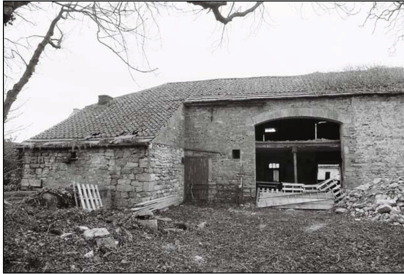
Plate 23, 48: view of the barn doorway and western extension, from the southwest
