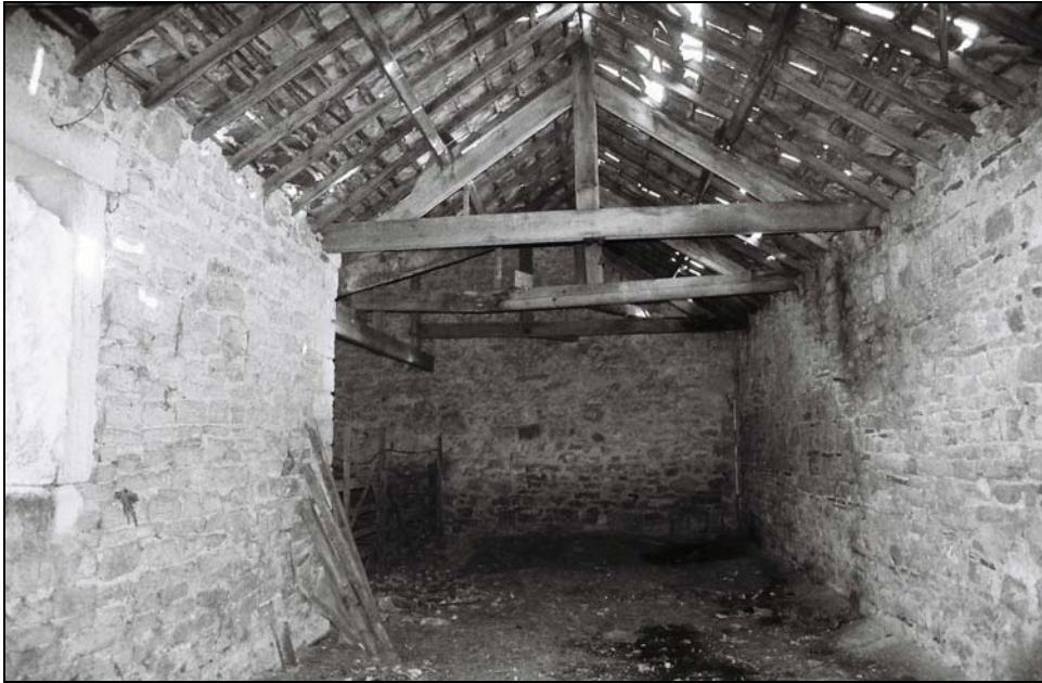
Plate 45, 199: general view of the roof with type 5 trusses, from the west
