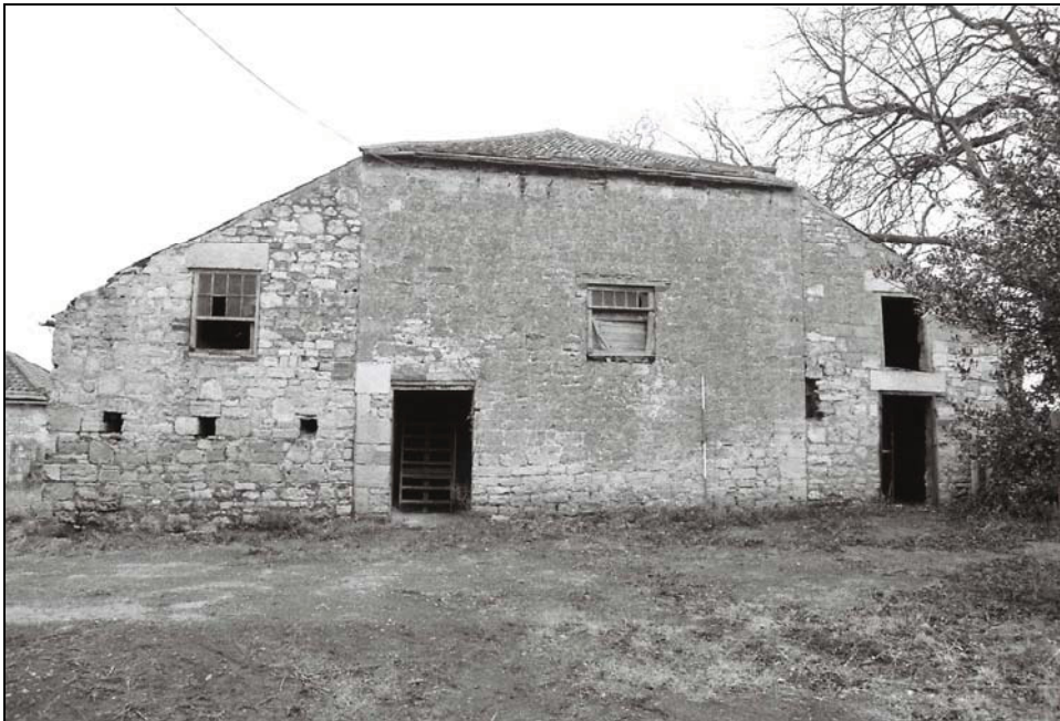
Plate 22, 46: view of the north elevation with the two appended extensions, from the north
