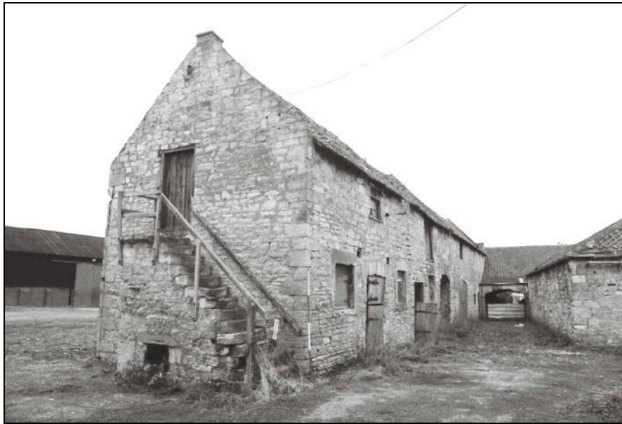
Plate 1, 7: oblique view of the west and south elevations, from the southwest
