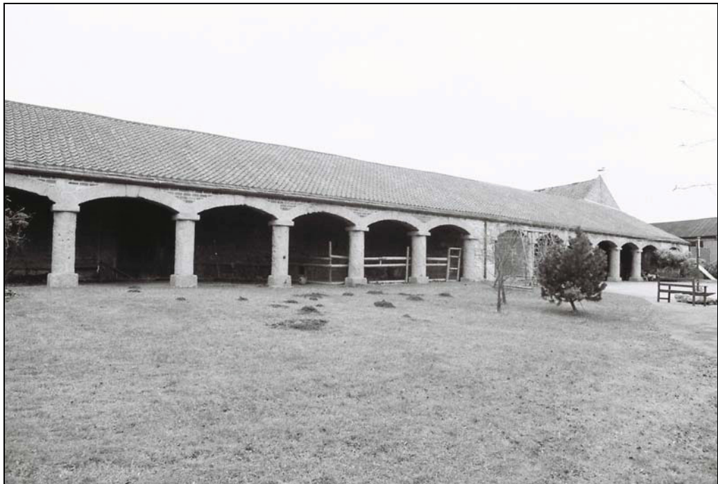
Plate 48 , 13: view of the shelter sheds, from the southeast
