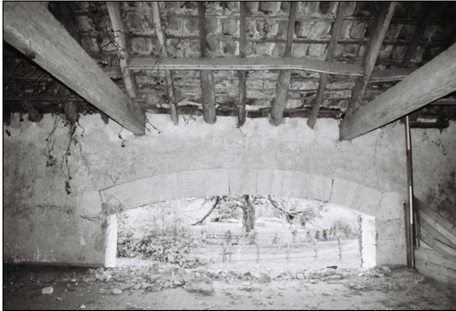
Plate 33, 98: general view of the east wall with the top of the exposed barn door and inserted floor, from the east
