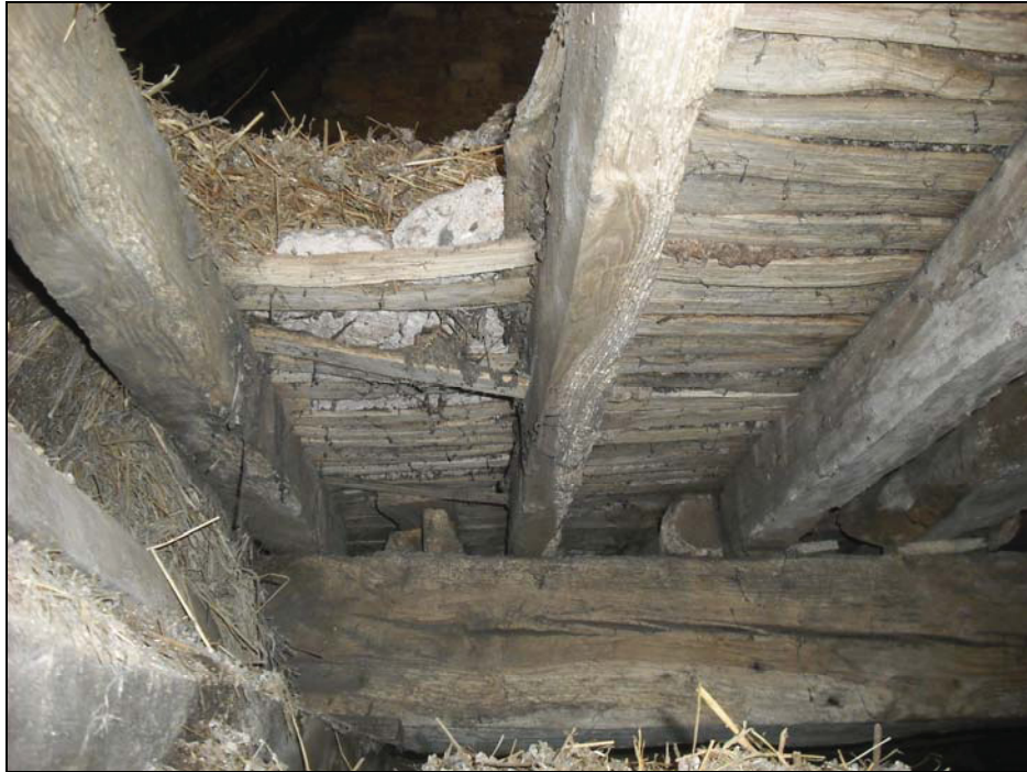
Plate 13, 231: detail of the limecrete ceiling, from the west
