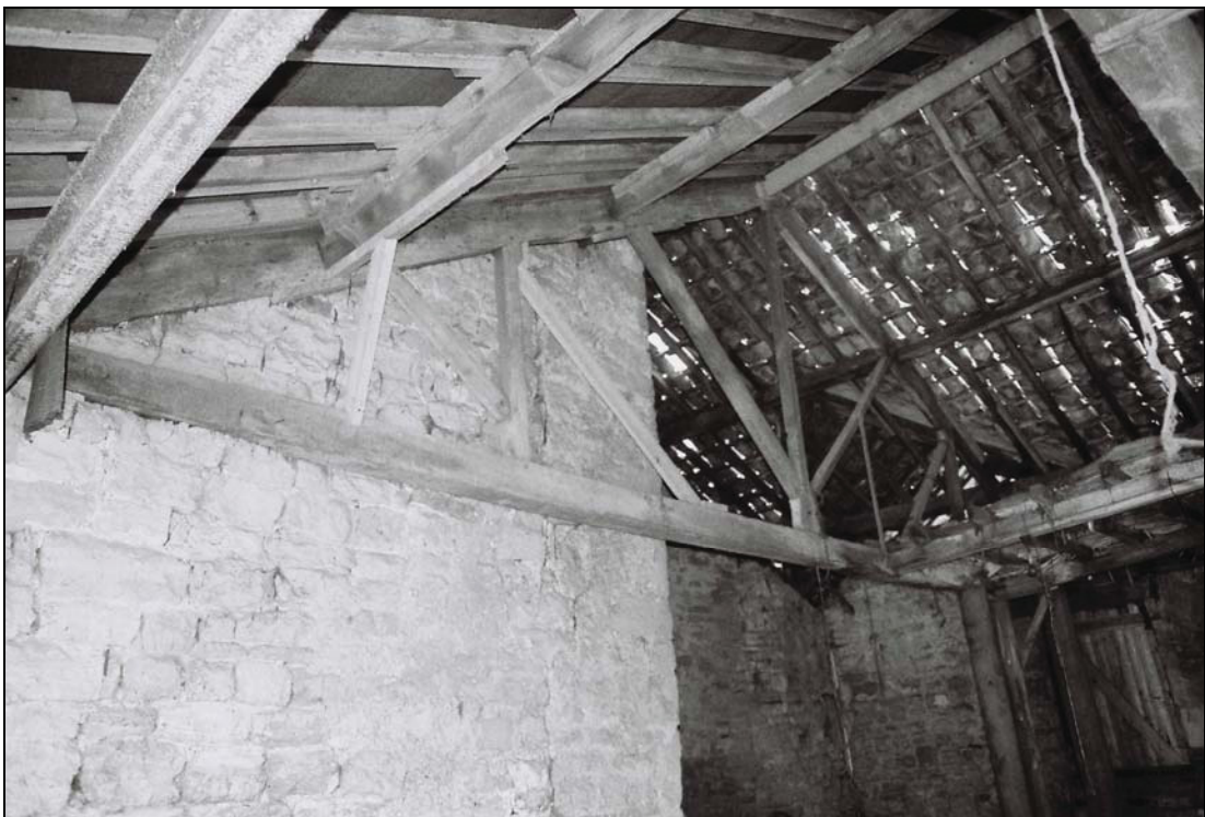
Plate 38, 225: view of the roof truss, from the northeast
