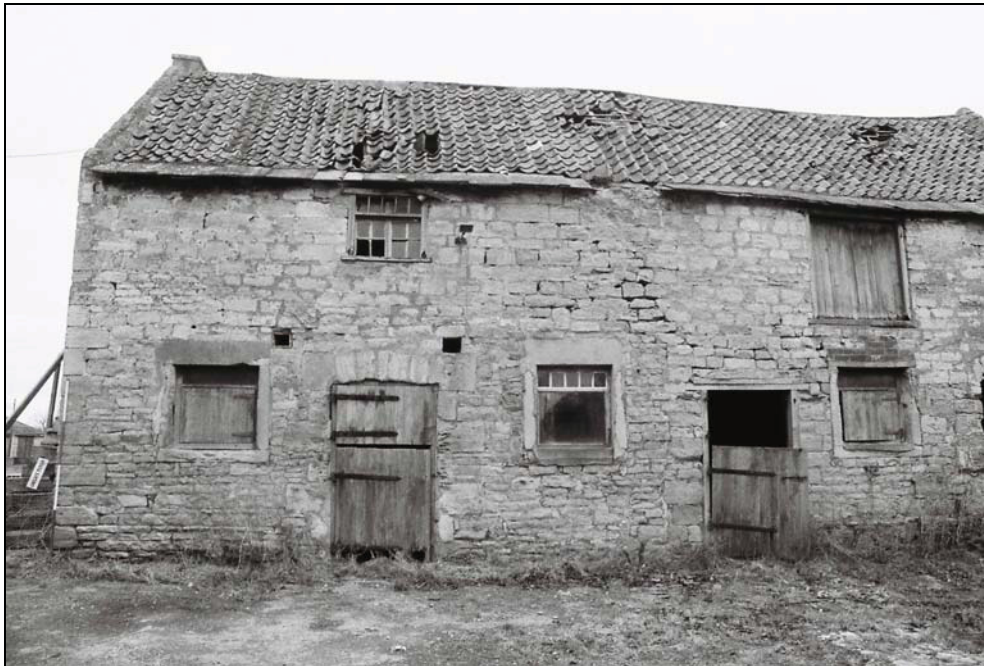
Plate 2, 8: western end of the south elevation, from the south
