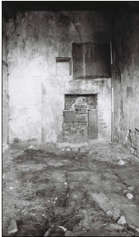
Plate 7, 125: general view towards the fireplace in the north, from the south
