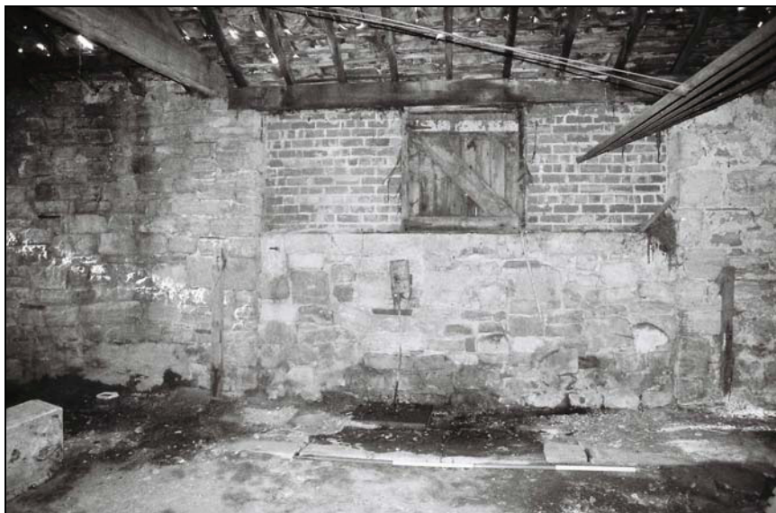
Plate 39, 196: view of the blocked barn doorway, from the east
