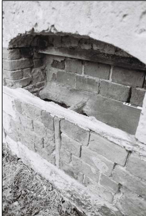
Plate 31, 45: detail of the trough, from the northeast
