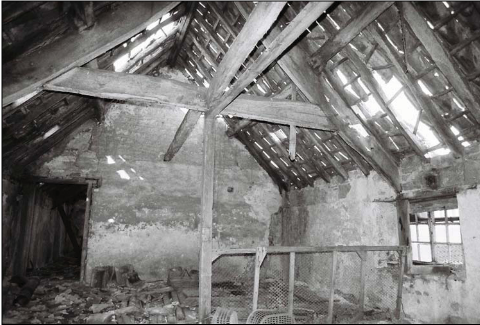
Plate 15, 152: general view of the type 3 truss, from the west
