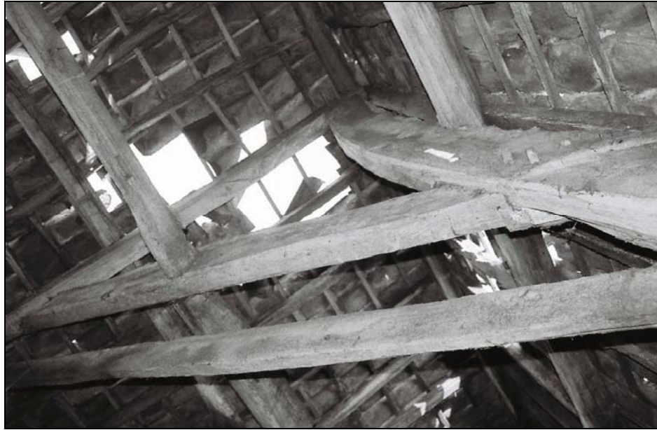
Plate 17, 157: General view of the type 3 truss, from the southeast
