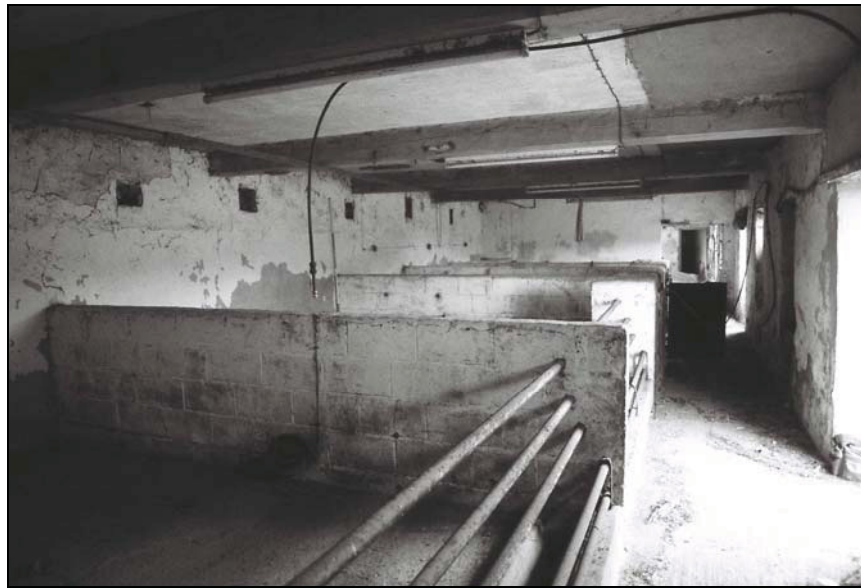
Plate 27, 63: general view, from the west
