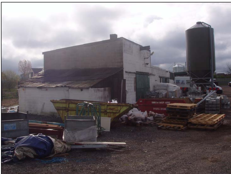
Plate 1: general view of the extant former slaughter house, from the northwest
