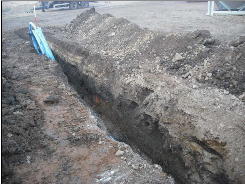
Plate 1, 43: trench 2, general view, from the southeast
