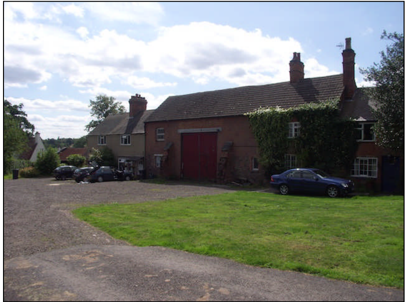
Plate 1: East facing elevation with farmhouse to the right of the threshing barn and cottages to the left
