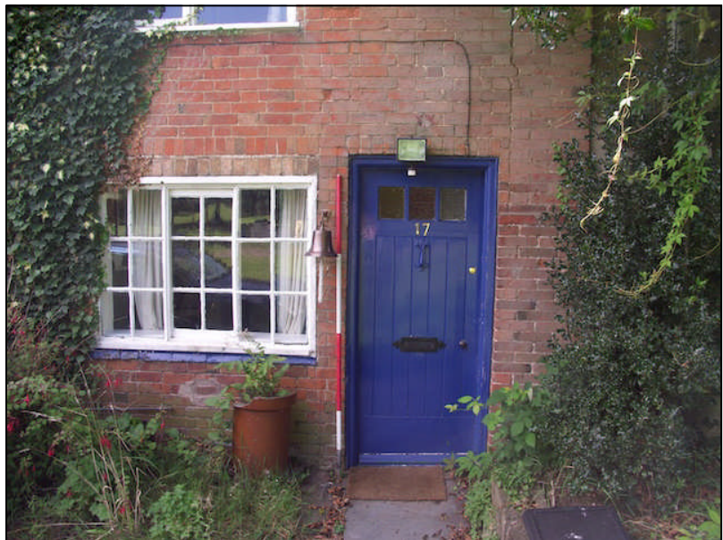
Plate 5: Surviving vertical sliding sash windows and timber ledged and braced front door
