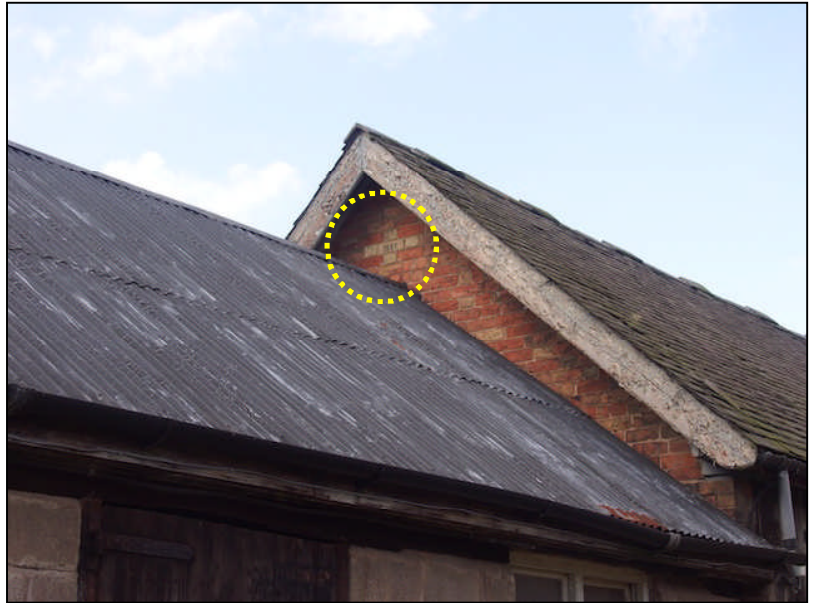
Plate 10: 1881 date marked in the brickwork in the apex of the gable
