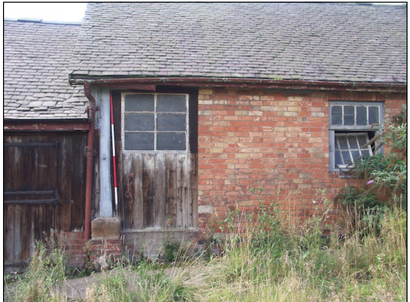
Plate 11: Original timber posts on stone plinths to cow sheds
