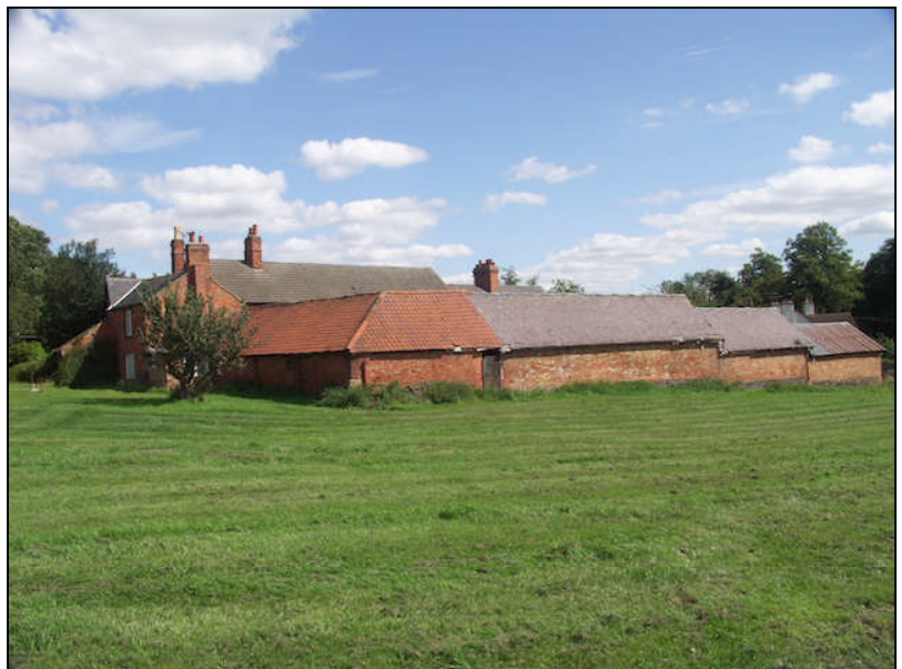
Plate 8: West facing elevation of the stock shed range
