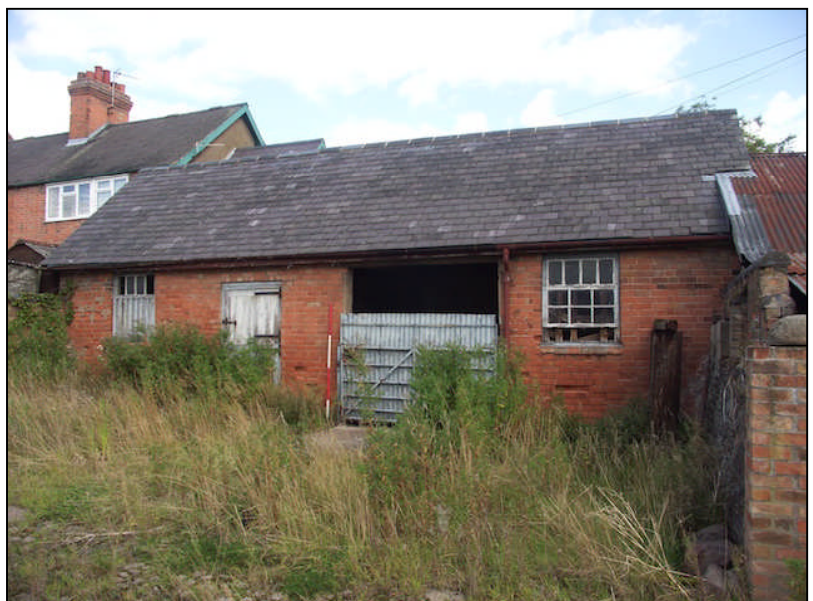
Plate 12: Front elevation of stable block with 'hit and miss' ventilator windows
