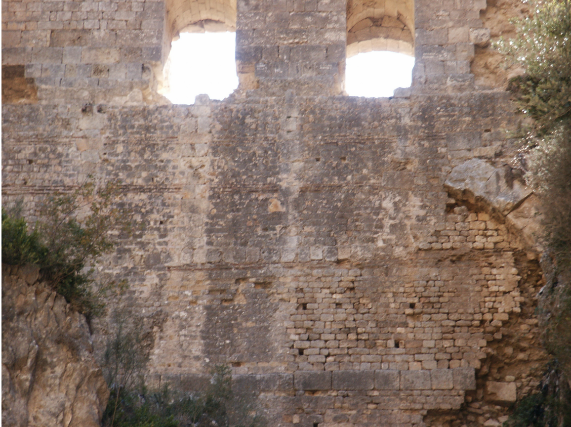
Fig. 4.8: Detail of the 'Iron Gates' dam, Antioch showing the brick courses [photo: author].
