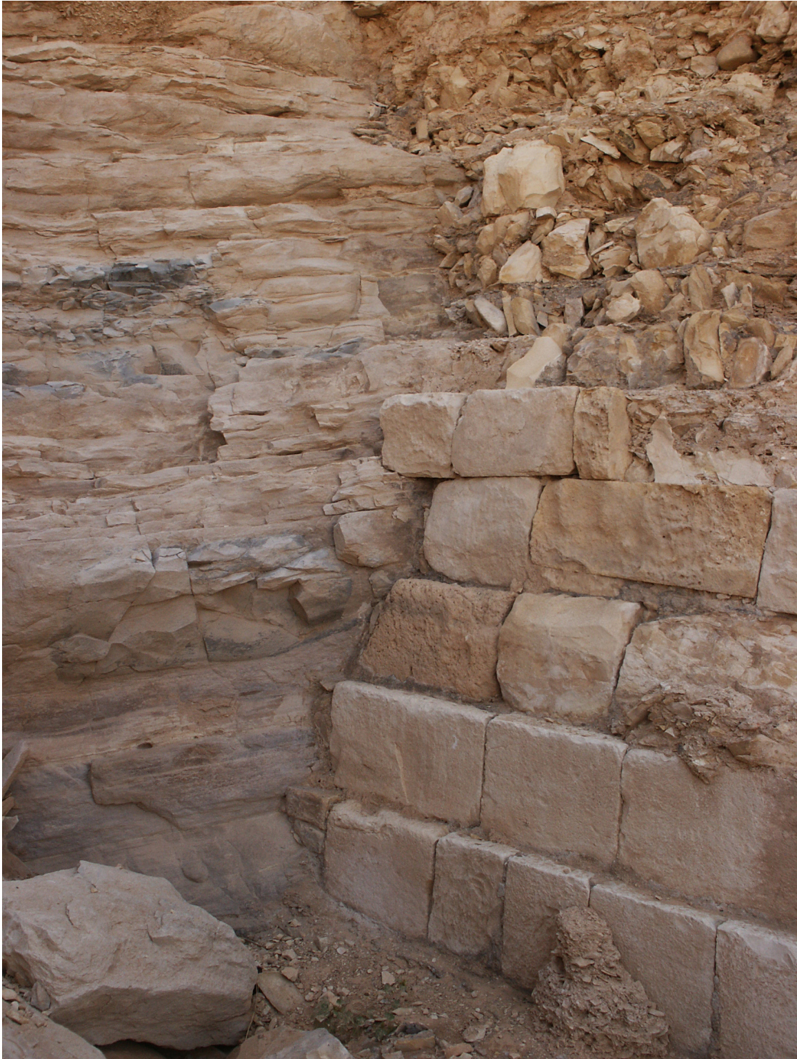
Fig. 4.10: Detail of the Harbaqa dam, Syria showing the stepped lower courses [photo: author].
