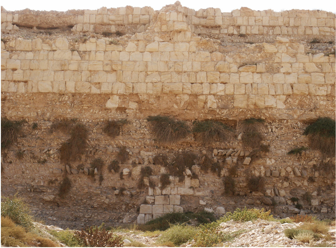
Fig. 4.15: Detail of the Harbaqa dam, Syria, showing the two building phases [photo: author].
