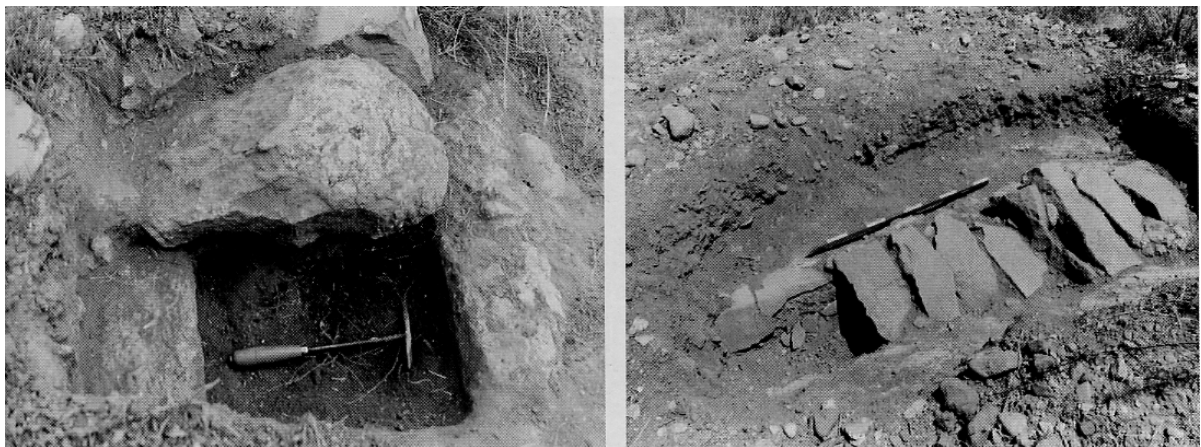
Fig. 6.5: Flat stone slabs covering the Hippos/Susita High Level aqueduct, Israel [Ben David 2002, figs 5 and 6].
