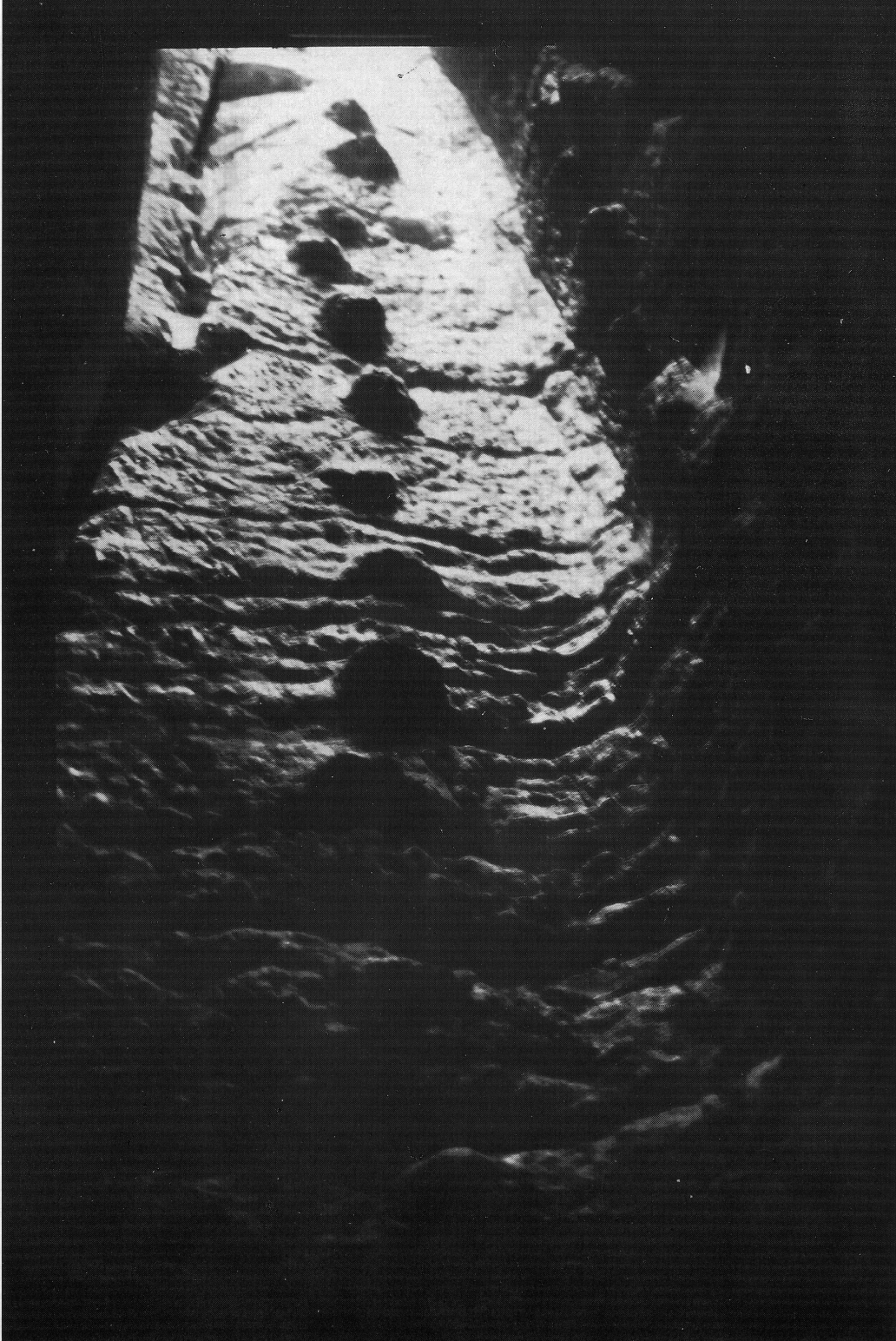
Fig. 6.12: Protrusions in a shaft of the Beirut tunnel, Lebanon [Davie et al. 1997, pl. 12].
