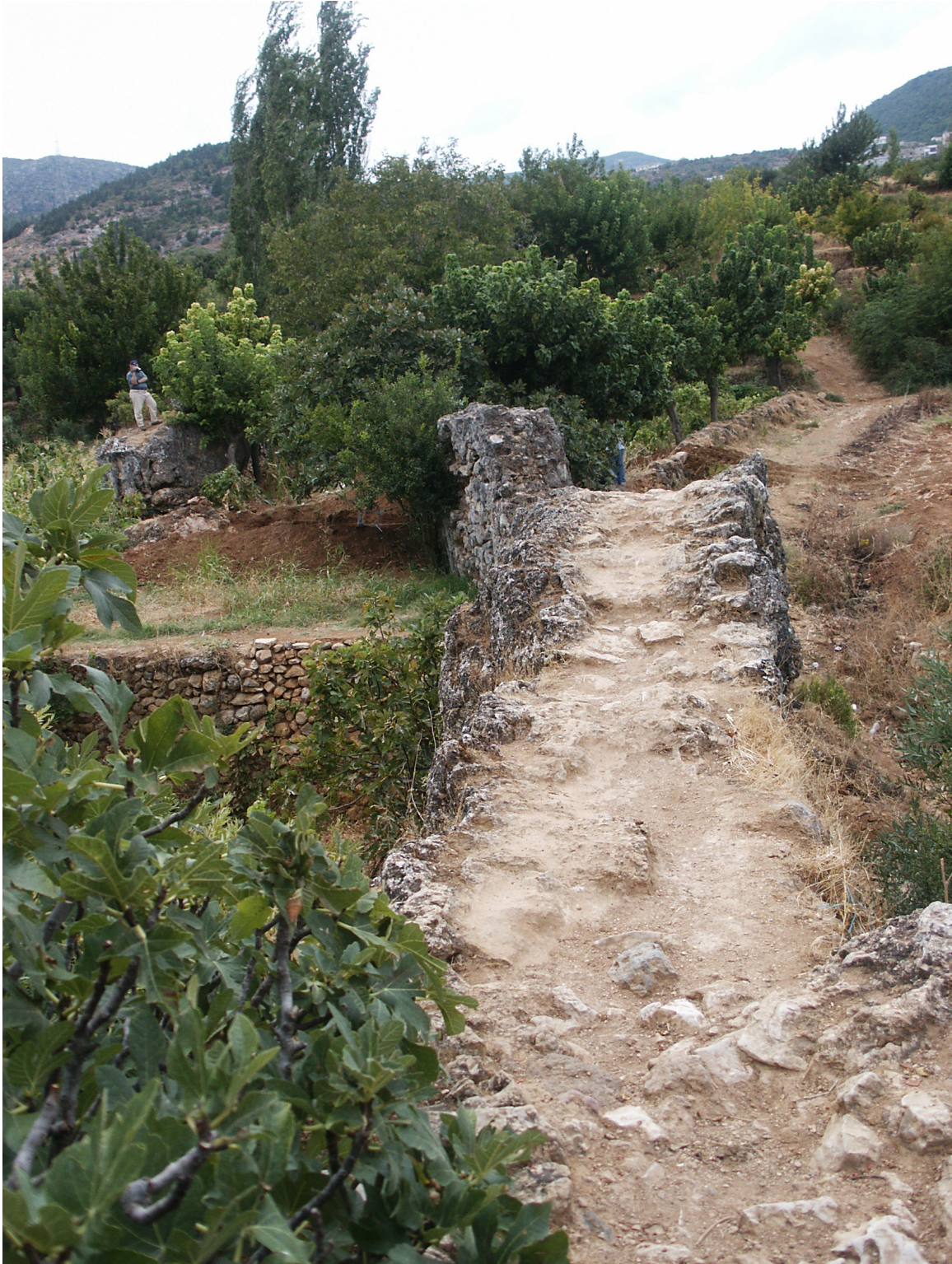
Fig. 6.29: Earthquake damage at the Misyaf aqueduct, Syria; the figure in the background is standing on the section of the aqueduct that has shifted [photo: author].
