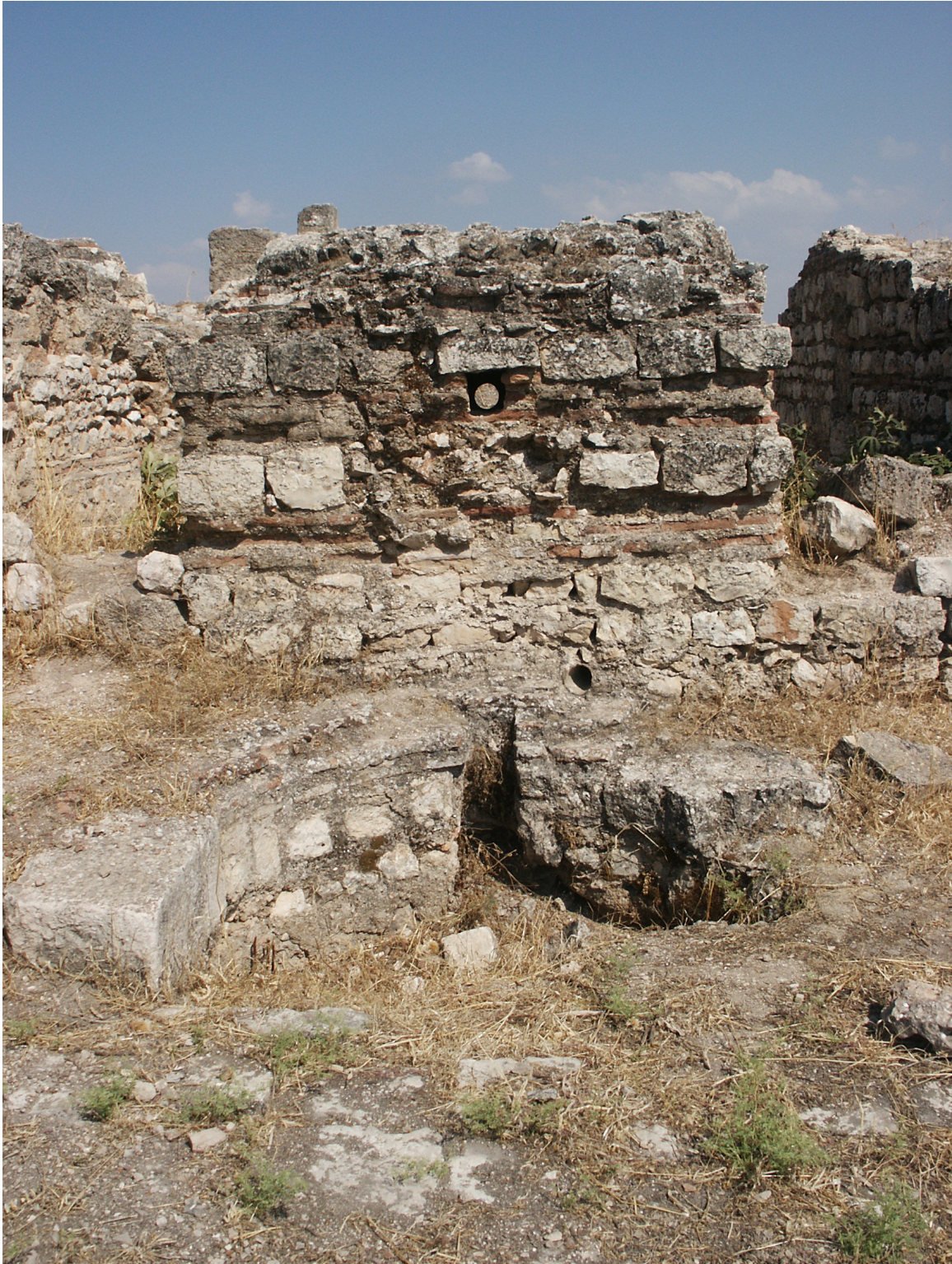
Fig. 9.14: Fountain with reservoir behind in the House of the Console Capitals [#376], Apamea [photo: author].
