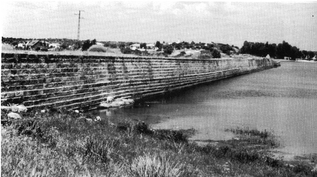
Fig. 4.9: Stepped dam at Proserpina, serving the city of Mérida, Spain [Hodge 1992, fig. 41].
