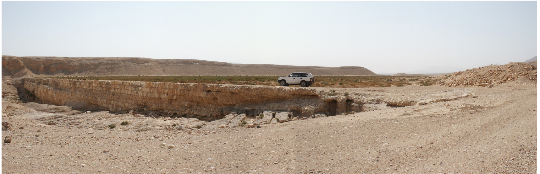
Fig. 4.6: Harbaqa dam, Syria, spanning a broad wadi [photo: author].
