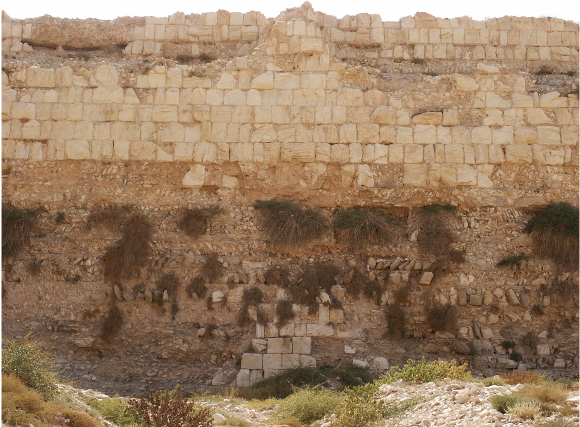
Fig. 4.15: Detail of the Harbaqa dam, Syria, showing the two building phases [photo: author].
